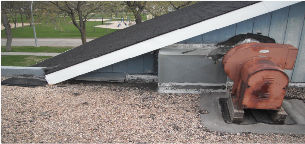
Fig.1: Coordinate 'boxing-in ' of overhang with Low-Slope Roofing.
