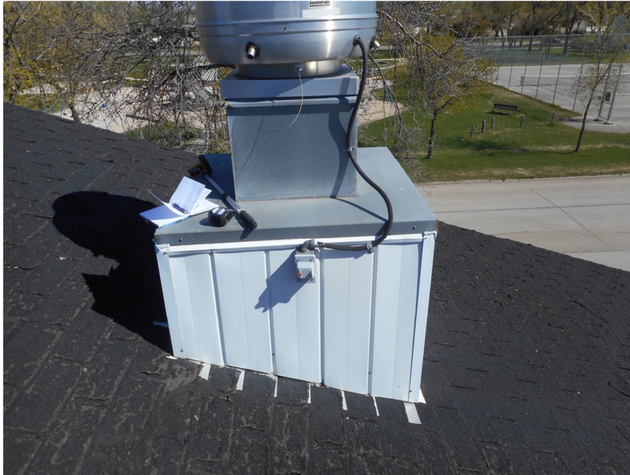
Fig. 3: Disengage curb flashing/sidings to envelope w/ waterproofing membrane. Supply & Install new flashings as required.
