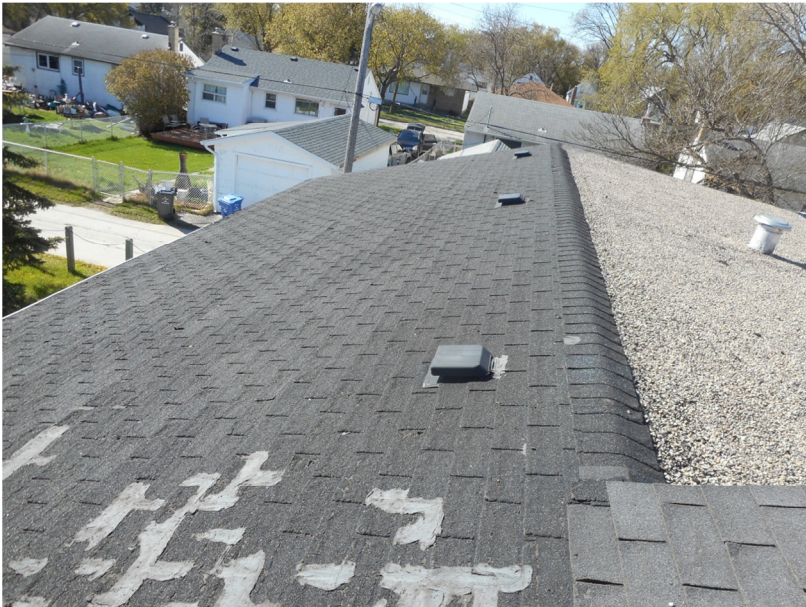
Fig. 2: Co-ordinate Steep-slope-to-BUR interface as required. Ensure attic venting is as per Code Requirements.
