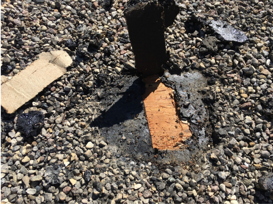
Fig. 3: Steep-slope BUR; 4-ply felt c/w gravel on plywood decking.
