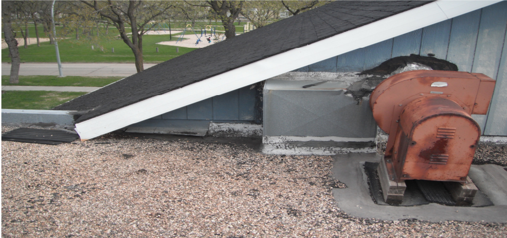
Fig.1: Coordinate 'boxing-in ' of overhang with Low-Slope Roofing.
