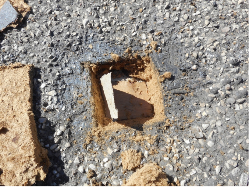
Fig. 2: Existing low-slope BUR core. 2" fibreboard & BUR.
