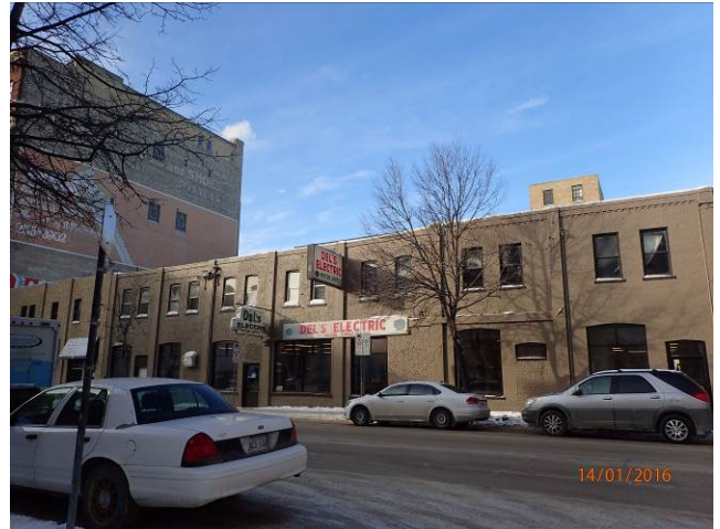
Photo 4. West view of west adjacent properties: commercial (54-68 Princess Street).
