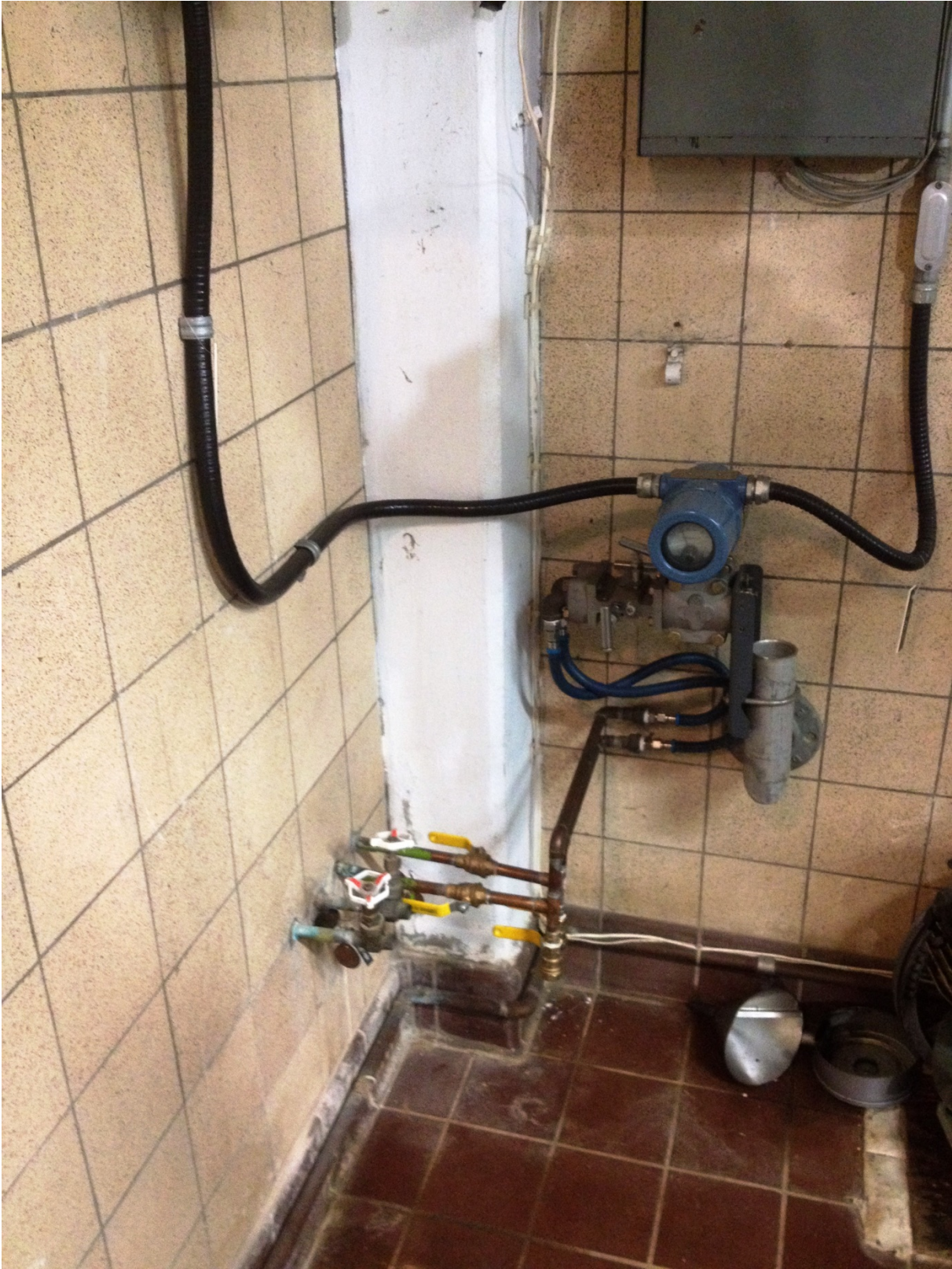
Photo 3: Hurst East Venturi Instrument Taps and Pressure Transmitter
