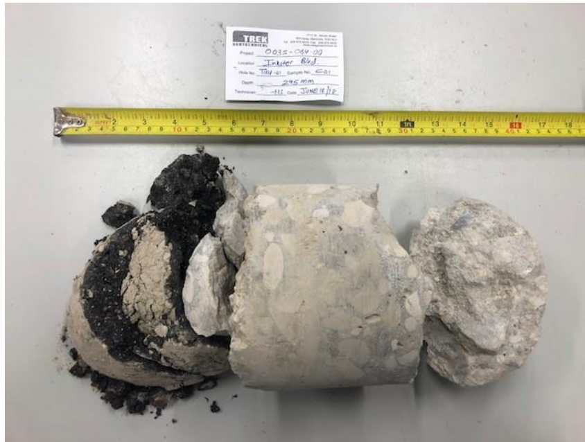
Photo 1: Pavement Core Sample at Test Hole TH18-01
