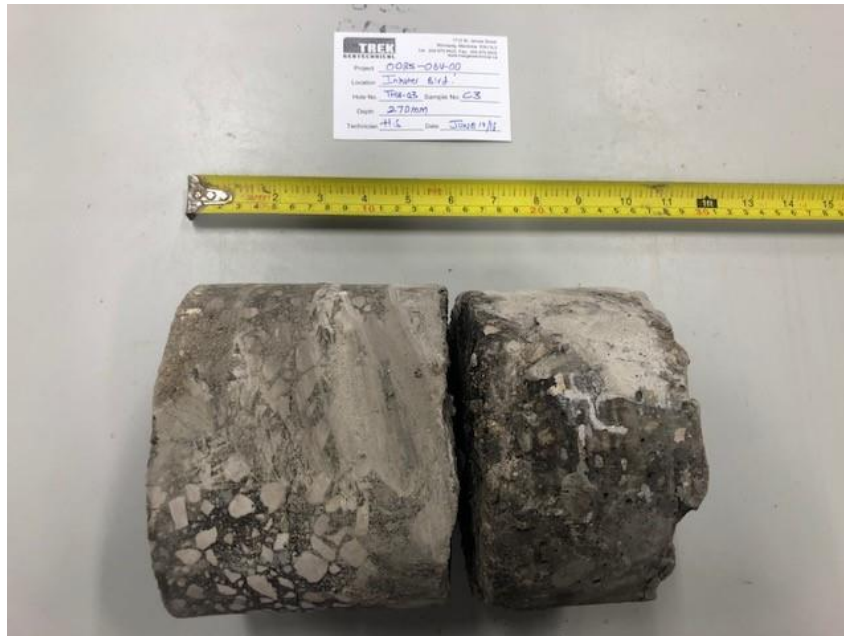
Photo 3: Pavement Core Sample at Test Hole TH18-03
