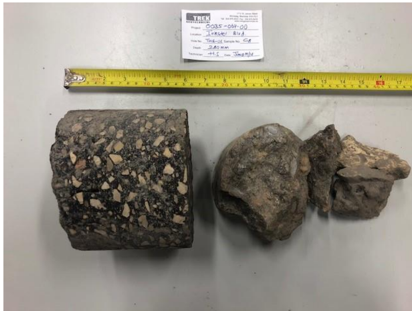
Photo 8: Pavement Core Sample at Test Hole TH18-08
