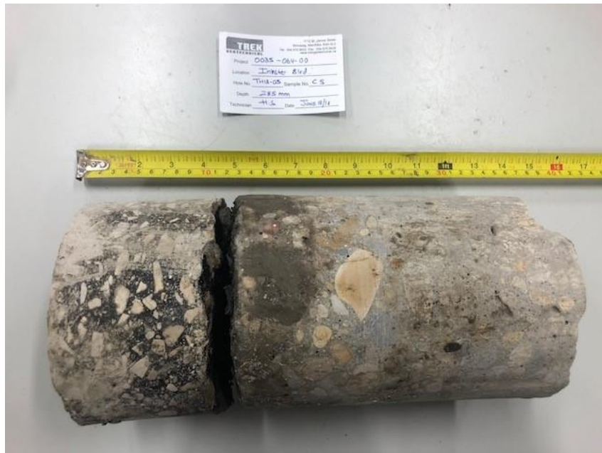
Photo 5: Pavement Core Sample at Test Hole TH18-05
