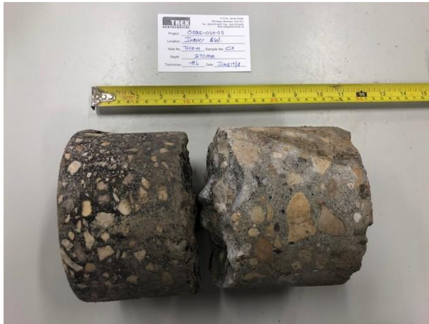
Photo 9: Pavement Core Sample at Test Hole TH18-09
