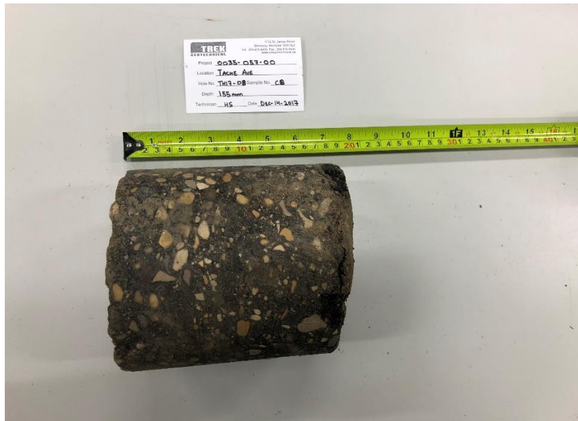
Photo 8: Pavement Core Sample at Test Hole TH17-08
