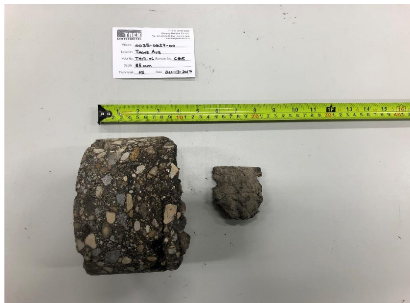
Photo 6: Pavement Core Sample at Test Hole TH17-06
