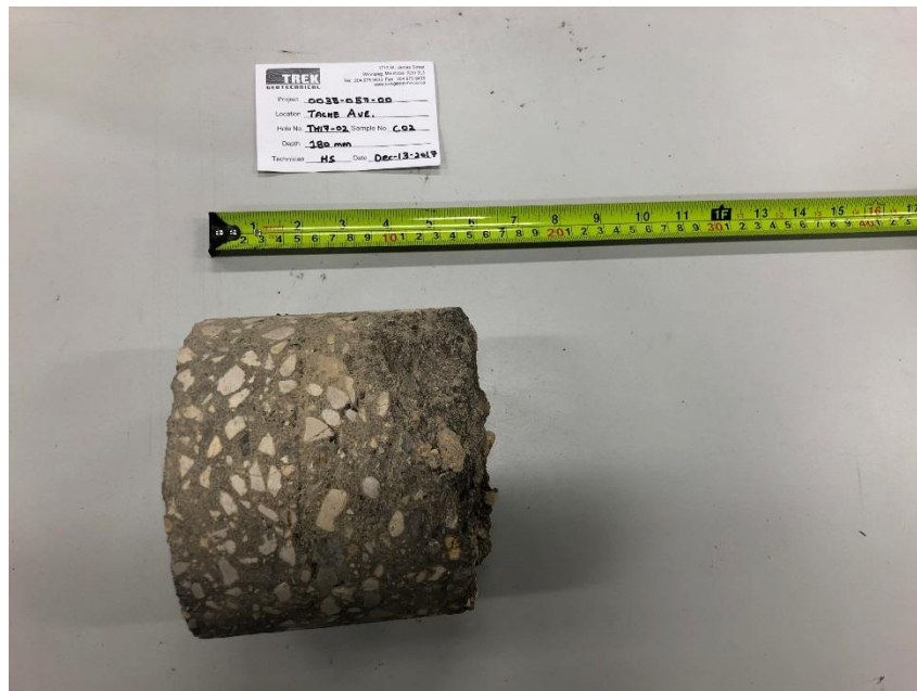
Photo 2: Pavement Core Sample at Test Hole TH17-02
