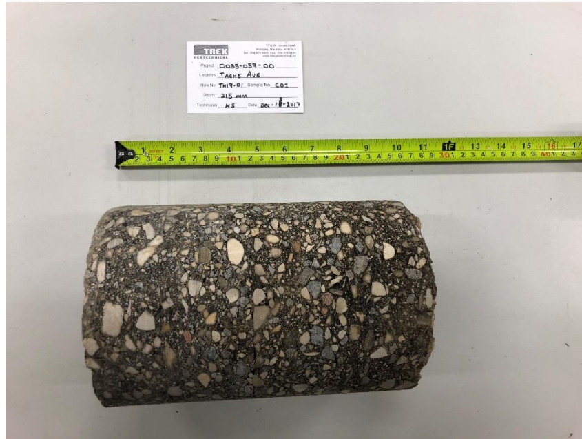
Photo 1: Pavement Core Sample at Test Hole TH17-01
