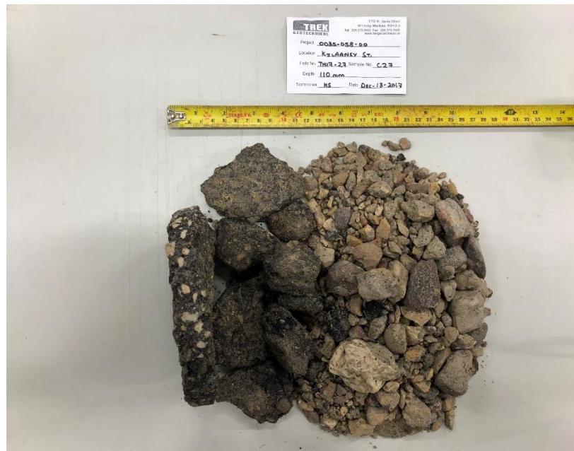
Photo 4: Pavement Core Sample at Test Hole TH17-27
