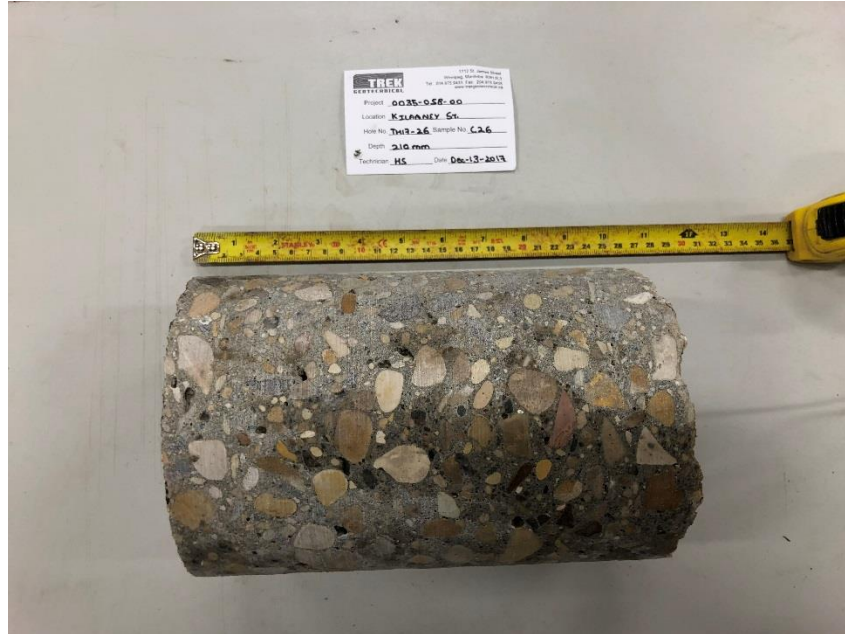
Photo 3: Pavement Core Sample at Test Hole TH17-26
