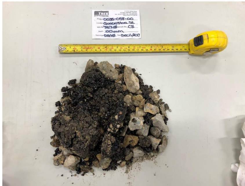
Photo 8: Pavement Core Sample at Test Hole TH17-08
