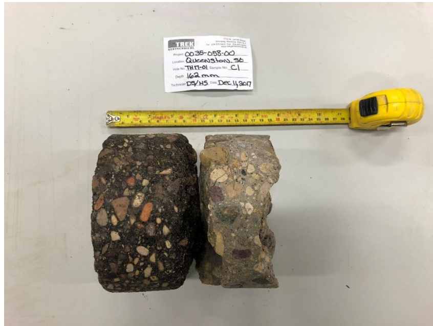
Photo 1: Pavement Core Sample at Test Hole TH17-01
