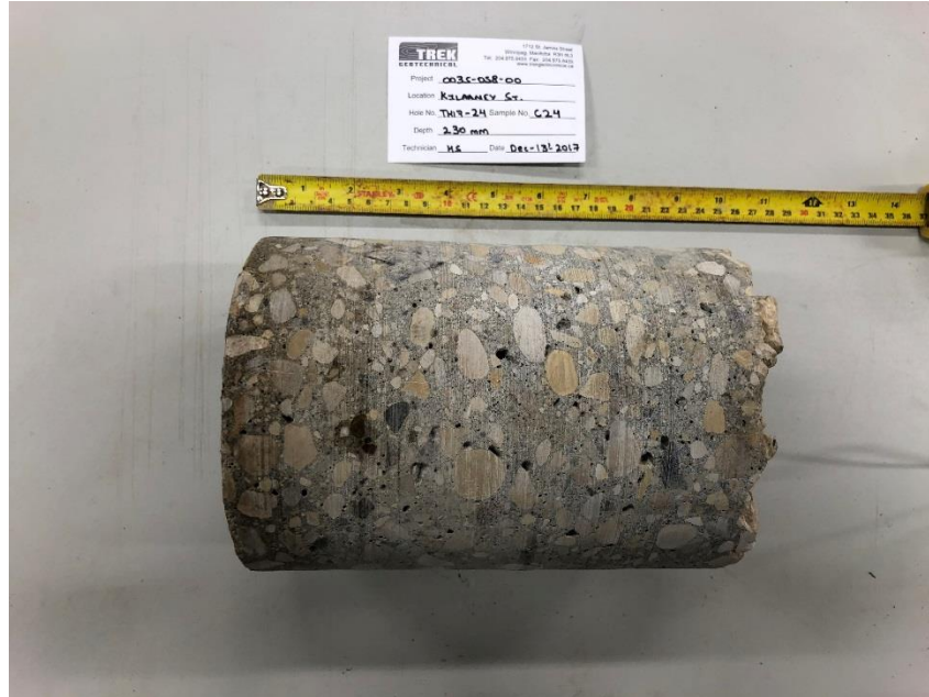
Photo 1: Pavement Core Sample at Test Hole TH17-24
