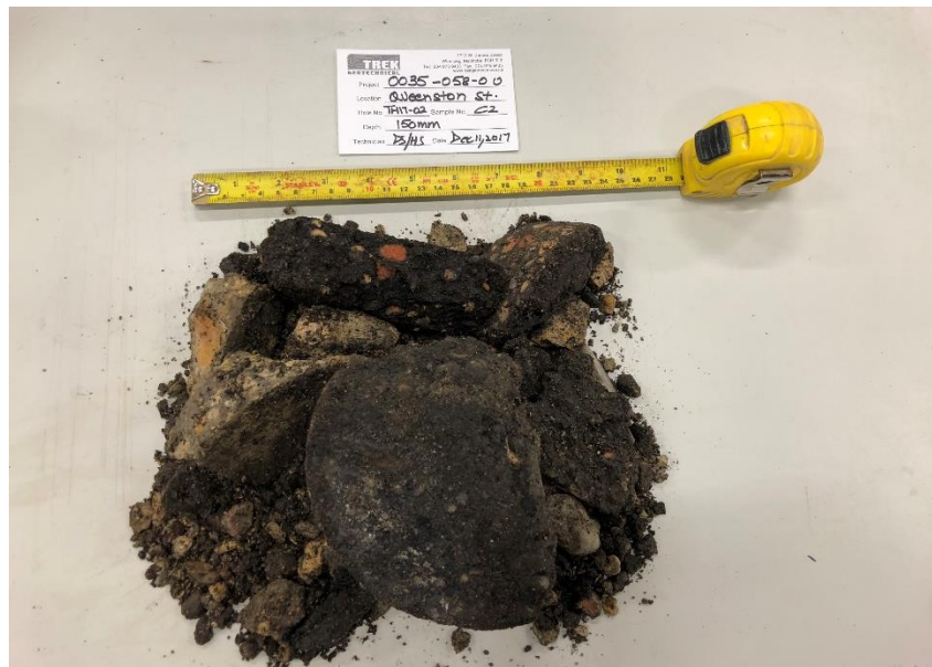
Photo 2: Pavement Core Sample at Test Hole TH17-02
