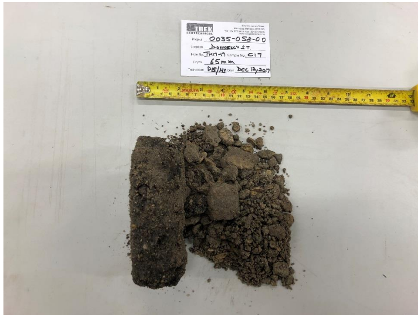
Photo 1: Pavement Core Sample at Test Hole TH17-17
