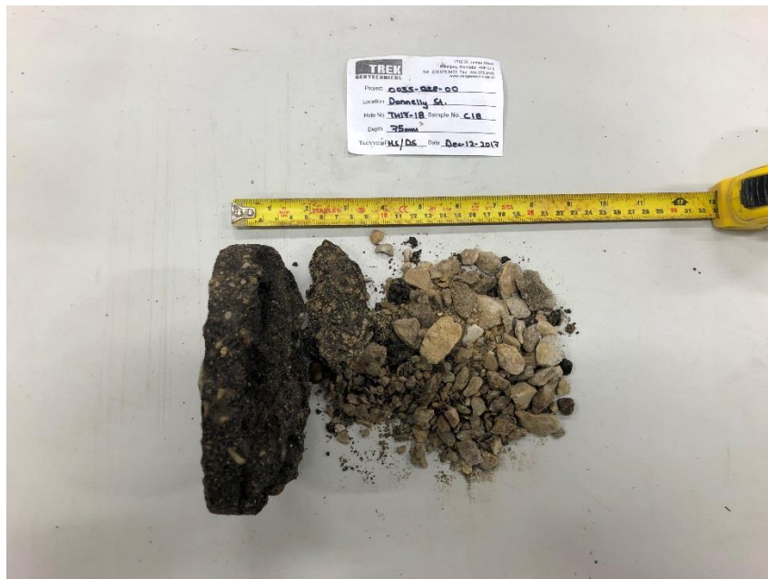
Photo 2: Pavement Core Sample at Test Hole TH17-18
