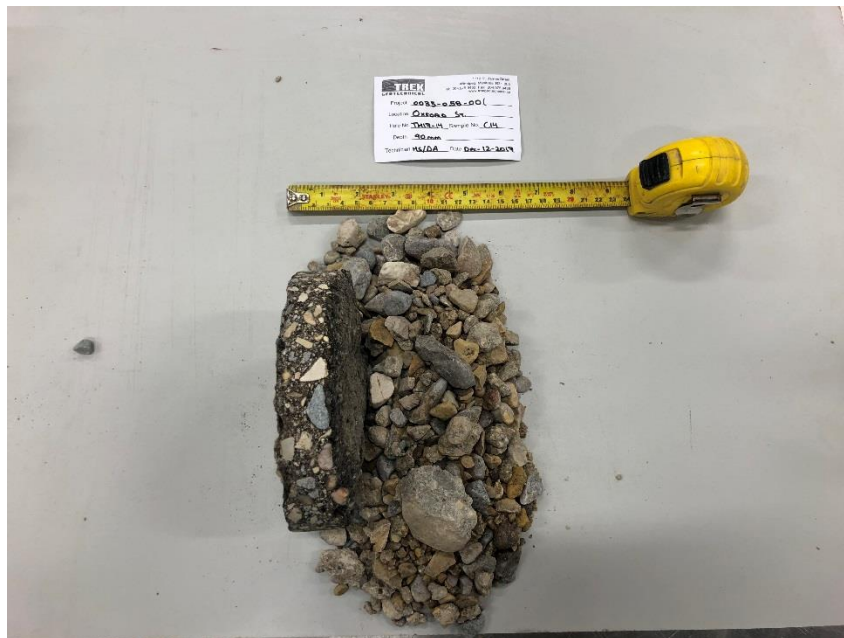
Photo 6: Pavement Core Sample at Test Hole TH17-14
