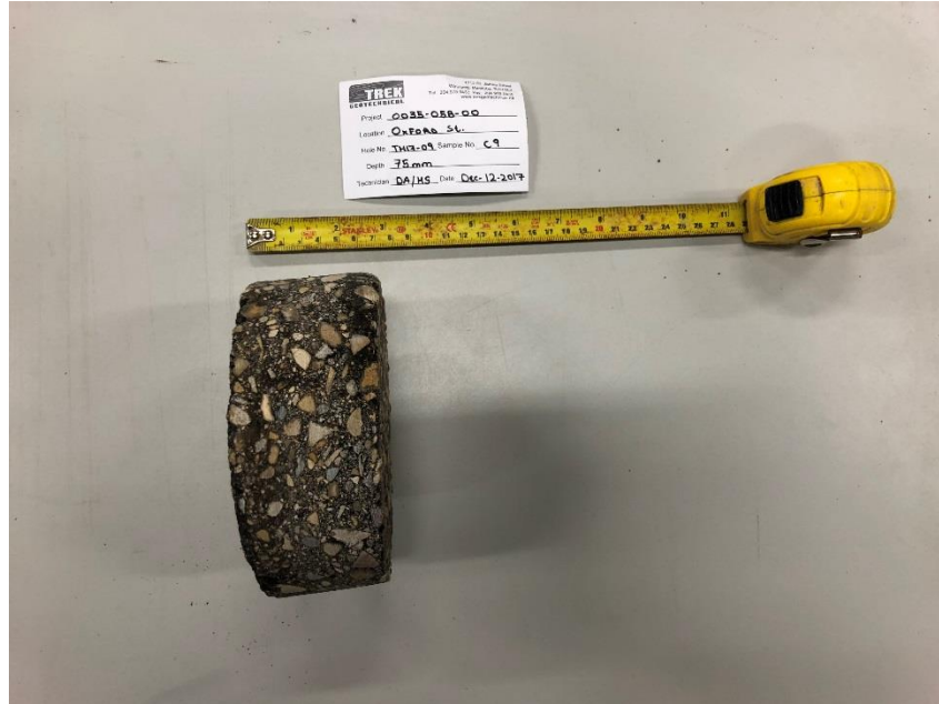
Photo 1: Pavement Core Sample at Test Hole TH17-09
