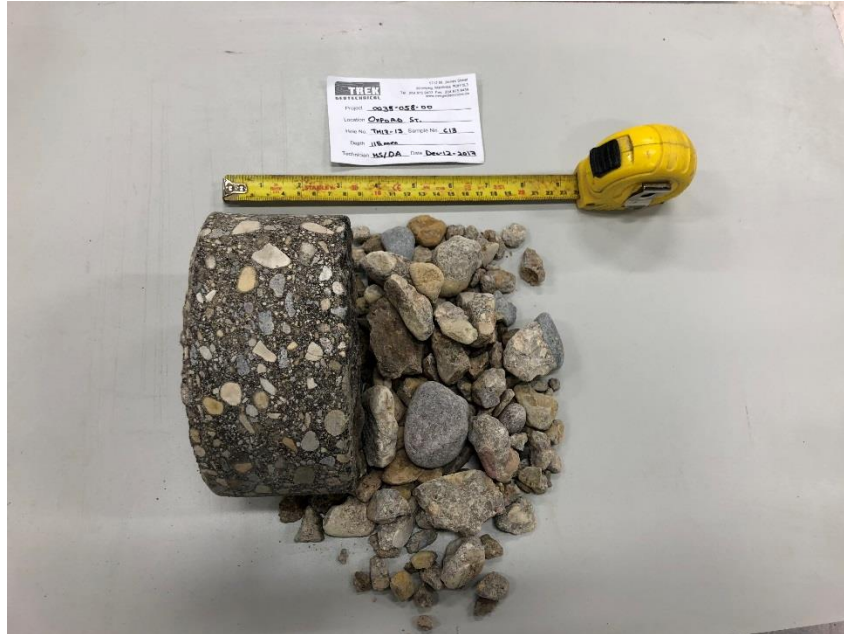
Photo 5: Pavement Core Sample at Test Hole TH17-13
