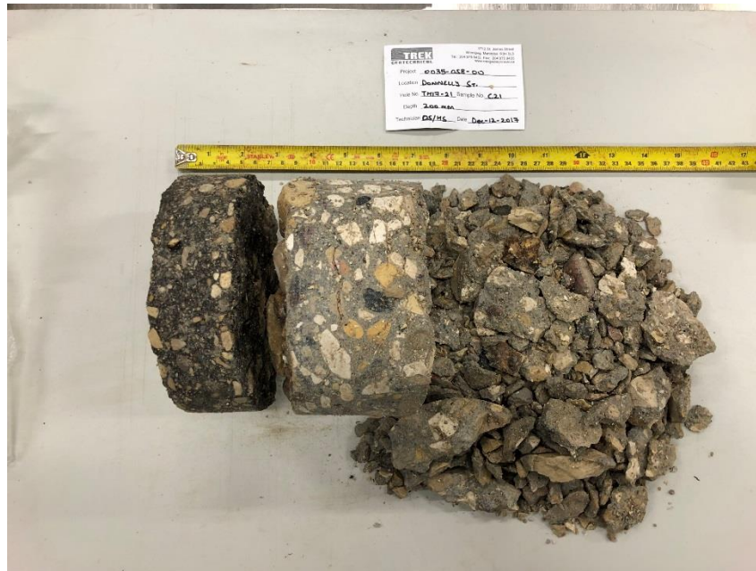
Photo 5: Pavement Core Sample at Test Hole TH17-21
