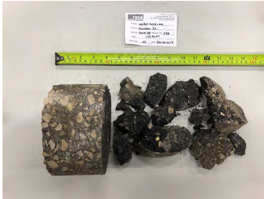
Photo 5: Pavement Core Sample at Test Hole TH17-38
