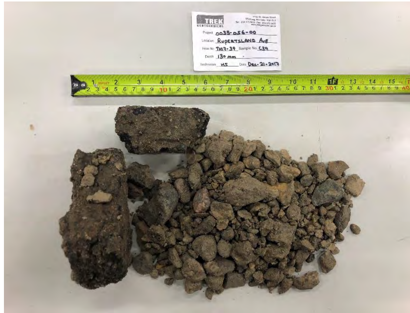
Photo 1: Pavement Core Sample at Test Hole TH17-39
