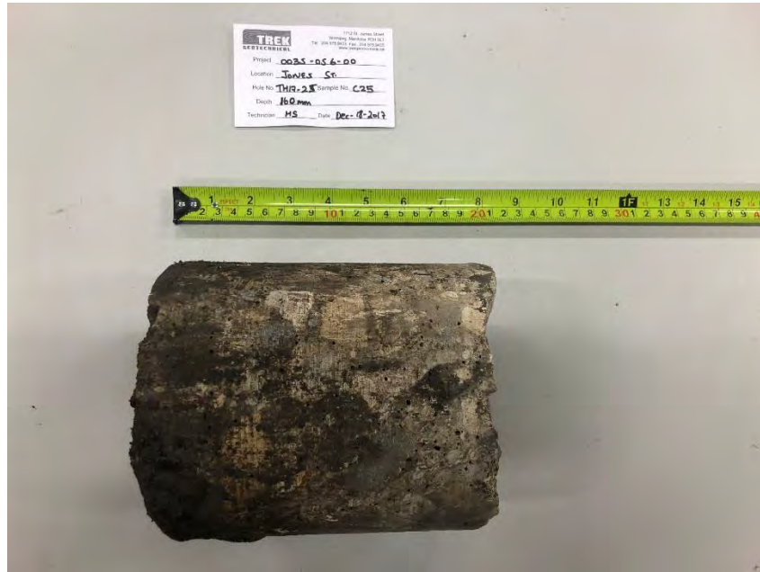
Photo 3: Pavement Core Sample at Test Hole TH17-25
