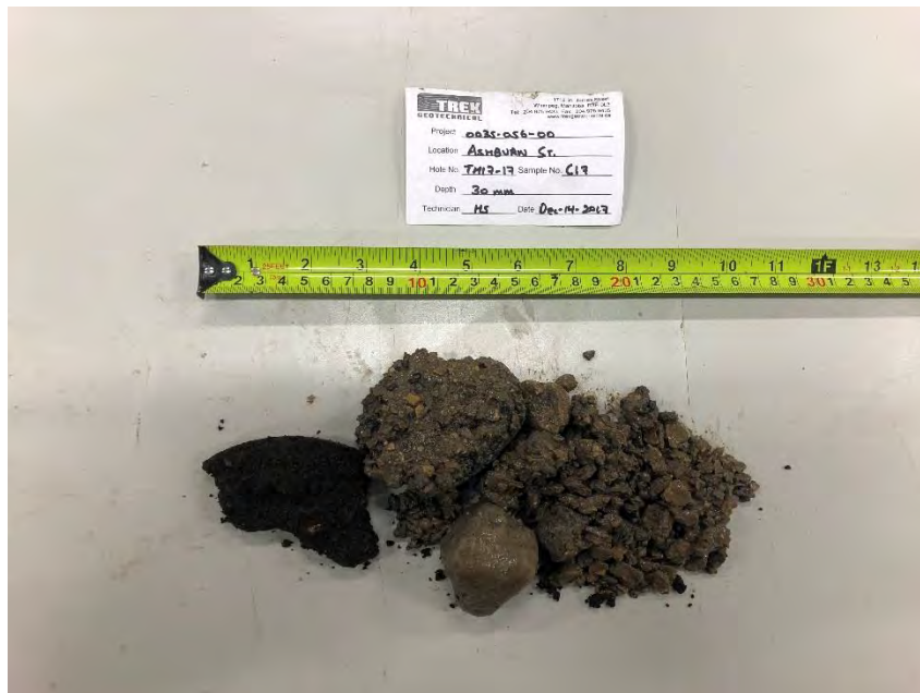
Photo 8: Pavement Core Sample at Test Hole TH17-17
