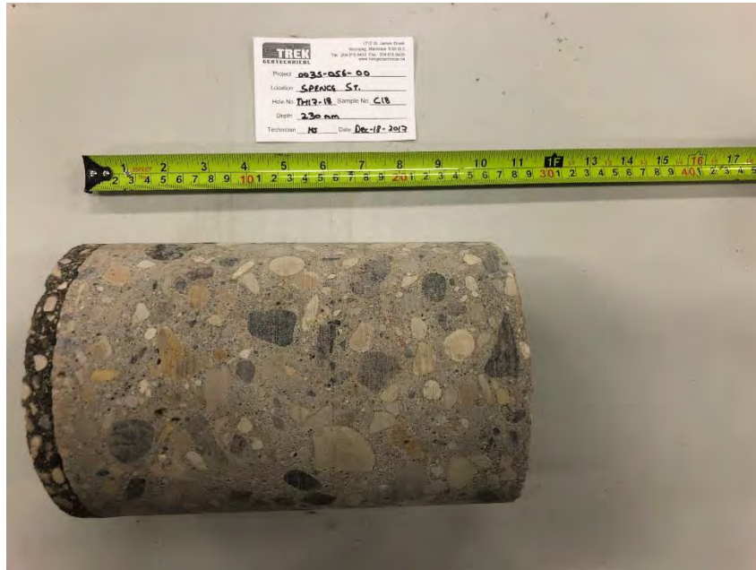
Photo 1: Pavement Core Sample at Test Hole TH17-18
