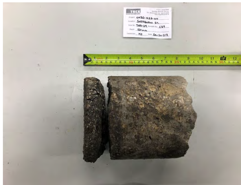
Photo 4: Pavement Core Sample at Test Hole TH17-29
