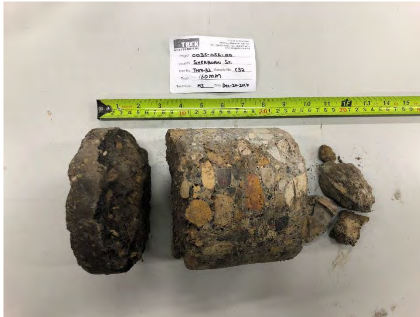
Photo 7: Pavement Core Sample at Test Hole TH17-32
