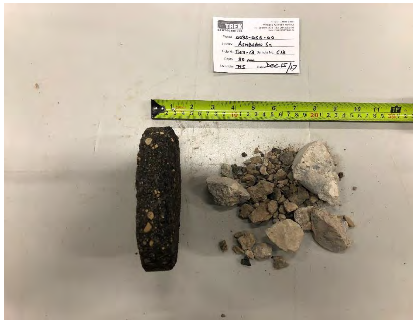
Photo 4: Pavement Core Sample at Test Hole TH17-13
