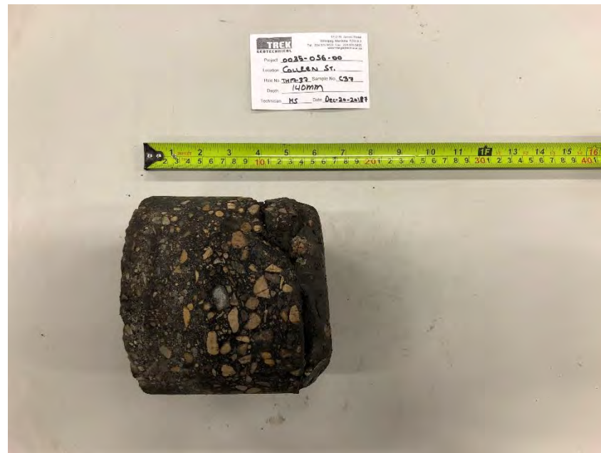
Photo 4: Pavement Core Sample at Test Hole TH17-37
