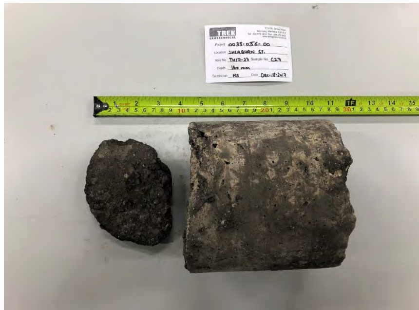
Photo 2: Pavement Core Sample at Test Hole TH17-27
