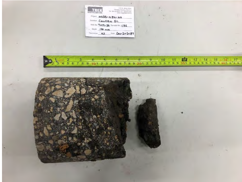
Photo 3: Pavement Core Sample at Test Hole TH17-36
