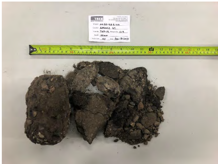
Photo 2: Pavement Core Sample at Test Hole TH17-19
