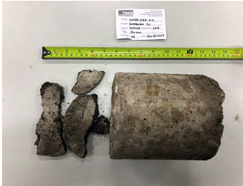
Photo 3: Pavement Core Sample at Test Hole TH17-28
