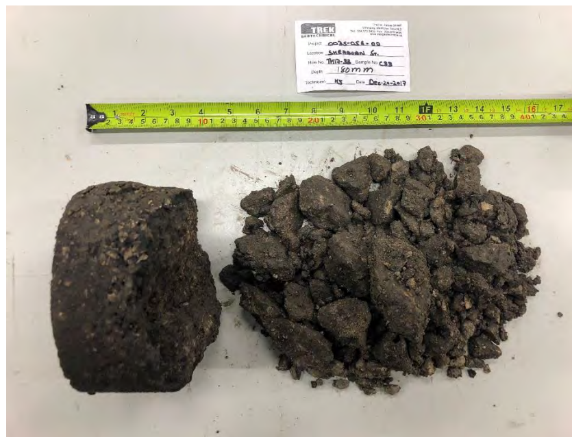
Photo 8: Pavement Core Sample at Test Hole TH17-33
