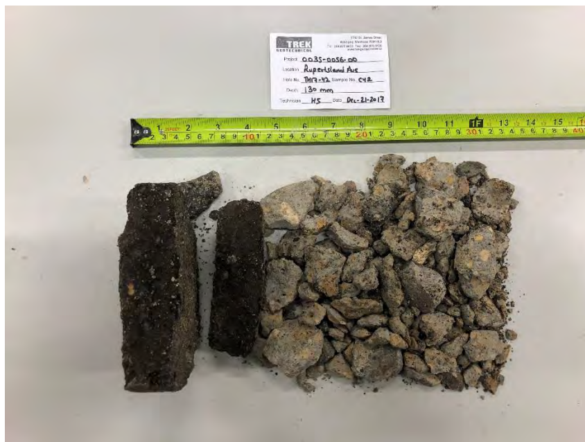
Photo 4: Pavement Core Sample at Test Hole TH17-42
