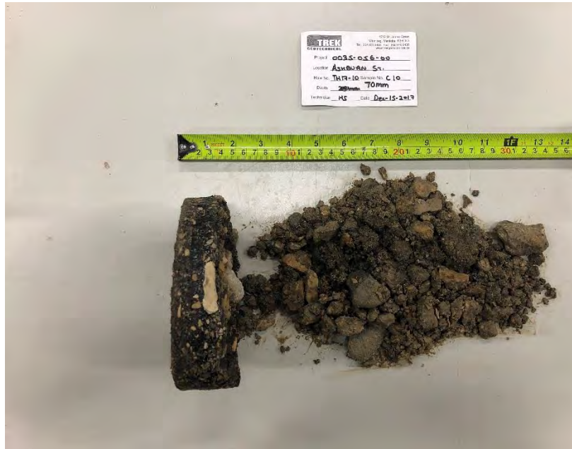
Photo 1: Pavement Core Sample at Test Hole TH17-10
