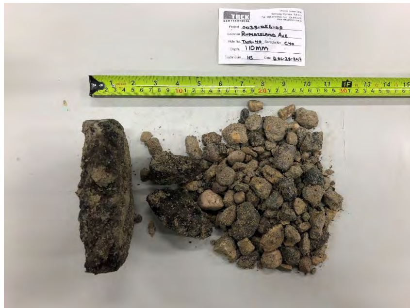
Photo 2: Pavement Core Sample at Test Hole TH17-40
