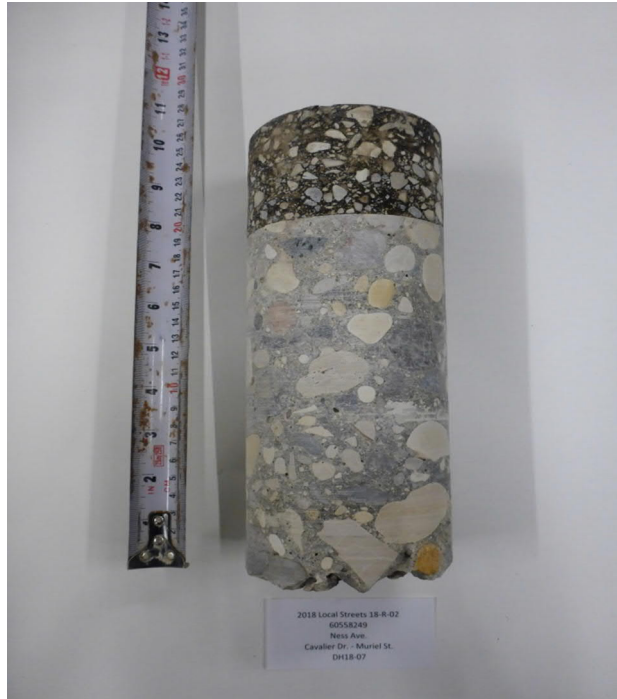
Photograph 16: Pavement Core PC18-17 – Ness Ave
