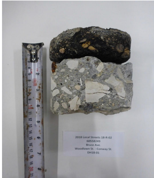
Photograph 10: Pavement Core PC18-11 – Bruce Ave
