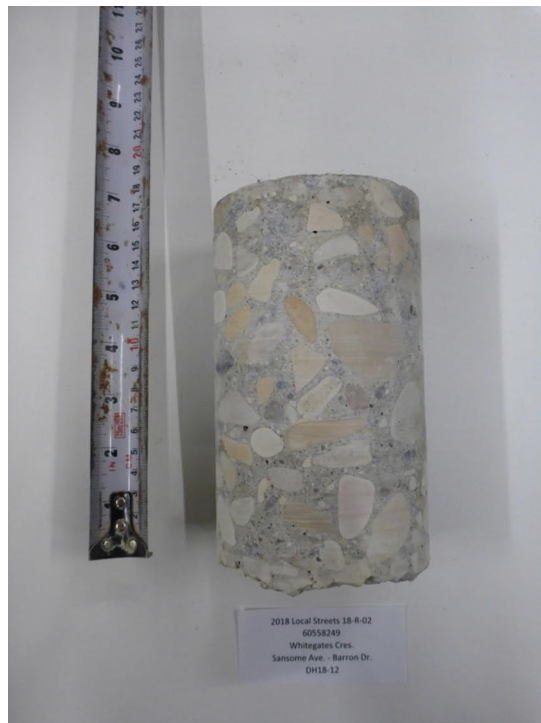
Photograph 21: Pavement Core PC18-22 – Whitegates Cresc
