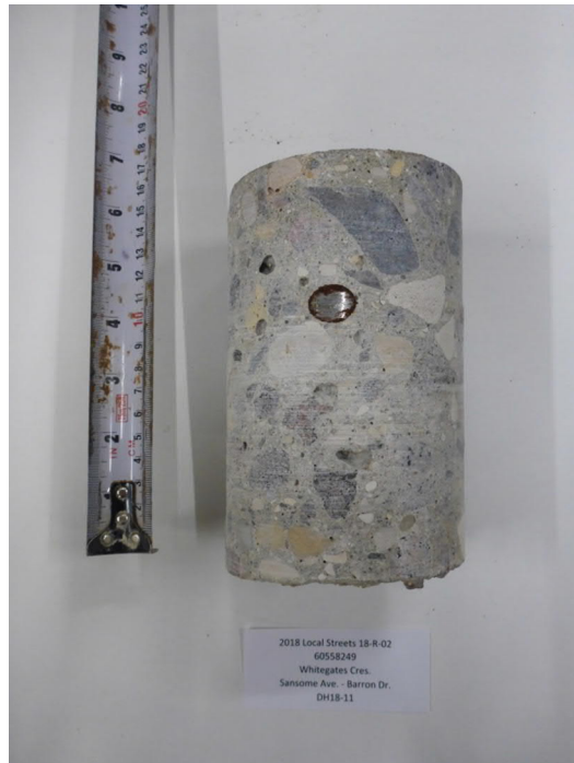
Photograph 20: Pavement Core PC18-21 – Whitegates Cresc
