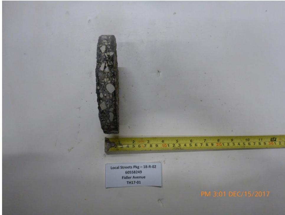
Photograph 1: Test Hole TH17-01 – Fidler Ave
