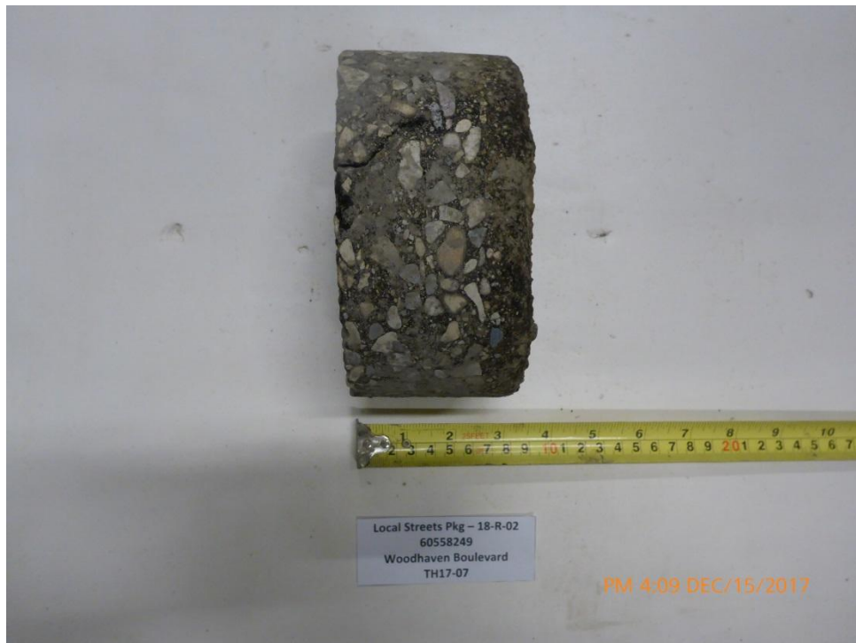
Photograph 6: Test Hole TH17-07 – Woodhaven Blvd
