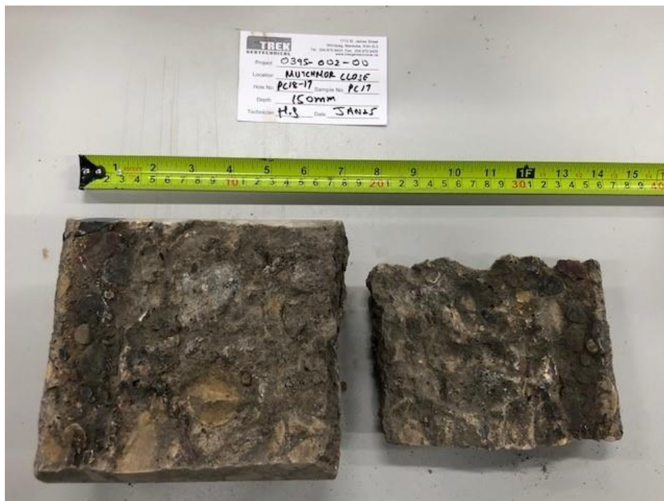
Photo 4: Pavement Core Sample at Test Hole PC18-17
