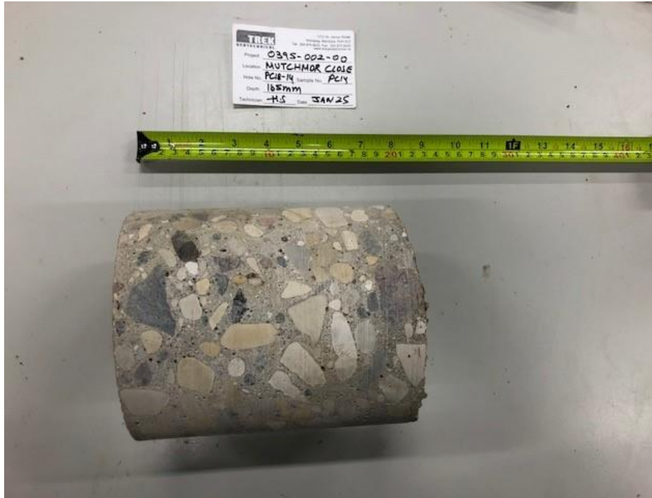
Photo 1: Pavement Core Sample at Test Hole PC18-14
