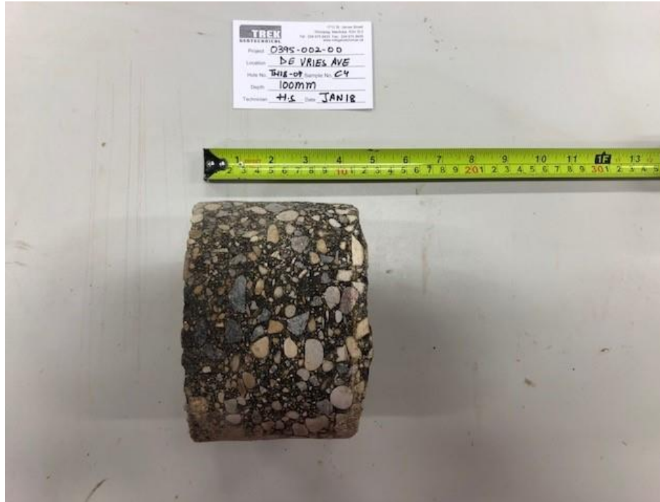
Photo 1: Pavement Core Sample at Test Hole TH18-04
