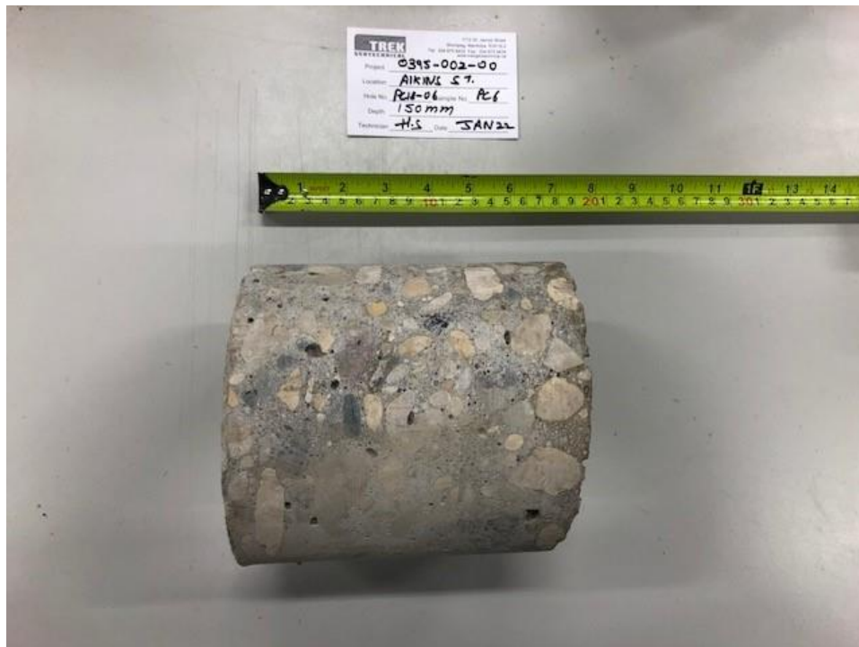
Photo 6: Pavement Core Sample at Test Hole PC18-06
