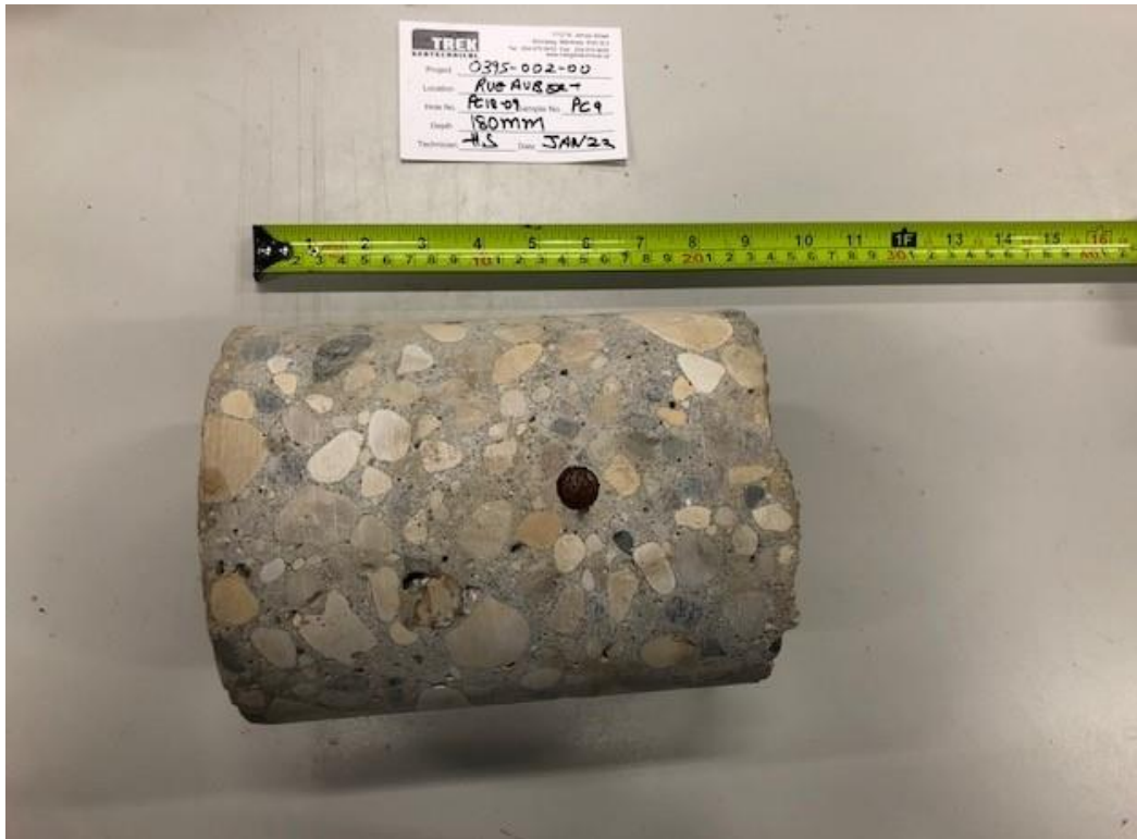
Photo 3: Pavement Core Sample at Test Hole PC18-09
