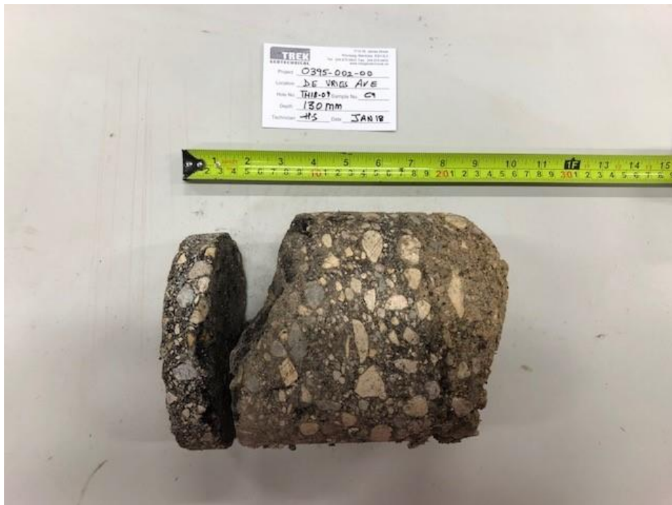
Photo 6: Pavement Core Sample at Test Hole TH18-09
