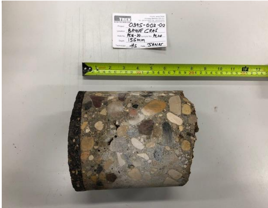
Photo 1: Pavement Core Sample at Test Hole PC18-20
