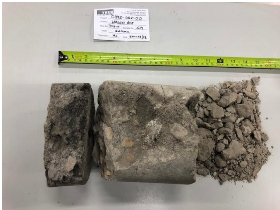
Photo 2: Pavement Core Sample at Test Hole TH18-14
