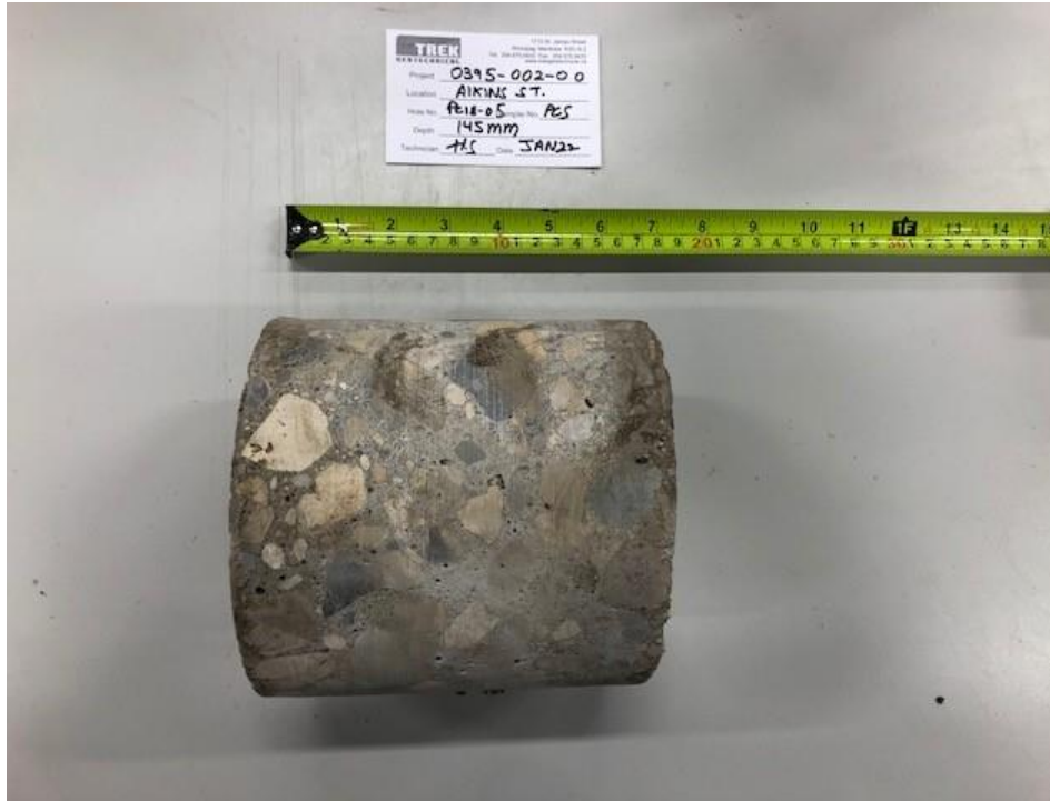
Photo 5: Pavement Core Sample at Test Hole PC18-05
