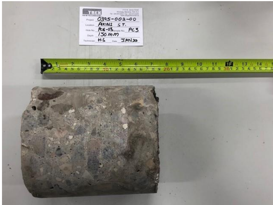
Photo 3: Pavement Core Sample at Test Hole PC18-03
