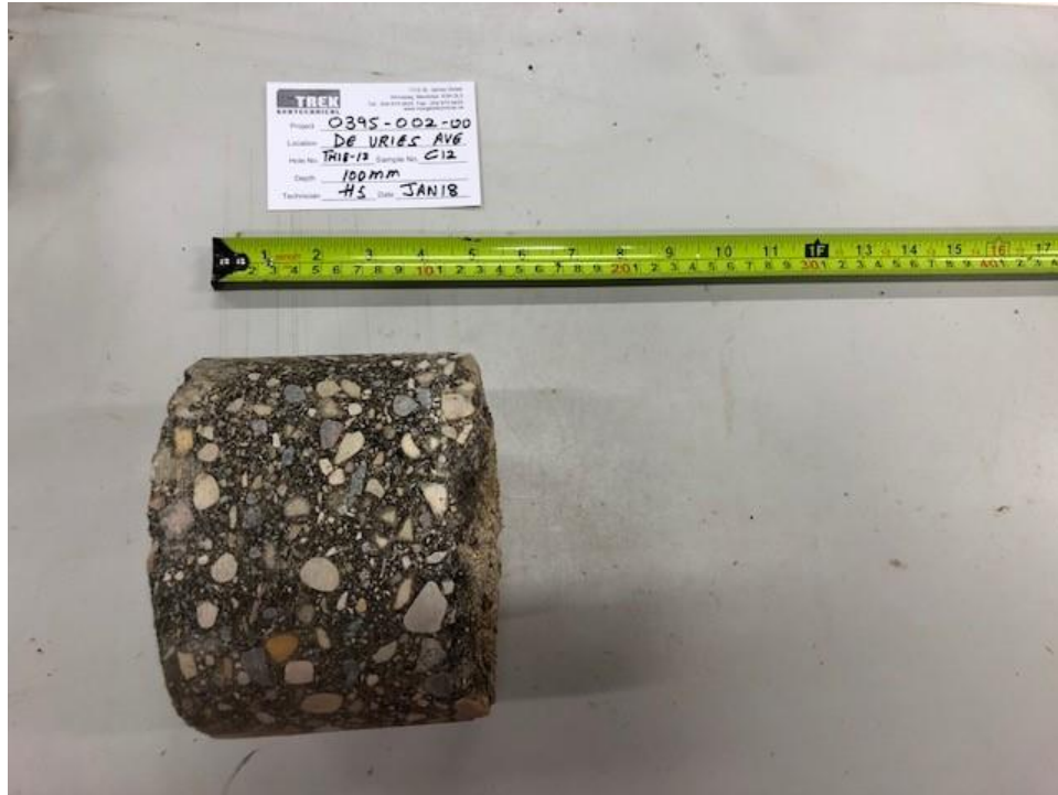
Photo 9: Pavement Core Sample at Test Hole TH18-12
