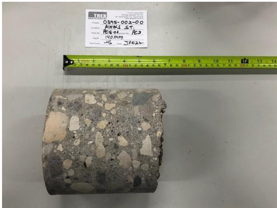
Photo 2: Pavement Core Sample at Test Hole PC18-02
