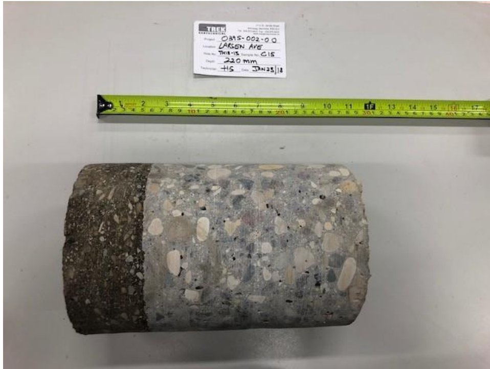
Photo 3: Pavement Core Sample at Test Hole TH18-15
