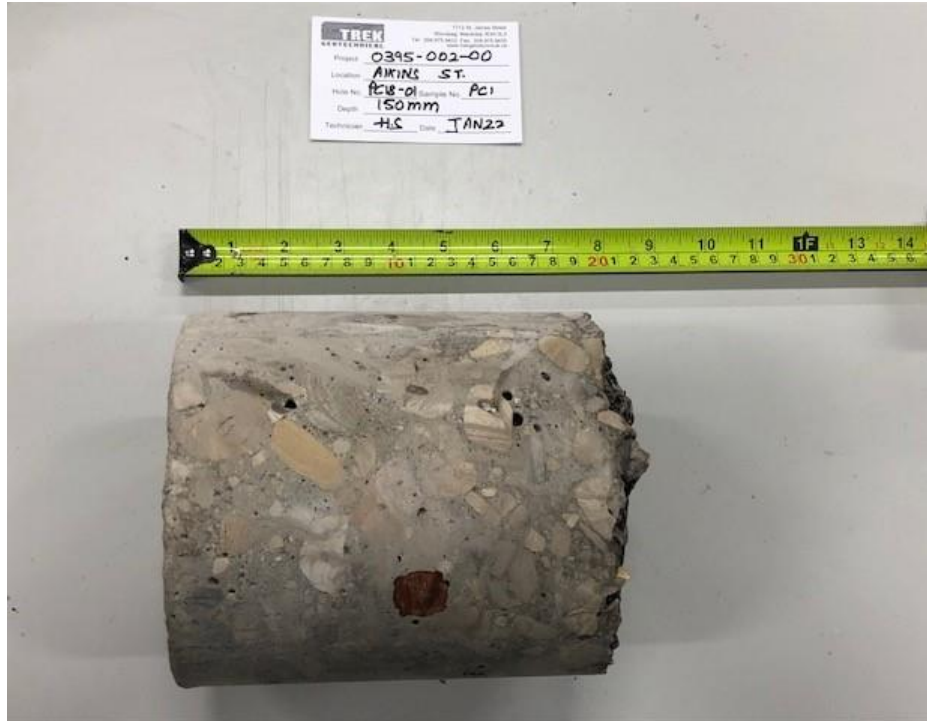
Photo 1: Pavement Core Sample at Test Hole PC18-01
