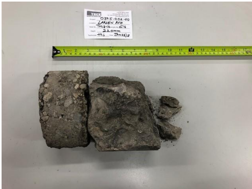
Photo 4: Pavement Core Sample at Test Hole TH18-16
