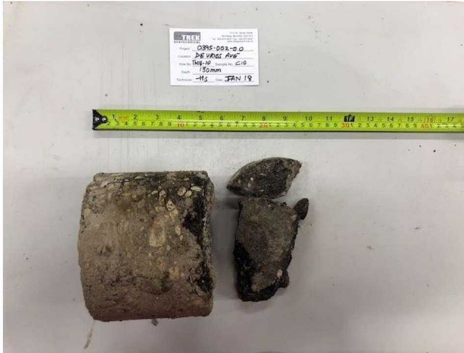
Photo 7: Pavement Core Sample at Test Hole TH18-10
