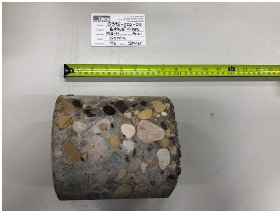
Photo 2: Pavement Core Sample at Test Hole PC18-21
