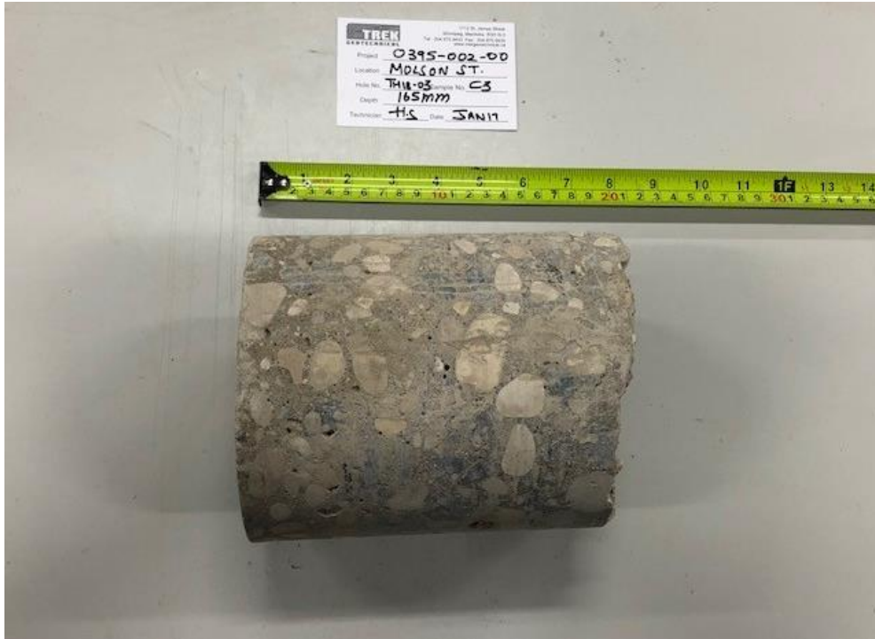
Photo 3: Pavement Core Sample at Test Hole TH18-03
