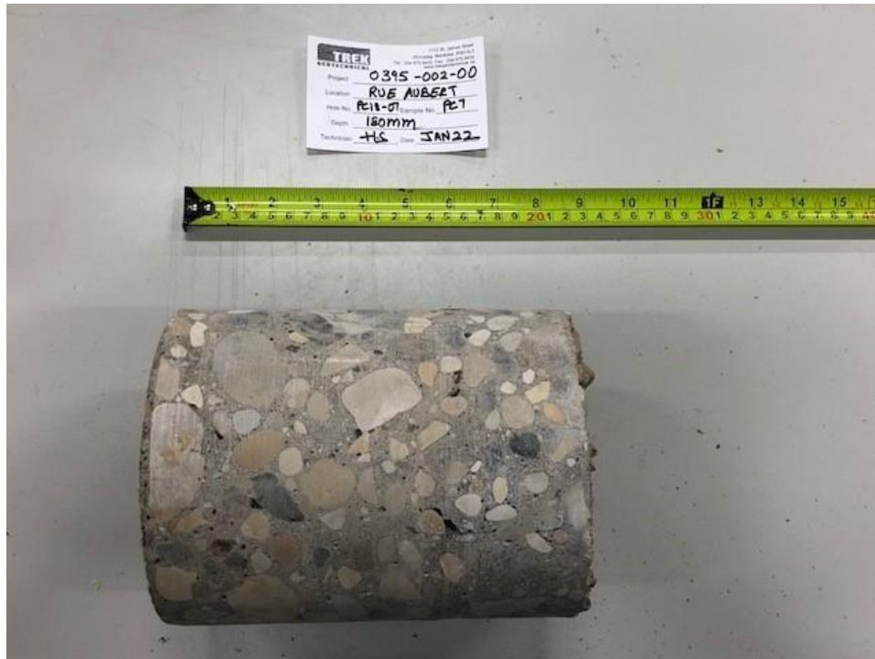
Photo 1: Pavement Core Sample at Test Hole PC18-07
