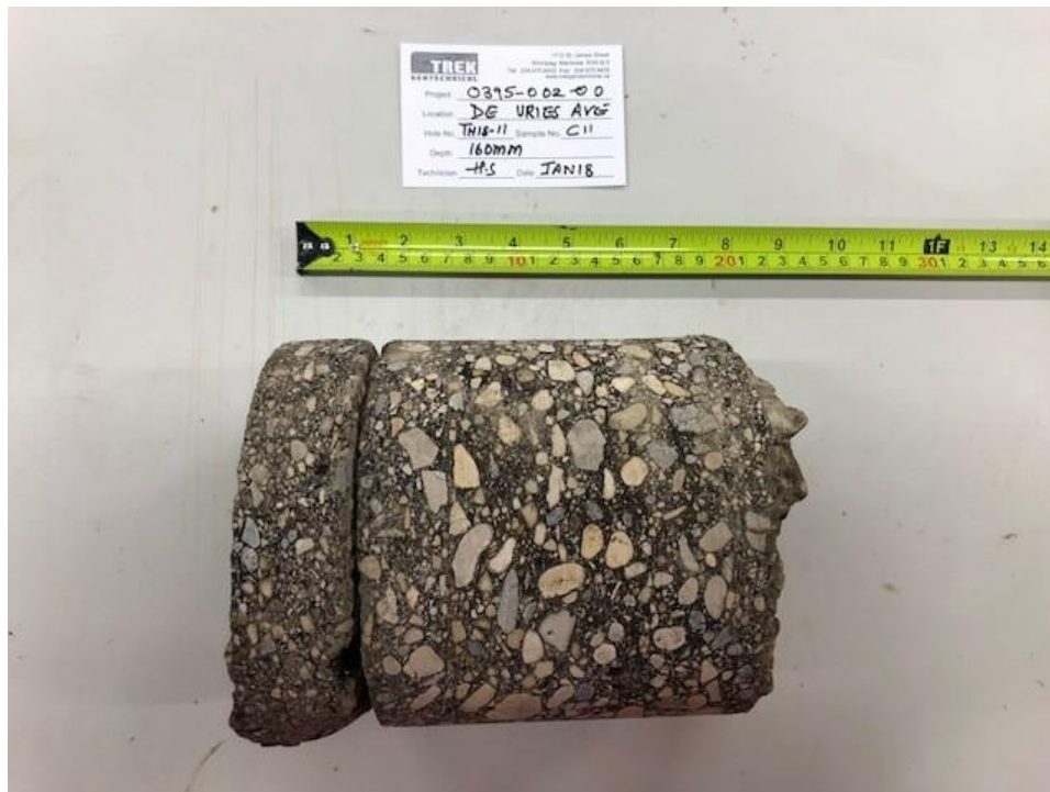
Photo 2: Pavement Core Sample at Test Hole PC18-11
