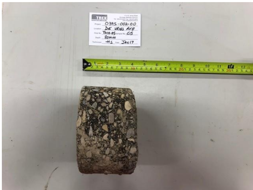
Photo 2: Pavement Core Sample at Test Hole TH18-05
