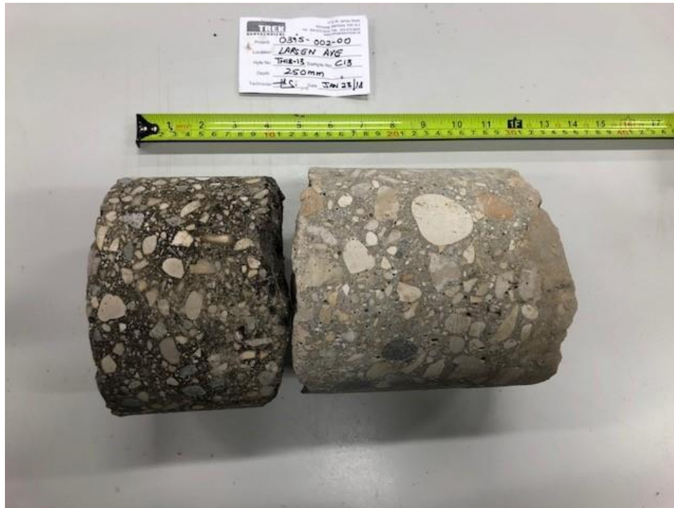
Photo 1: Pavement Core Sample at Test Hole TH18-13
