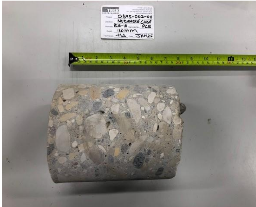
Photo 5: Pavement Core Sample at Test Hole PC18-18
