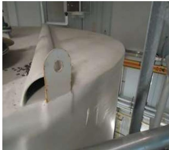
Photo Set 6: Appurtenances – Lid Rib and Lifting Lugs
