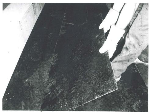
Step 2: Installation on the parapet.
