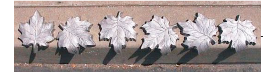
28 Maple Leaf Anti-Skateboarding Guards Cast Aluminum, 127mm Ø, for 25mm radius Concrete Edge. Install equally spaced around edge of Round Plinth as per manufacturer's instructions.
