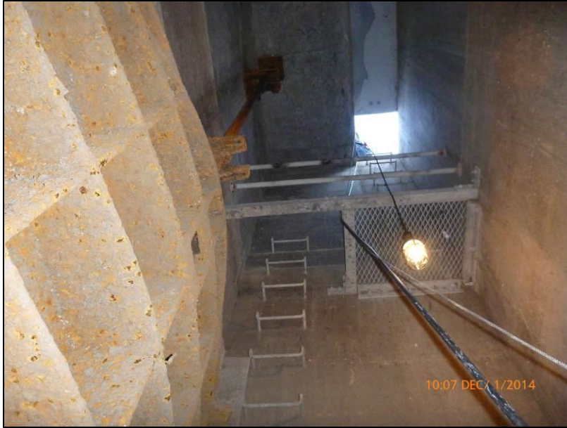
Photograph No. 7 Ladder and intermediate landing
