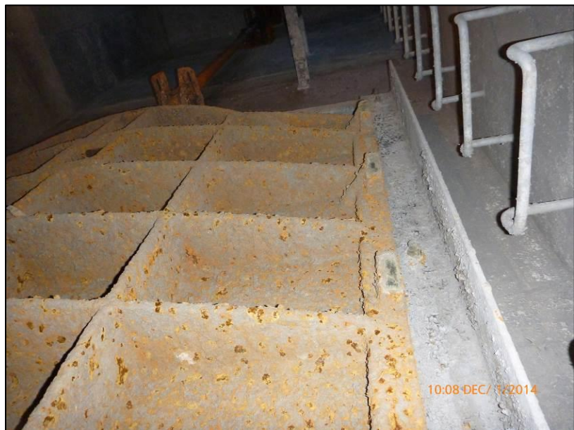
Photograph No. 8 Existing sluice and gate guide
