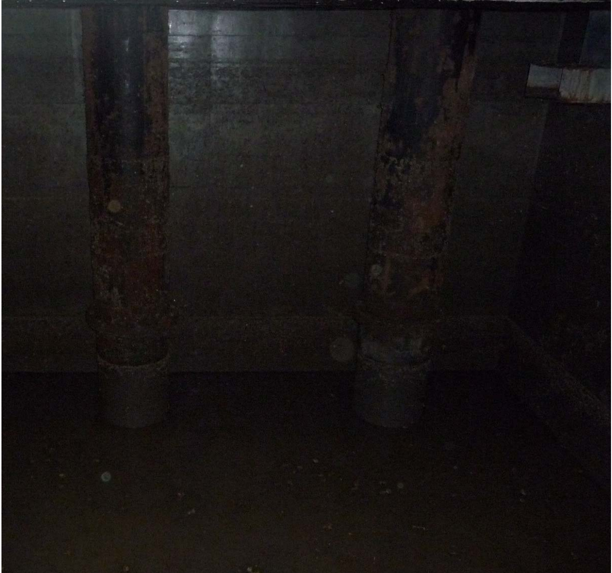
Figure 13: Metro Route 90 Underpass Pumping Station – Pump 1 and 2 Lower Columns
