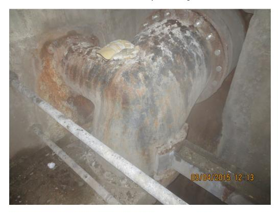
Site 1 – West chamber interior - existing side-outlet elbow with welded brace
