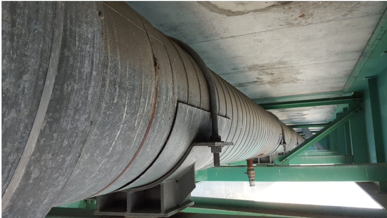
Site 3 – Force main at underside of bridge
