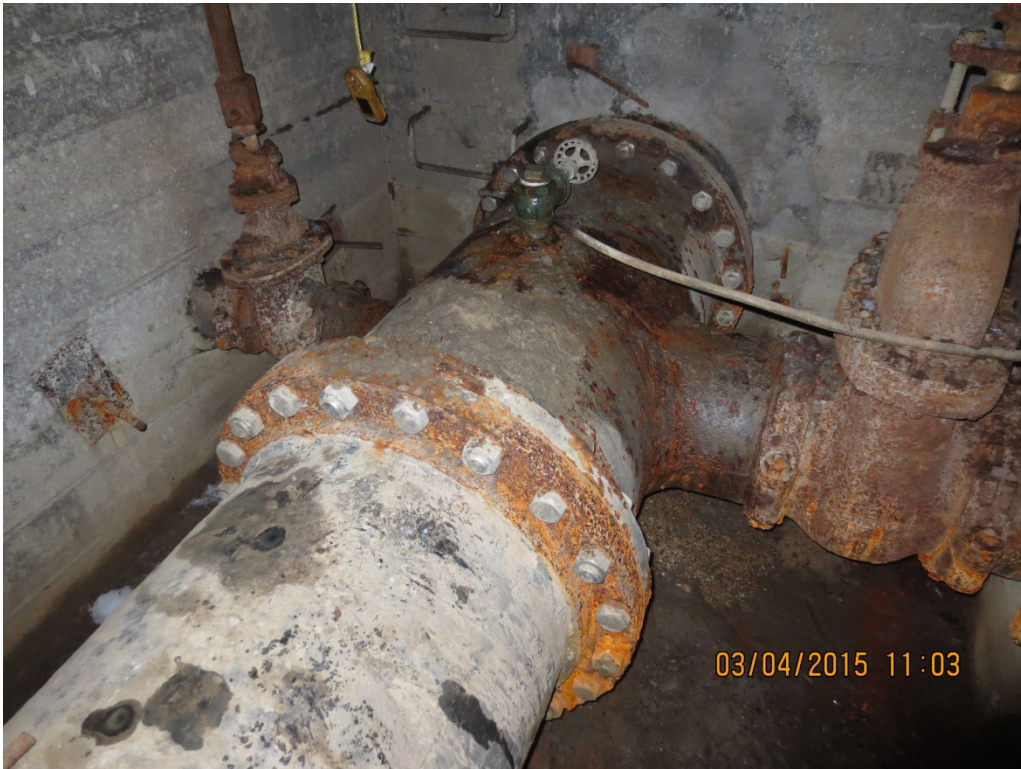
Site 1 – East chamber interior - existing cross and 300 mm offtake
