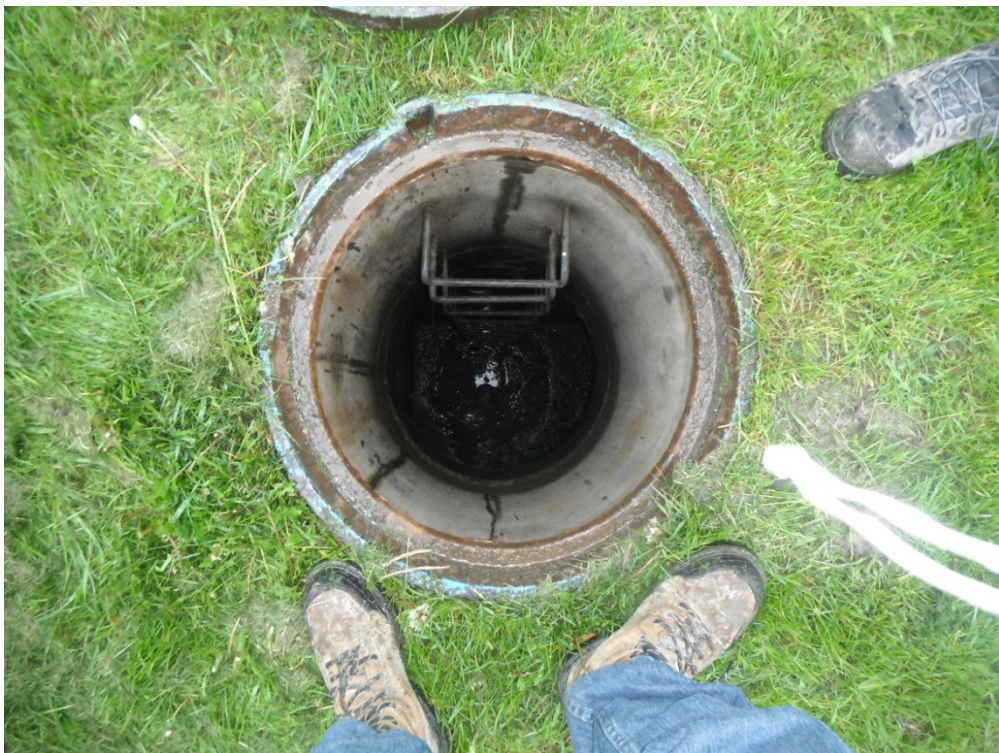
Site 2 – North chamber access.
