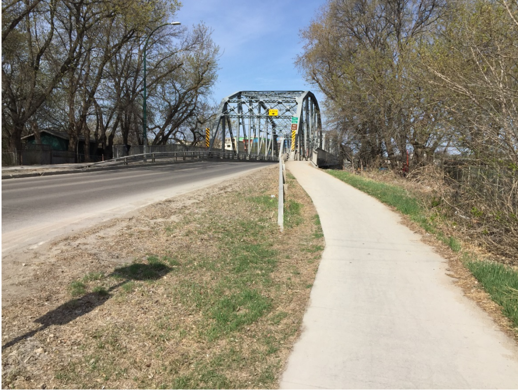
Site 1 – East site looking west towards bridge and chamber site
