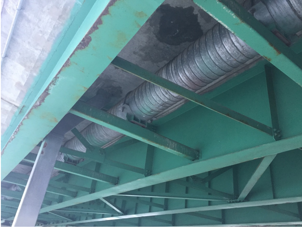
Site 3 – Force Main at underside of bridge
