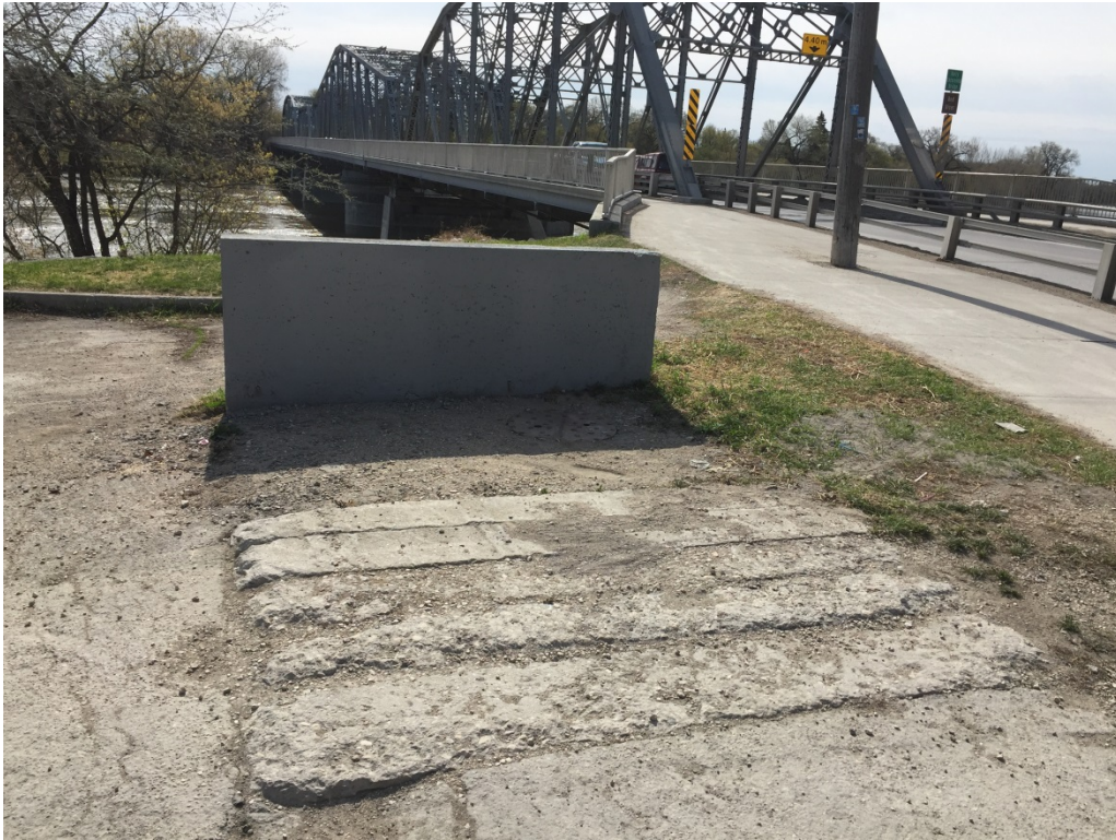
Site 1 – West chamber site top of crossing chamber
