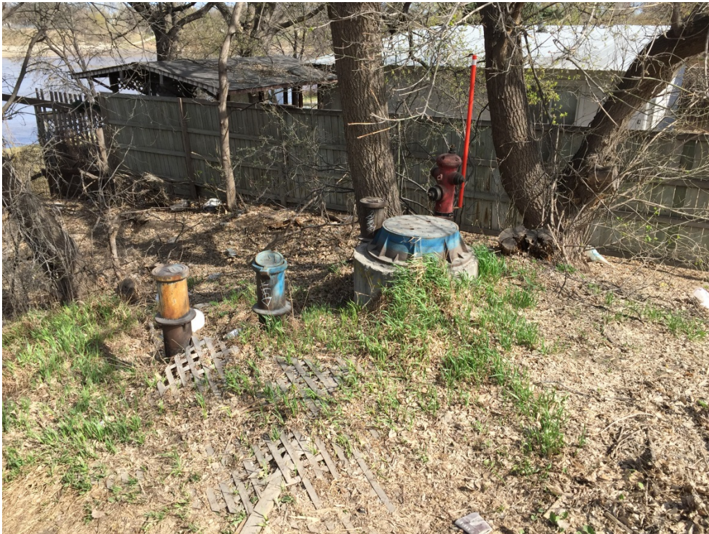
Site 1 – East chamber site looking north
