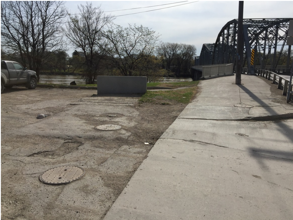
Site 1 – West chamber site looking east
