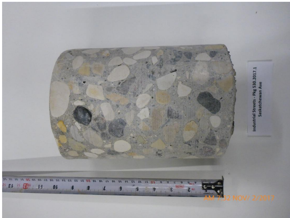
Photograph 28: Pavement Core PC17-28 – Saskatchewan Avenue
