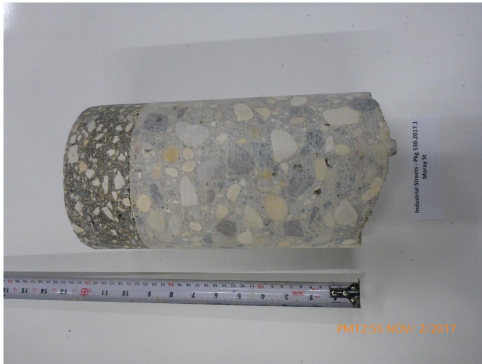
Photograph 23: Pavement Core PC17-23 – Moray Street
