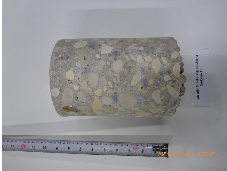
Photograph 3: Test Hole TH17-03 – Saulteaux Crescent
