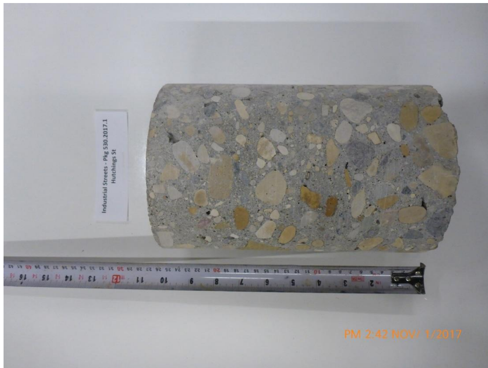
Photograph 32: Pavement Core PC17-32 – Hutchings Street
