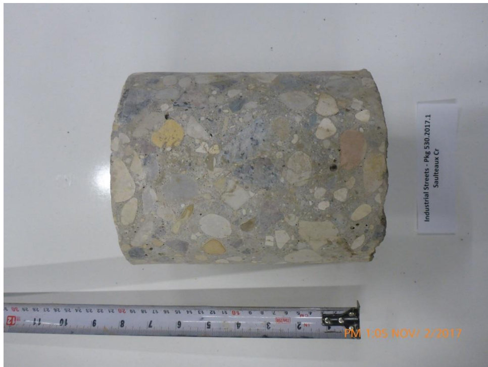
Photograph 2: Test Hole TH17-02 – Saulteaux Crescent
