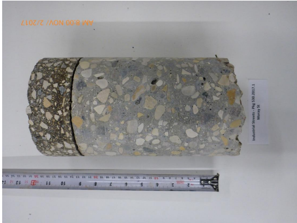
Photograph 21: Pavement Core PC17-21 – Moray Street
