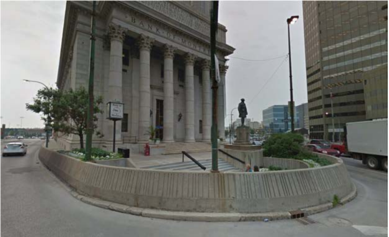
Figure 22 – Depressed Patio Area on SE corner
