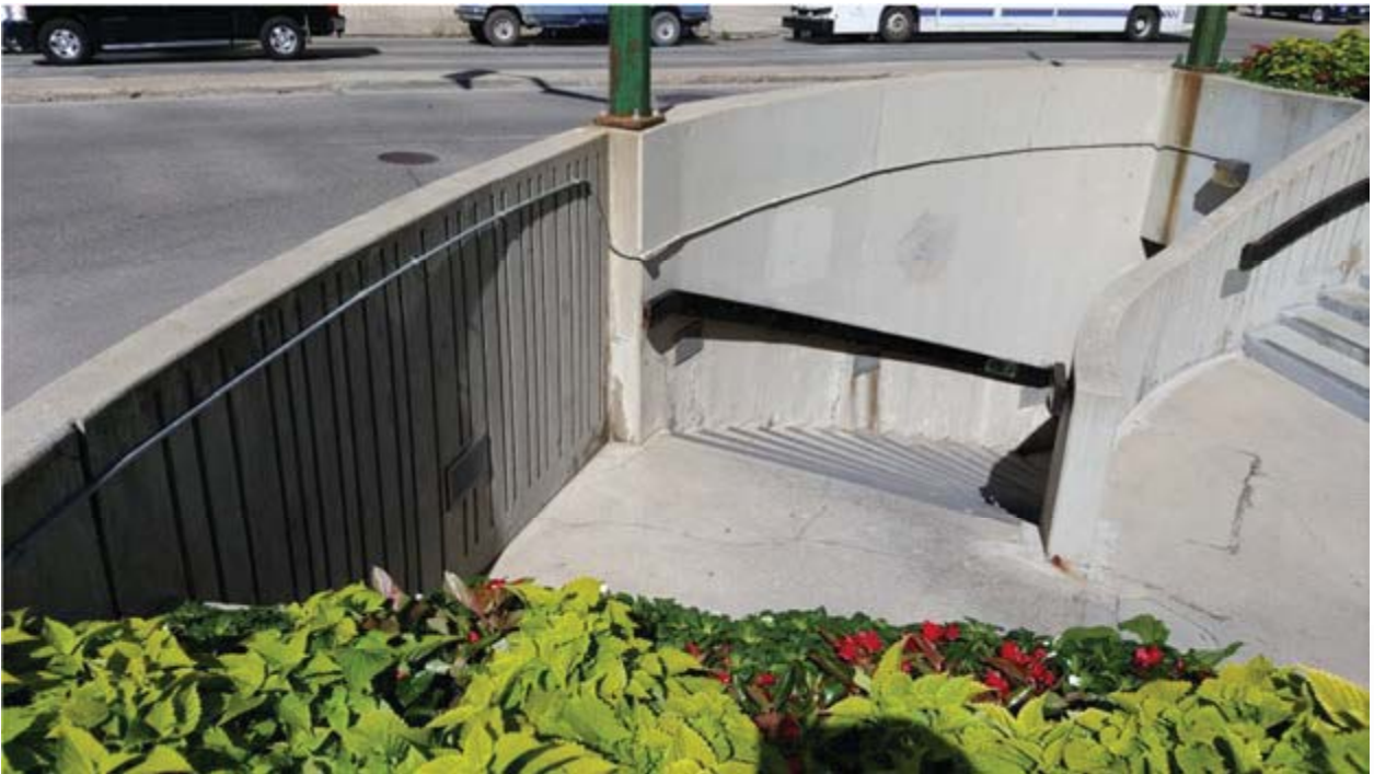
Figure 23 – Depressed Patio Area - Existing Staircase on SE corner
