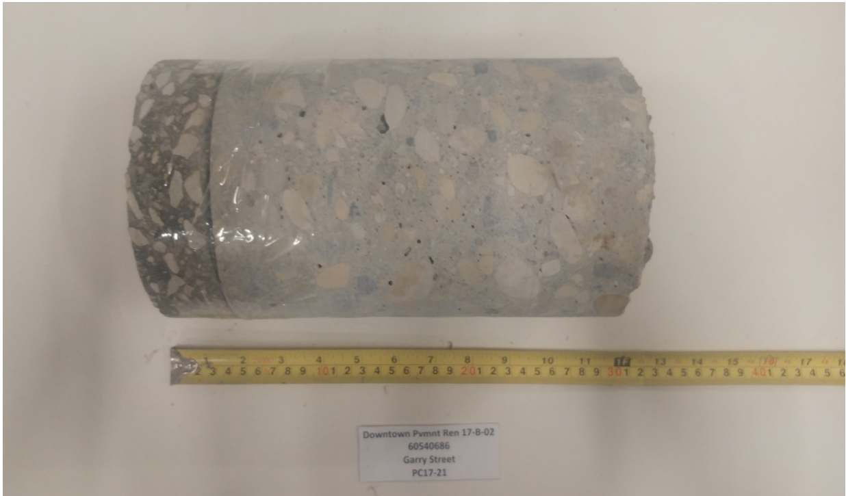
Photograph 22: Pavement Core PC17-21 – Garry Street
