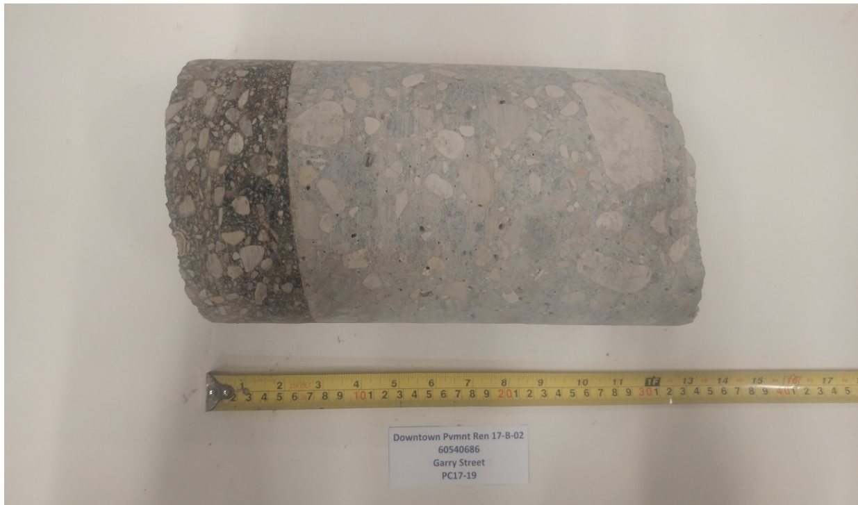
Photograph 20: Pavement Core PC17-19 – Garry Street
