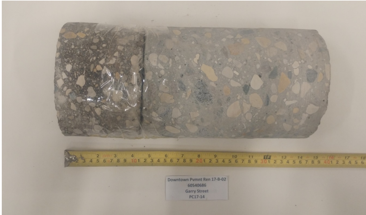
Photograph 15: Pavement Core PC17-14 – Garry Street
