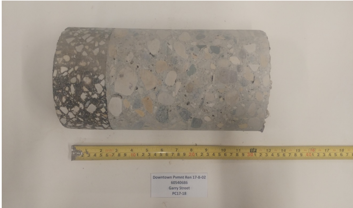
Photograph 19: Pavement Core PC17-18 – Garry Street
