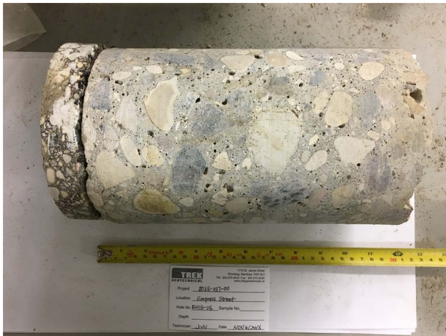
Photo 4: Pavement Core Sample at Test Hole RH16-06
