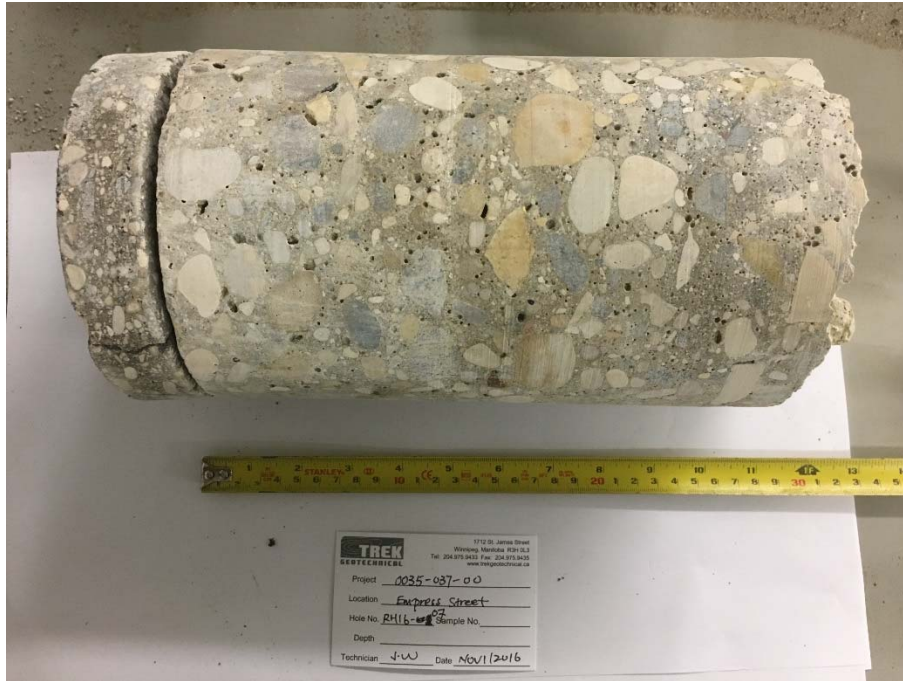
Photo 5: Pavement Core Sample at Test Hole RH16-07
