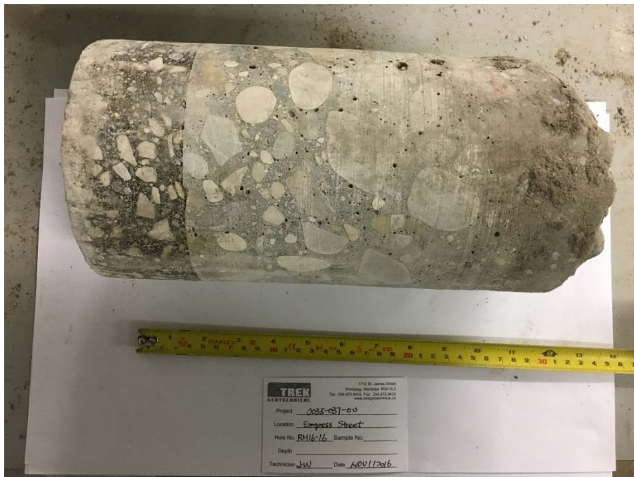
Photo 14: Pavement Core Sample at Test Hole RH16-16
