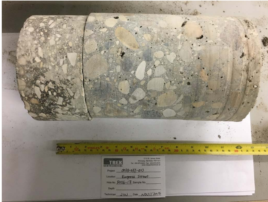
Photo 15: Pavement Core Sample at Test Hole RH16-17
