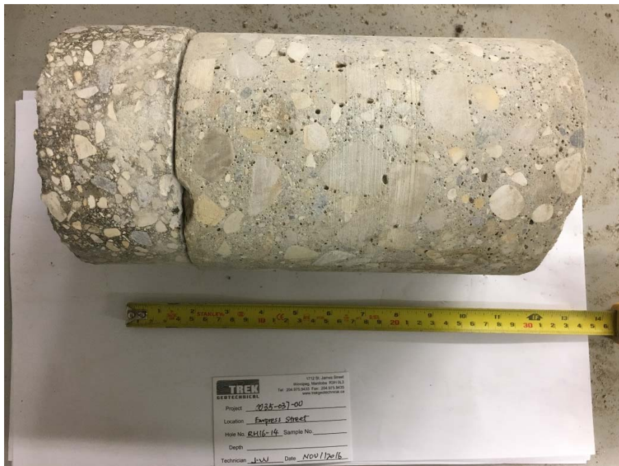
Photo 12: Pavement Core Sample at Test Hole RH16-14
