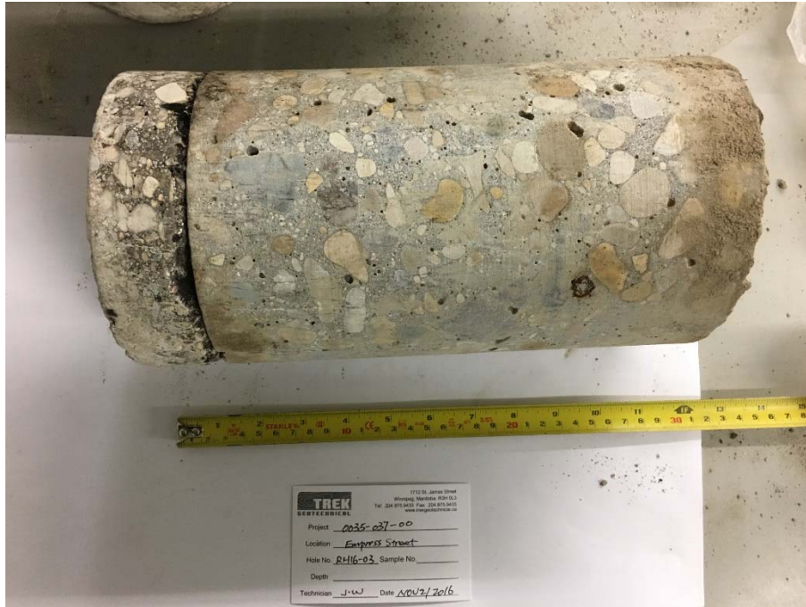
Photo 1: Pavement Core Sample at Test Hole RH16-03
