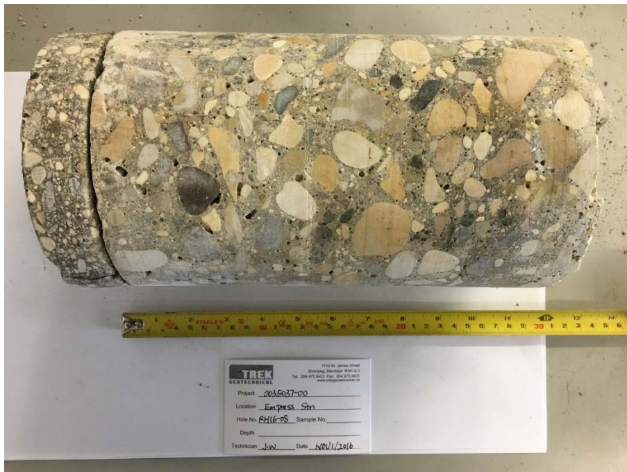
Photo 6: Pavement Core Sample at Test Hole RH16-08
