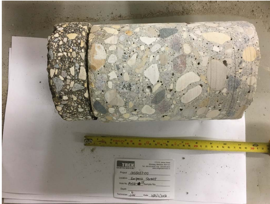
Photo 13: Pavement Core Sample at Test Hole RH16-15
