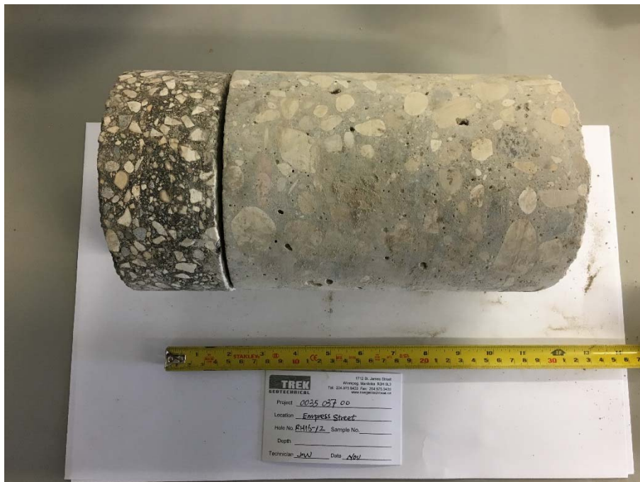
Photo 10: Pavement Core Sample at Test Hole RH16-12
