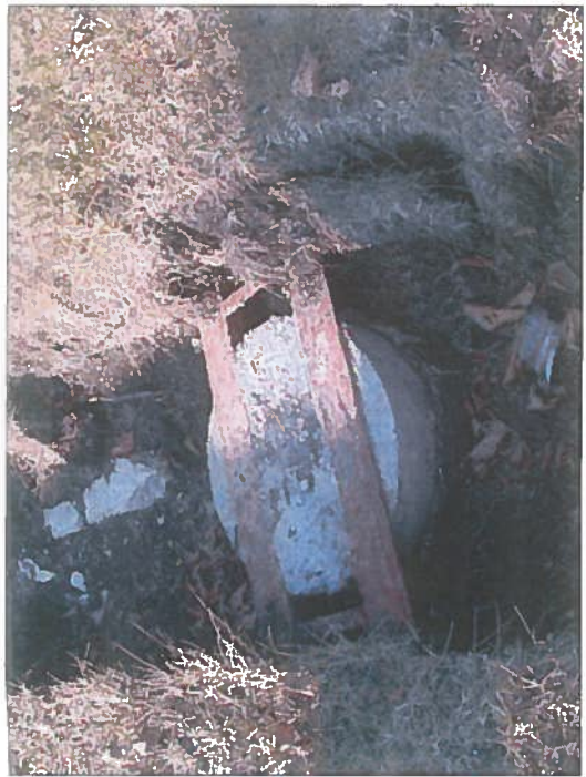
PHOTO OF EXISTING STEEL SUPPORT & CONCRETE PIER
