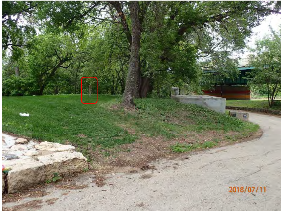
Photo 1 – Looking downslope (SE) from street side of Assiniboine Avenue to elevated upper bank area and existing Donald Outfall chamber. TH18-01 is highlighted.
