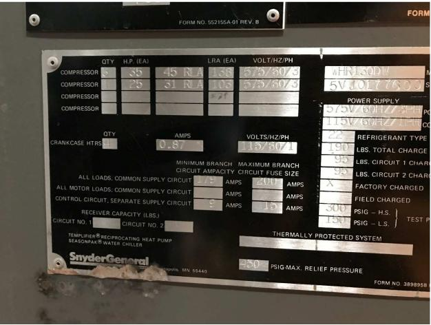
PHOTOGRAPH 2: McPhillips Regional Pumping Station – Existing chiller nameplate
