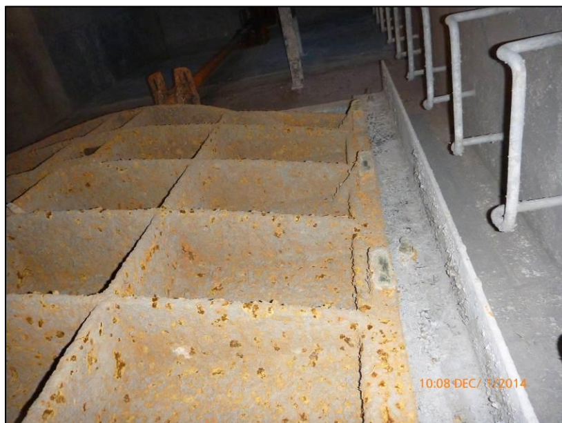
Photograph No. 8 Existing sluice and gate guide
