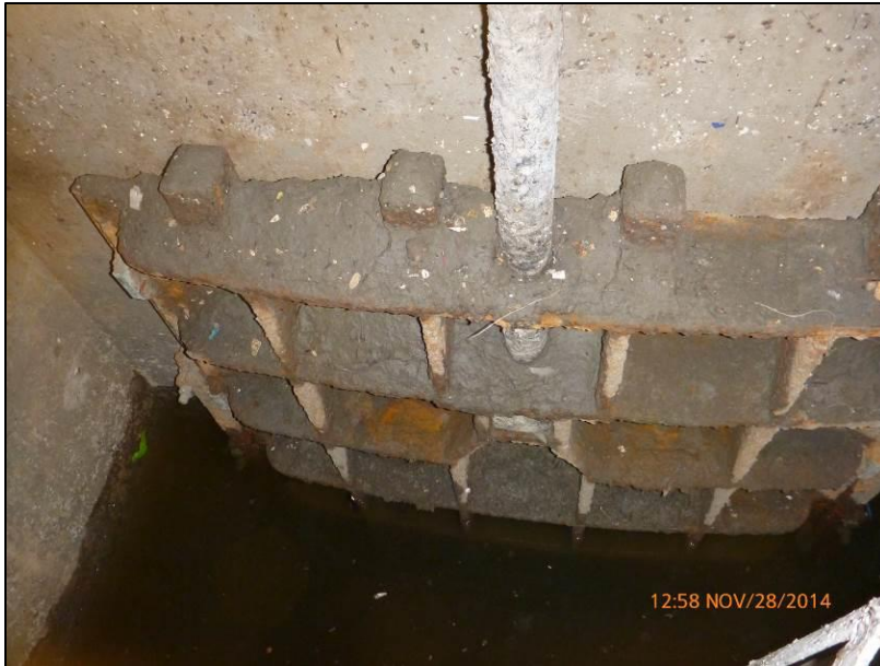
Photograph No. 9 Positive sluice gate
