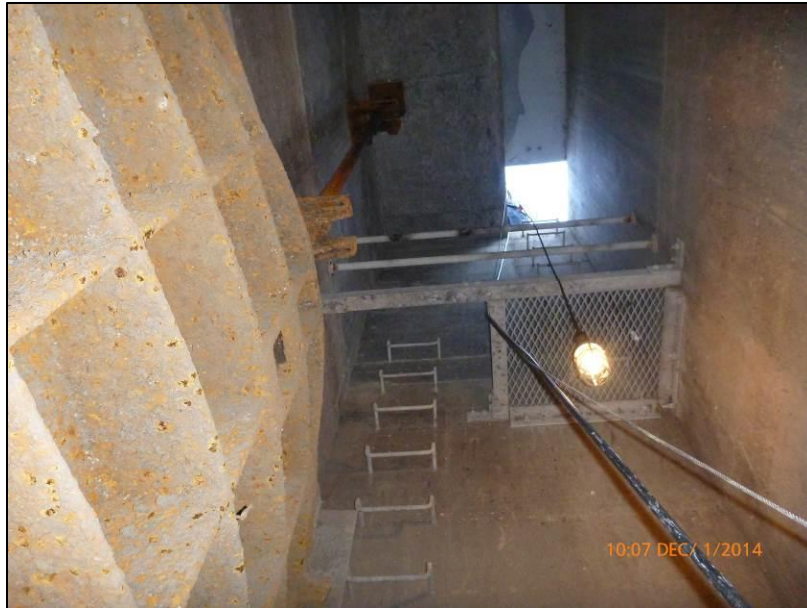
Photograph No. 7 Ladder and intermediate landing
