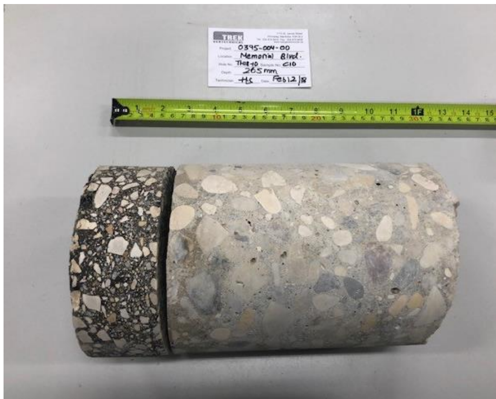
Photo 8: Pavement Core Sample at Test Hole TH18-10
