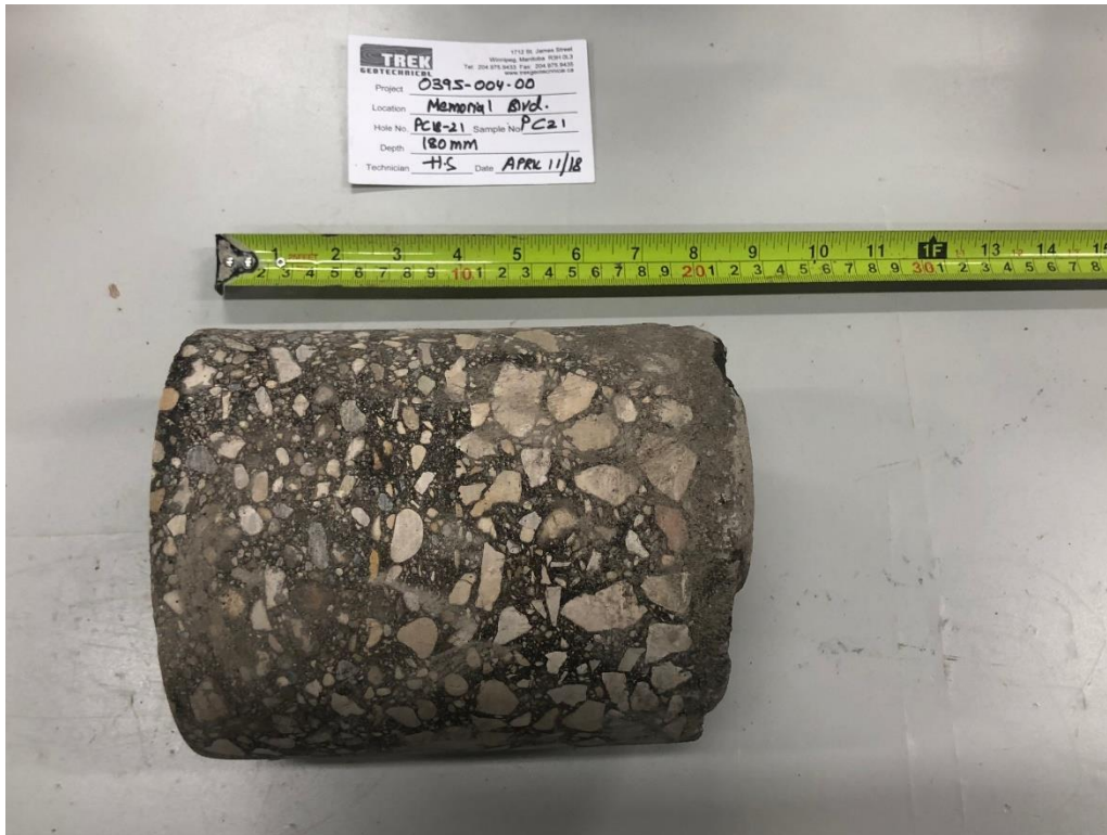
Photo 7: Pavement Core Sample at Pavement Hole PC18-21
