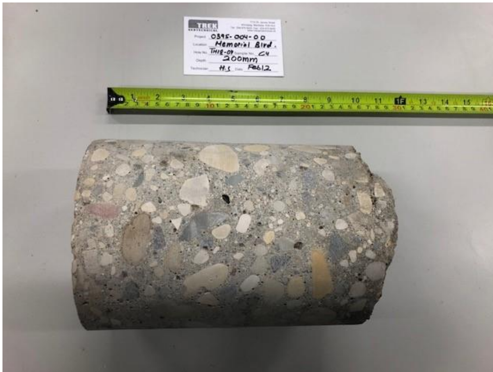
Photo 2: Pavement Core Sample at Test Hole TH18-04
