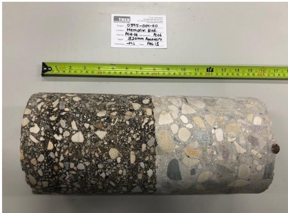
Photo 6: Pavement Core Sample at Pavement Hole PC18-06
