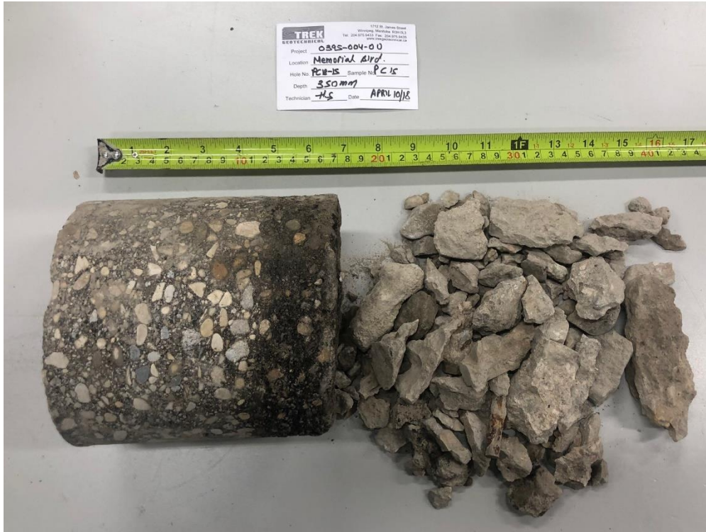
Photo 1: Pavement Core Sample at Pavement Hole PC18-15
