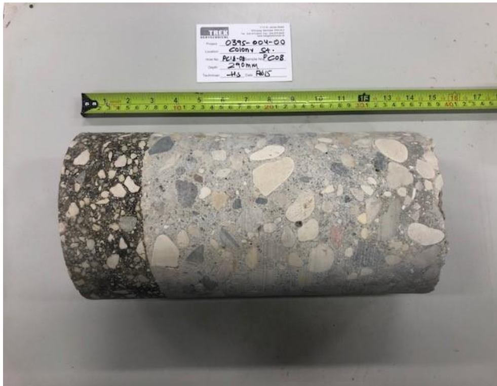
Photo 2: Pavement Core Sample at Pavement Hole PC18-08
