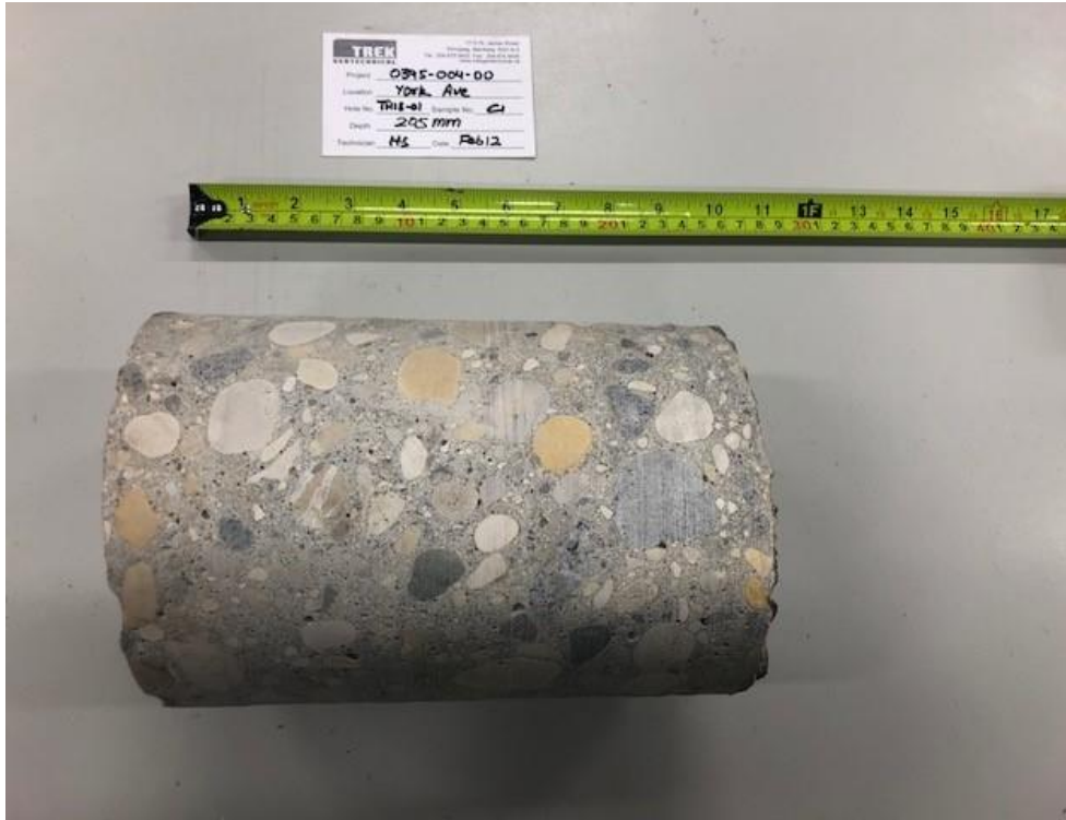
Photo 1: Pavement Core Sample at Test Hole TH18-01
