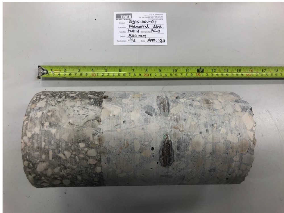
Photo 4: Pavement Core Sample at Pavement Hole PC18-18
