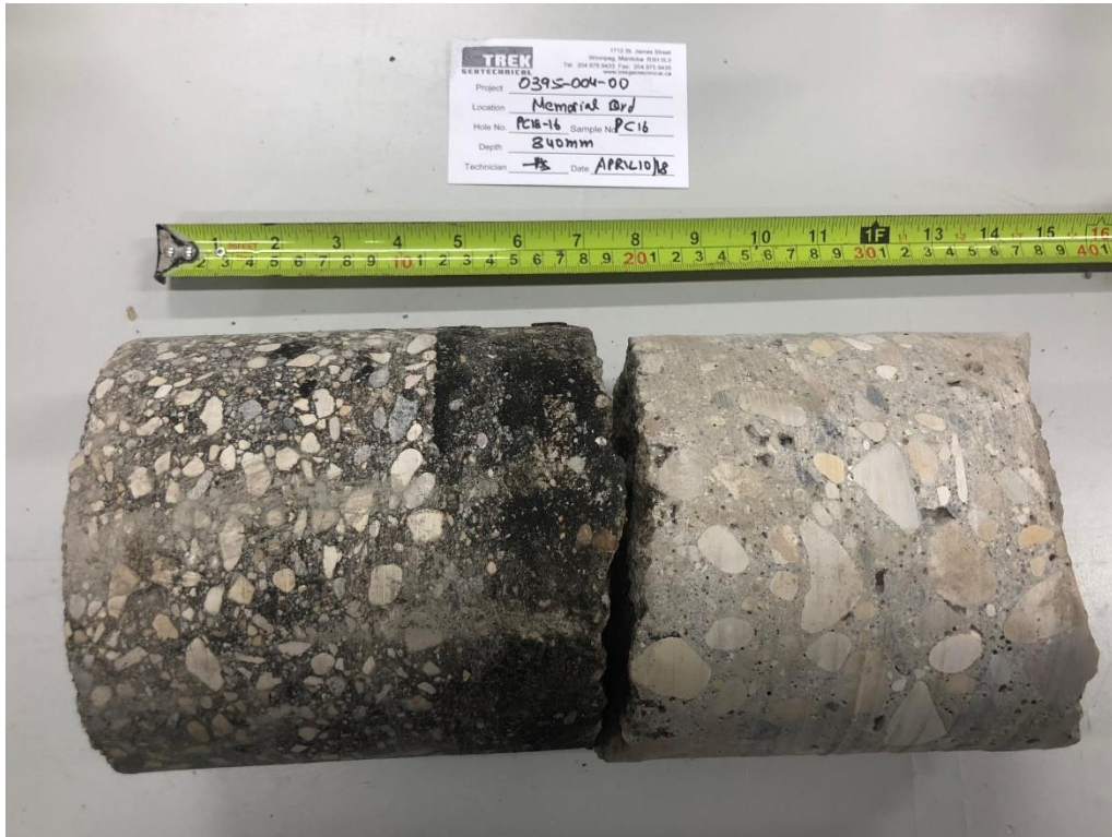
Photo 2: Pavement Core Sample at Pavement Hole PC18-16
