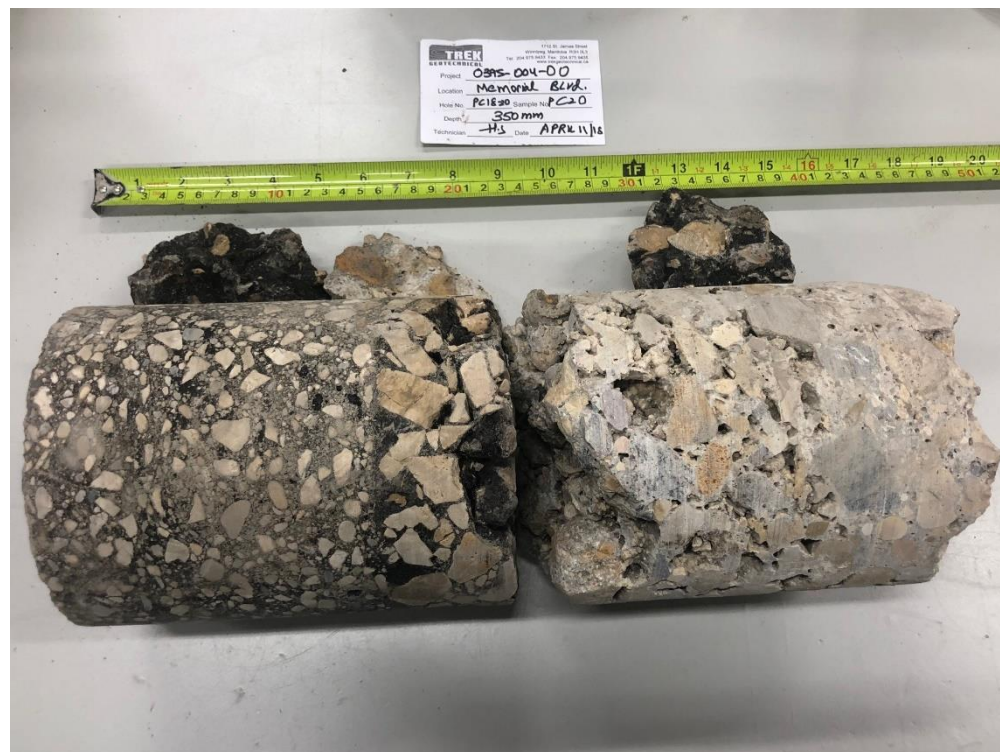
Photo 6: Pavement Core Sample at Pavement Hole PC18-20
