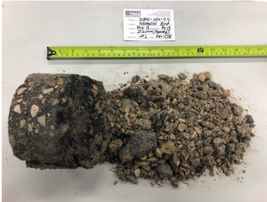
Photo 7: Pavement Core Sample at Pavement Hole PC18-13
