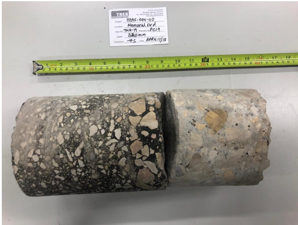
Photo 5: Pavement Core Sample at Pavement Hole PC18-19
