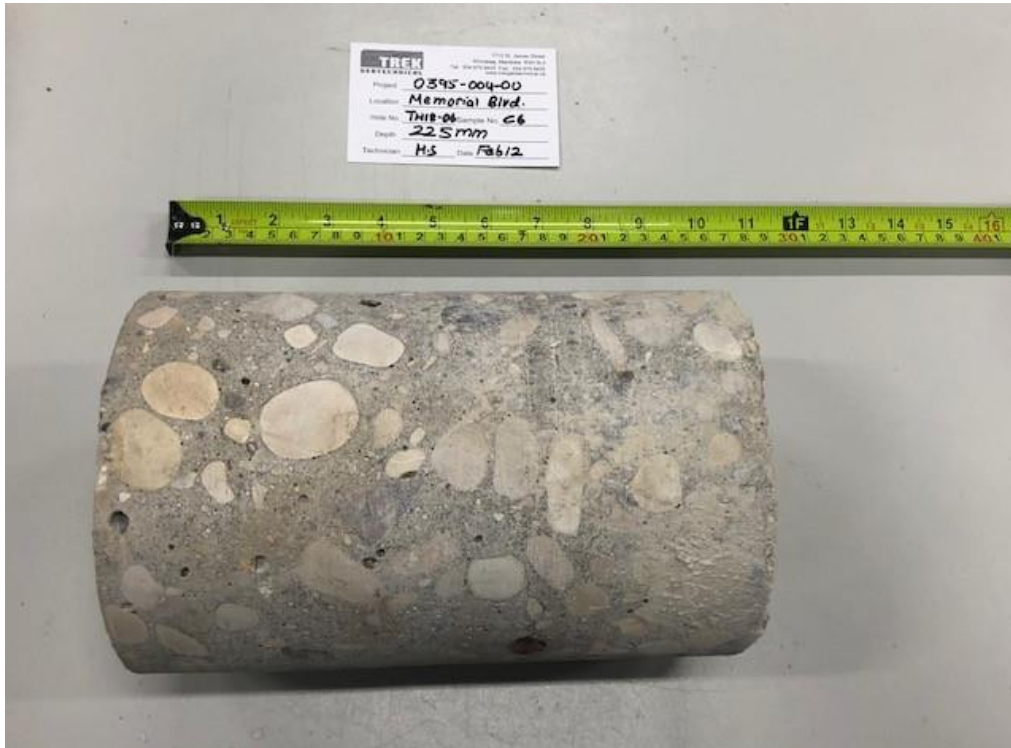
Photo 4: Pavement Core Sample at Test Hole TH18-06
