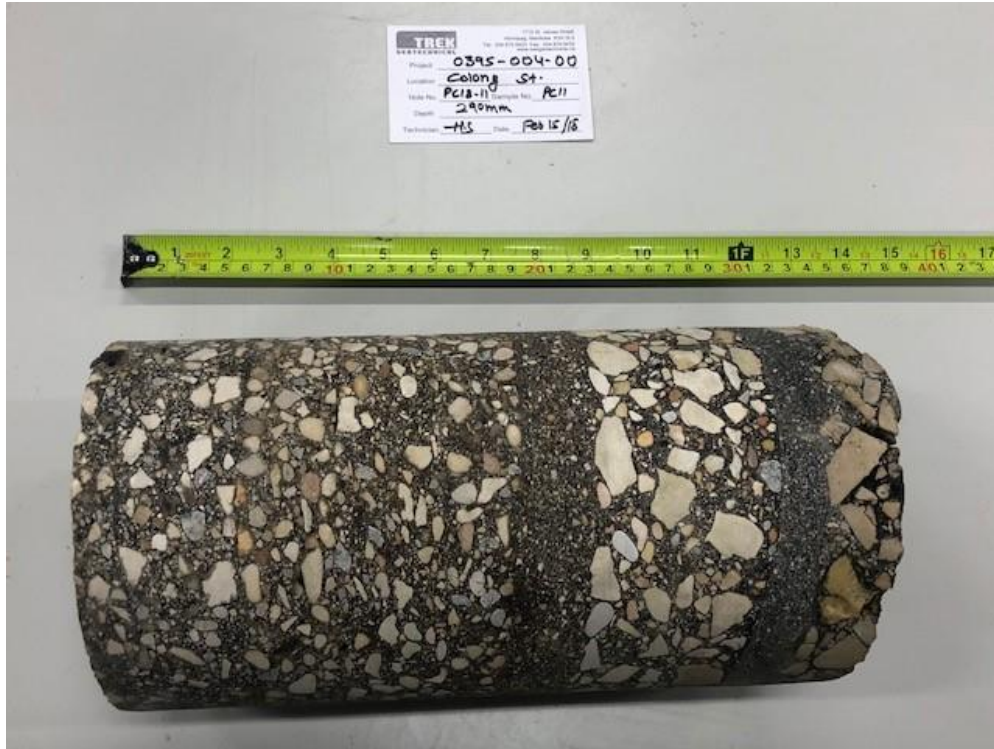
Photo 5: Pavement Core Sample at Pavement Hole PC18-11
