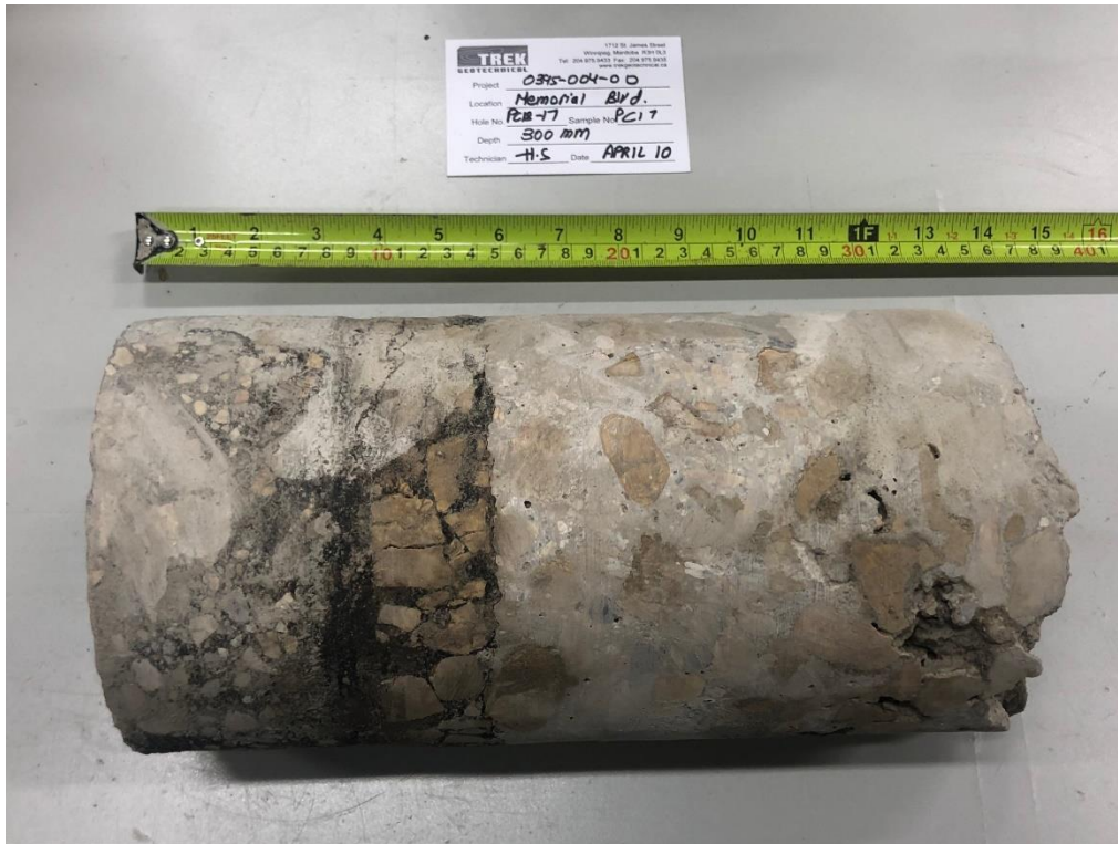
Photo 3: Pavement Core Sample at Pavement Hole PC18-17
