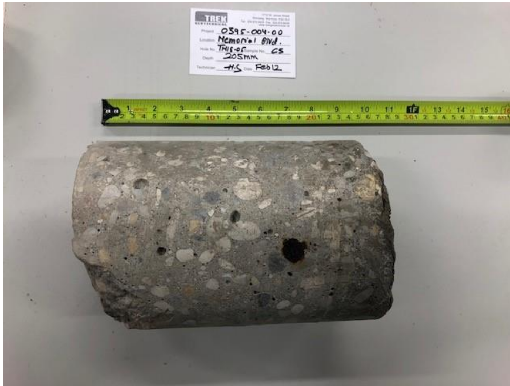
Photo 3: Pavement Core Sample at Test Hole TH18-05
