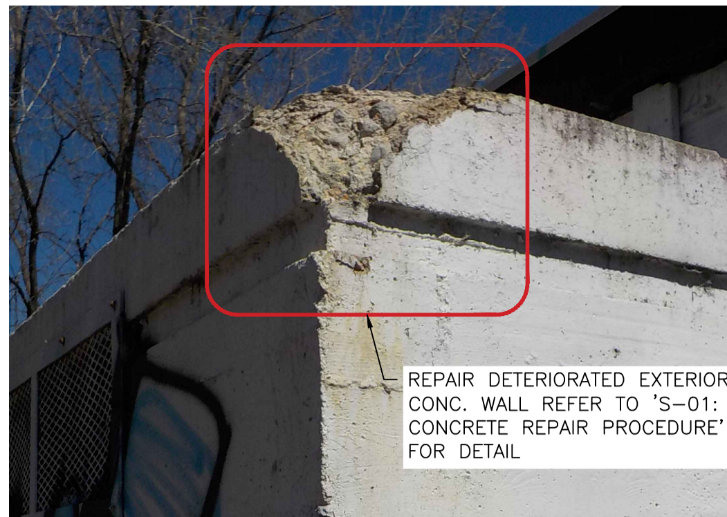
1 DETERIORATED CONC. REPAIR DETAIL S-07
