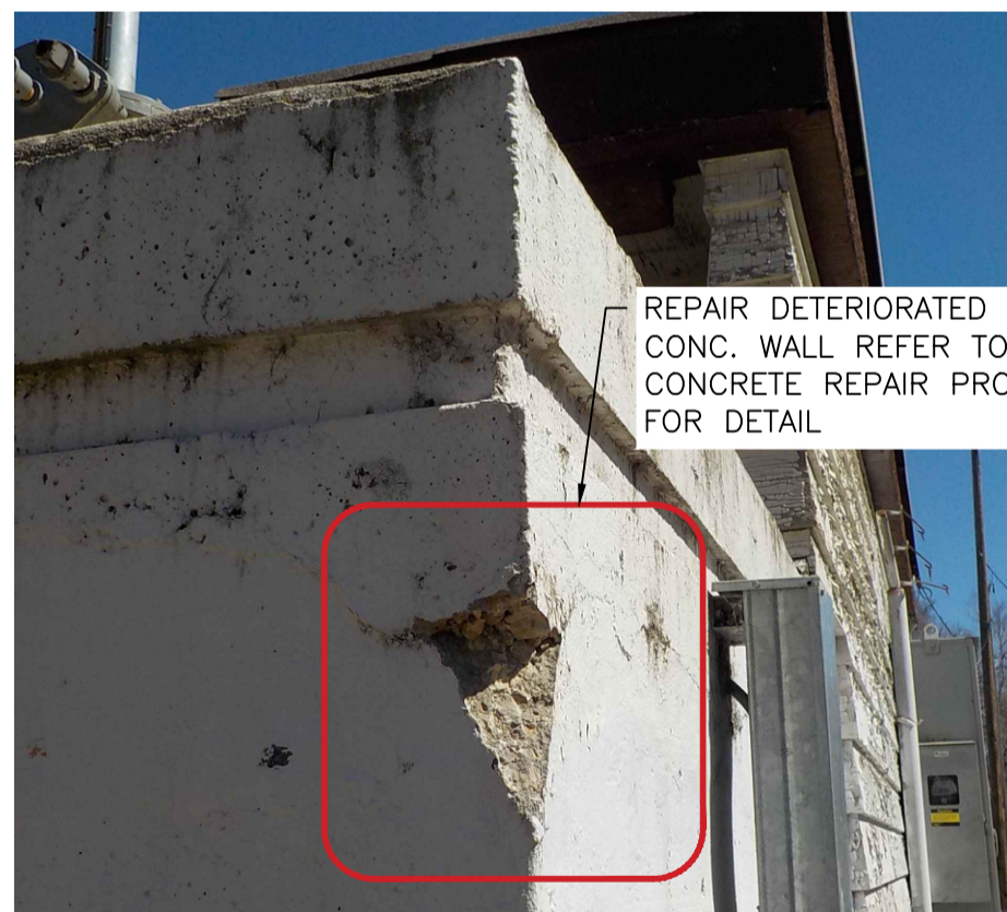
3 DETERIORATED CONC. REPAIR DETAIL S-07
