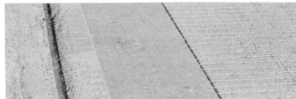
Figure 8 – PCC Light Corduroy or ribbed pattern made with properly spaced, gang stacked cutting blades.
