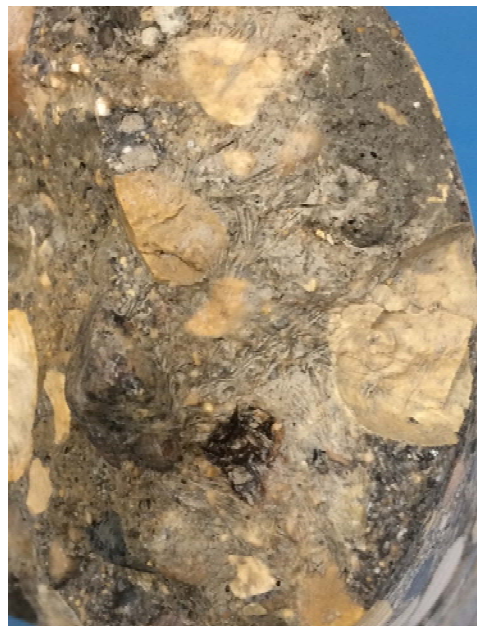
Figure 4 - Core no. 3 (frost/rootlets)
