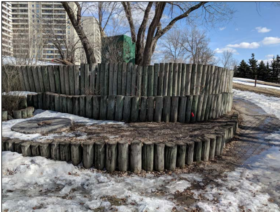
PHOTO 1 LODGE AVENUE OUTFALL – EXISTING RETAINING WALL STRUCTURE
