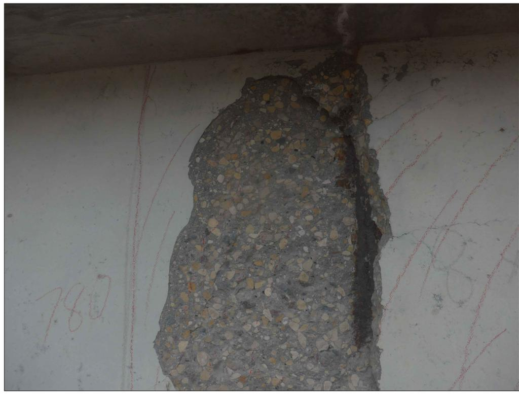
TYPICAL DELAMINATION ON NORTHBOUND BRIDGE SPANDREL WALL
