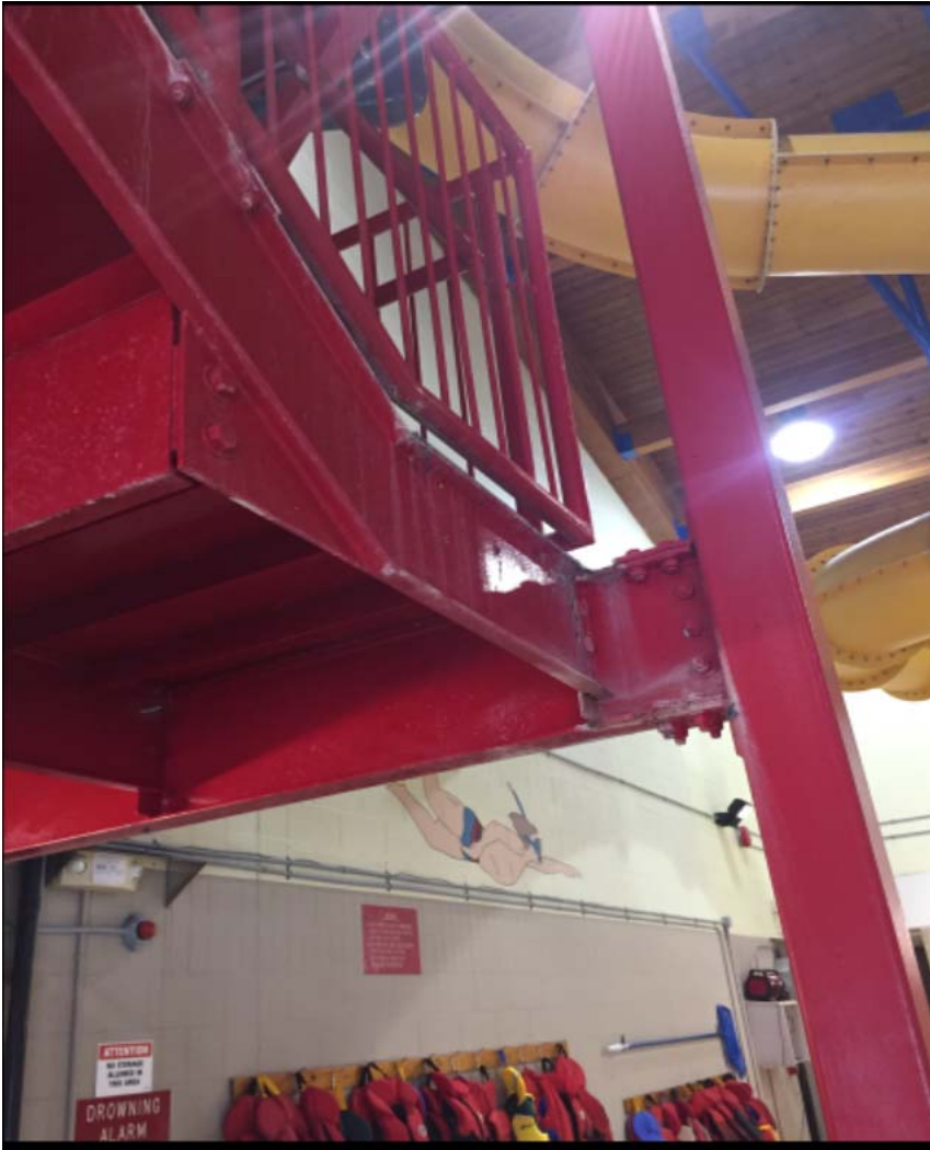
Image 1: Steel Tower Support Column/Beam Connections
