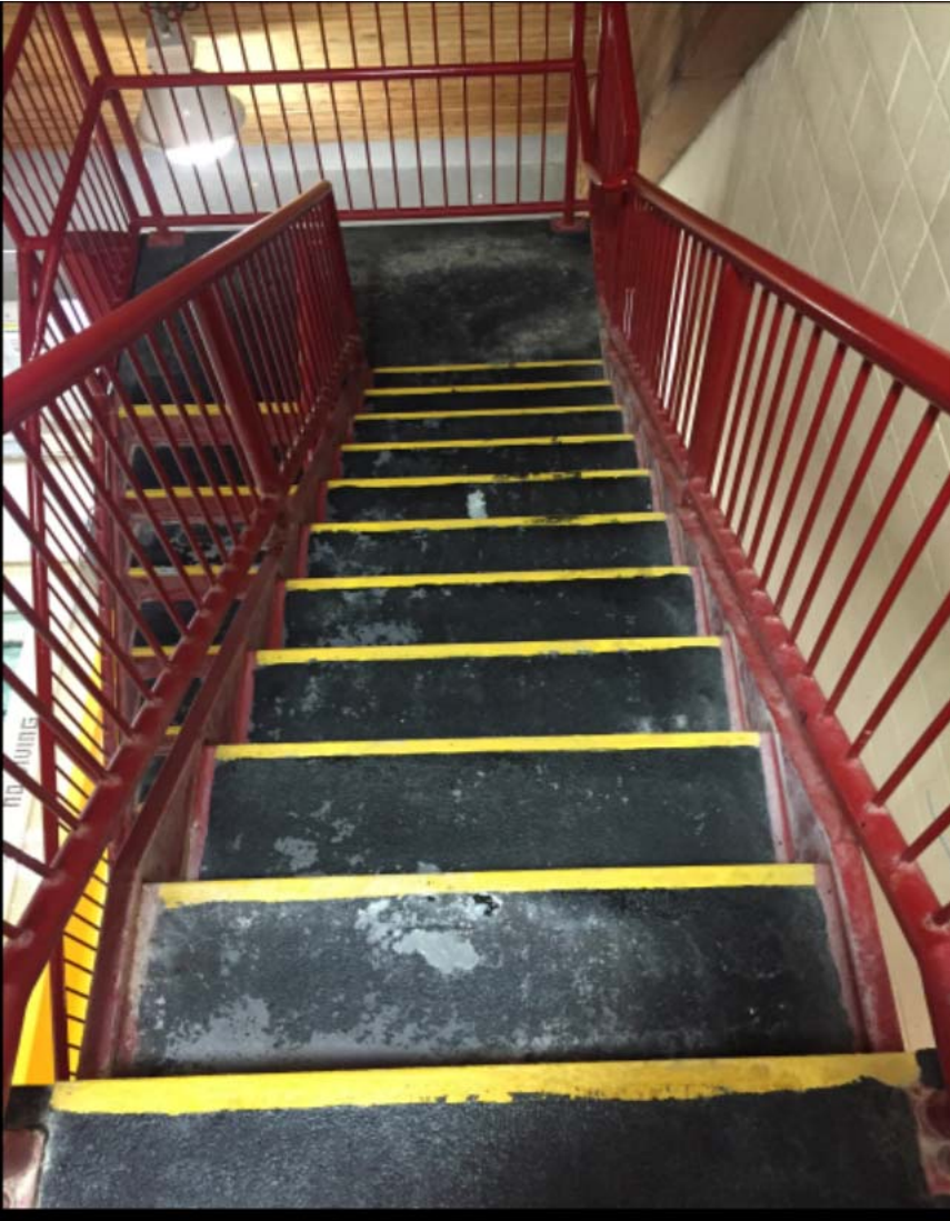
Image 9: View from Top of Stair Trads and Tower Landing
