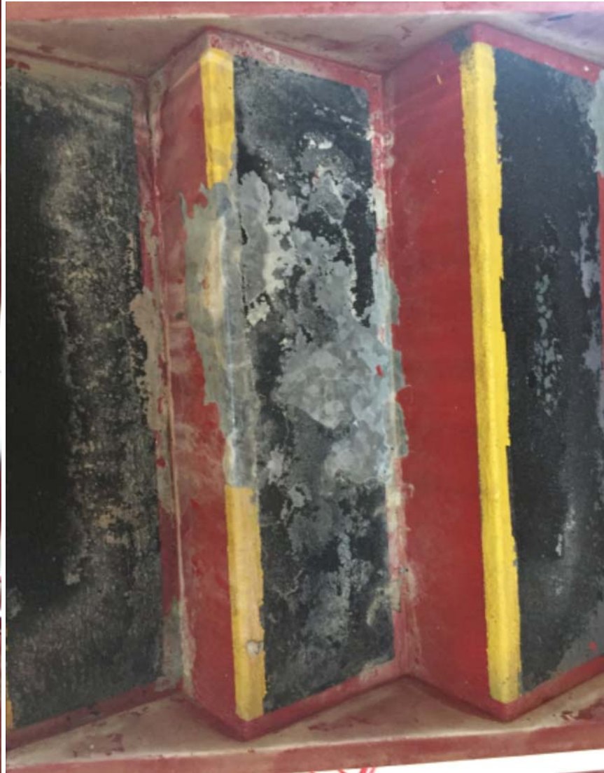
Image 6: View of exposed galvanized finish beneath power coat paint finishes
