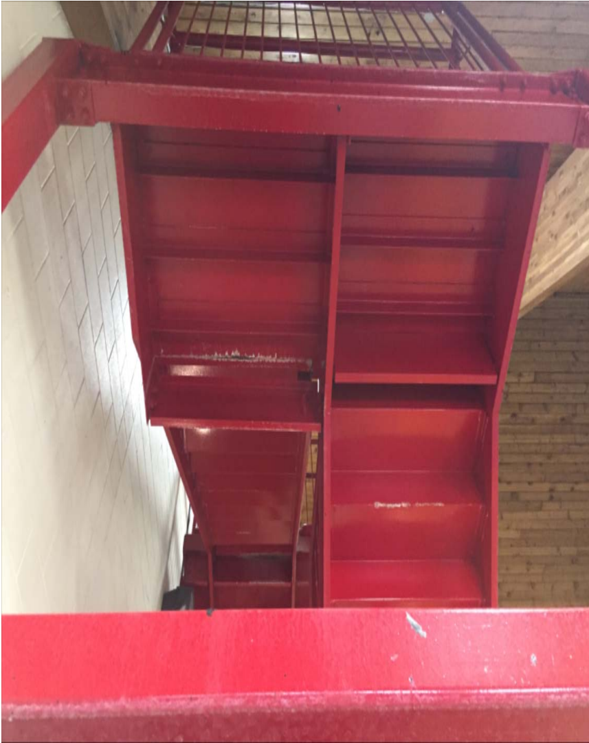
Image 7: View of underside pan of waterslide steel stairs
