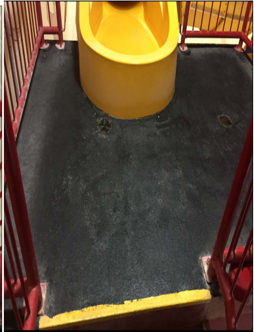
Image 10: Top View of Highest Waterslide Tower Landing
