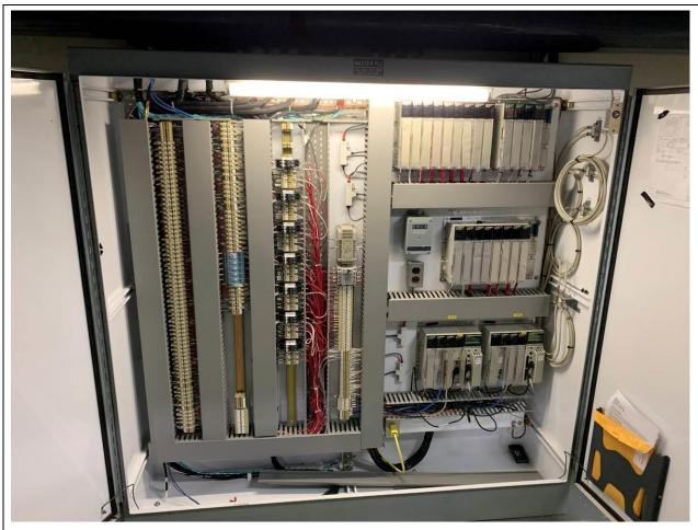
PHOTOGRAPH 31: DBPS UV Master PLC panel interior.
