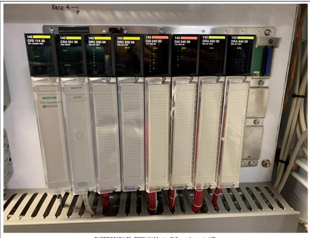
PHOTOGRAPH 35: DBPS UV Master PLC panel remote I/O.
