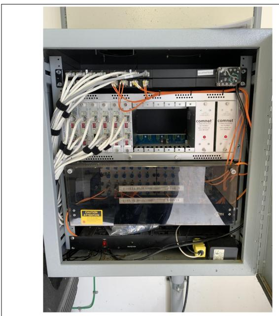
PHOTOGRAPH 86: SLAIF Electrical Shed network panel NP-H800 interior showing the existing network media converter.
