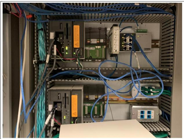
PHOTOGRAPH 47: SLAIF control room main alarm panel PL-15 redundant station PLCs.
