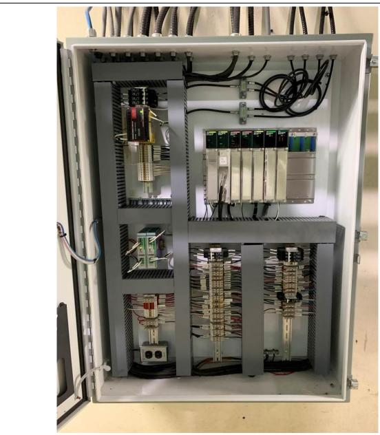
PHOTOGRAPH 22: DBPS local control panel LCP-D12 interior.
