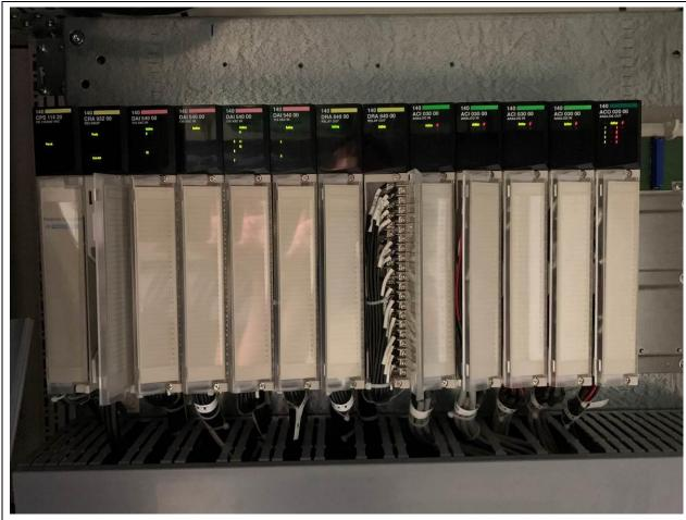
PHOTOGRAPH 29: DBPS control panel CP-D21 Quantum remote I/O.
