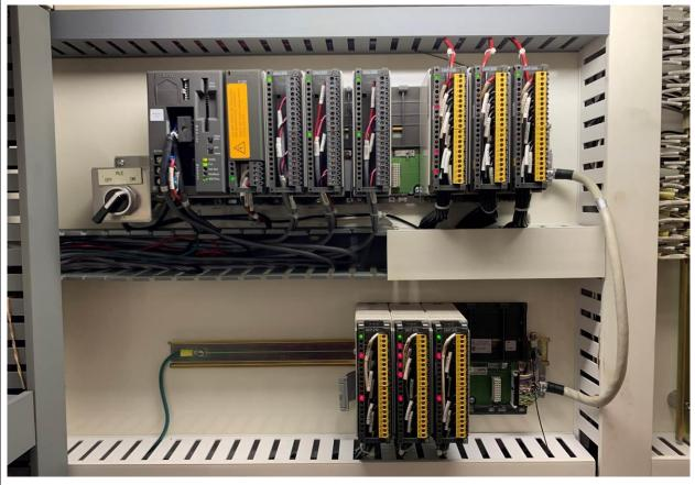
PHOTOGRAPH 4: Hurst RPS pump 15 local control panel LCP-15 interior showing the pump PLC.
