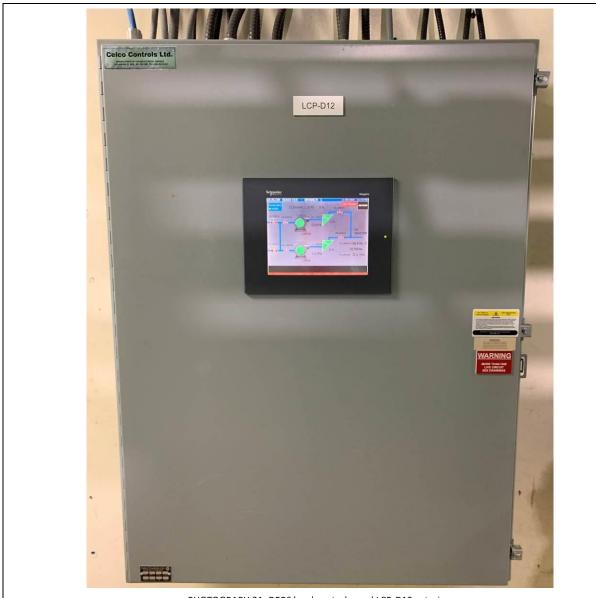
PHOTOGRAPH 21: DBPS local control panel LCP-D12 exterior.
