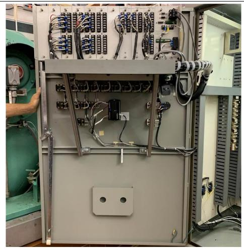
PHOTOGRAPH 3: Hurst RPS pump 15 local control panel LCP-15 facing the rear of the door panel showing the connections on the Bently Nevada pump and motor condition monitoring unit.
