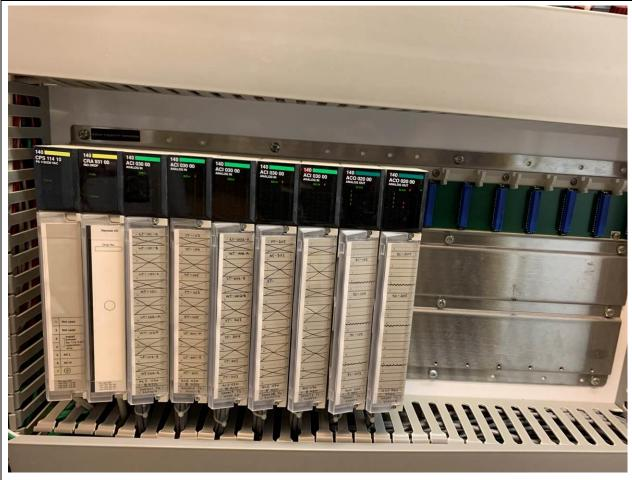
PHOTOGRAPH 41: DCFF main control panel remote I/O.
