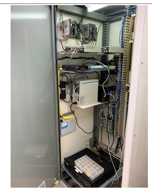
PHOTOGRAPH 7: Hurst RPS main control panel left side interior showing station PLCs and Modbus+ equipment.
