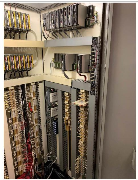
PHOTOGRAPH 19: MacLean RPS main control panel right side interior showing station analog I/O and terminal block wiring.
