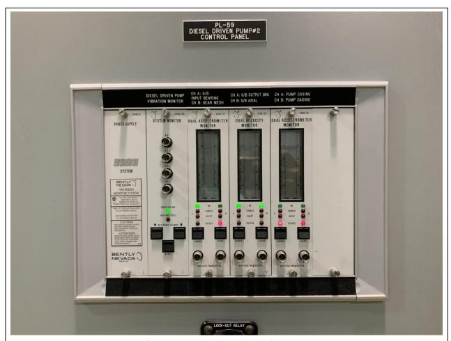
PHOTOGRAPH 70: SLAIF pump room low lift pump #2 control panel PL-59 exterior showing the Bently Nevada pump and motor condition monitoring unit.
