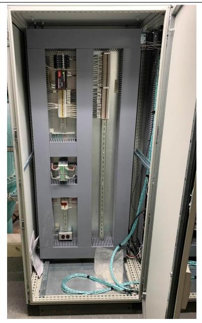
PHOTOGRAPH 26: DBPS control panel CP-D21 left interior section.
