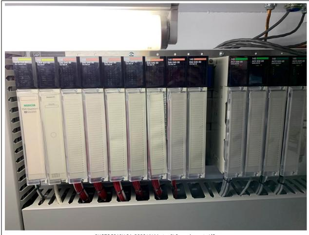
PHOTOGRAPH 34: DBPS UV Master PLC panel remote I/O.
