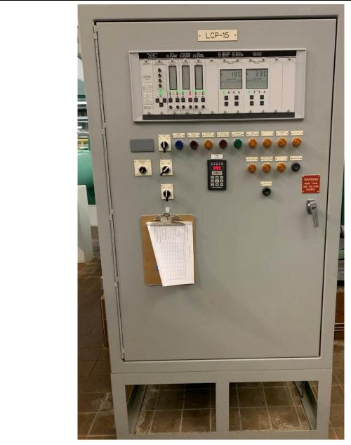
PHOTOGRAPH 1: Hurst RPS pump 15 local control panel LCP-15 exterior.
