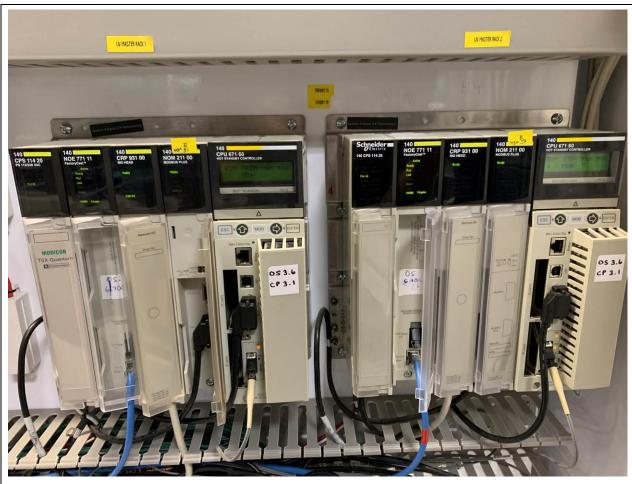
PHOTOGRAPH 36: DBPS UV Master PLC panel Quantum redundant PLCs.
