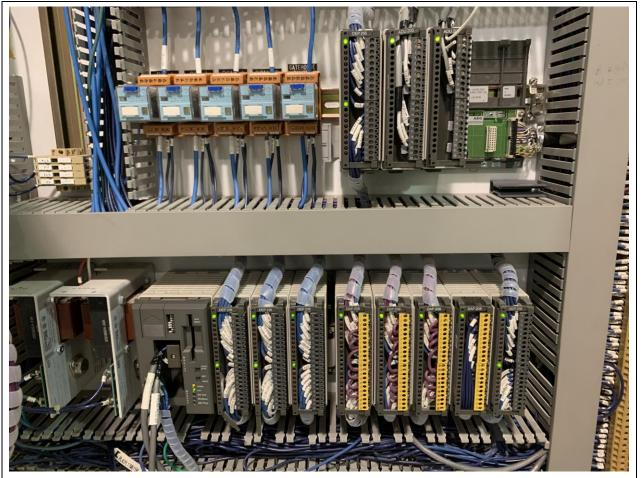
PHOTOGRAPH 65: SLAIF pump room alarm panel PL-17 PLC 30.
