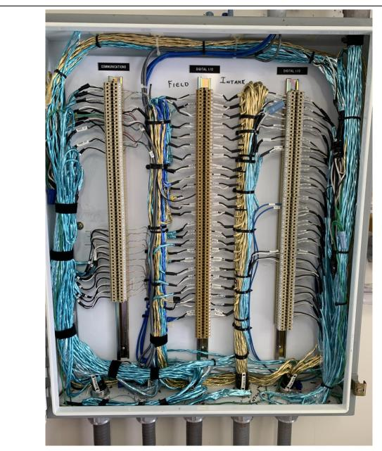
PHOTOGRAPH 88: SLAIF Electrical Shed panel PL-64 interior showing extisting terminal block wiring.
