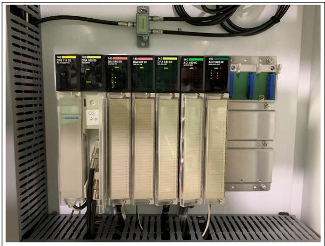
PHOTOGRAPH 24: DBPS local control panel LCP-D12 Quantum remote I/O.
