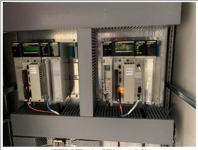
PHOTOGRAPH 30: DBPS control panel CP-D21 Quantum redundant PLCs.
