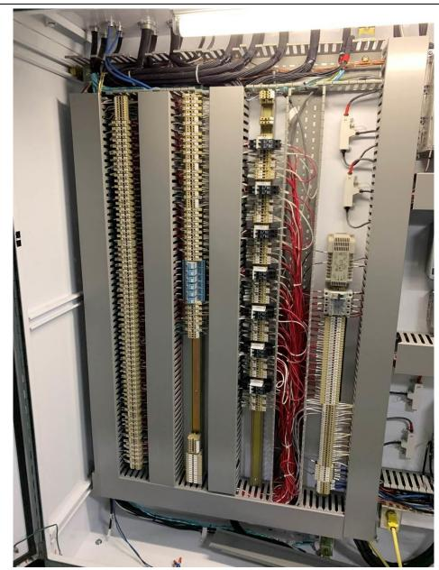
PHOTOGRAPH 32: DBPS UV Master PLC panel left side interior showing terminal block wiring.
