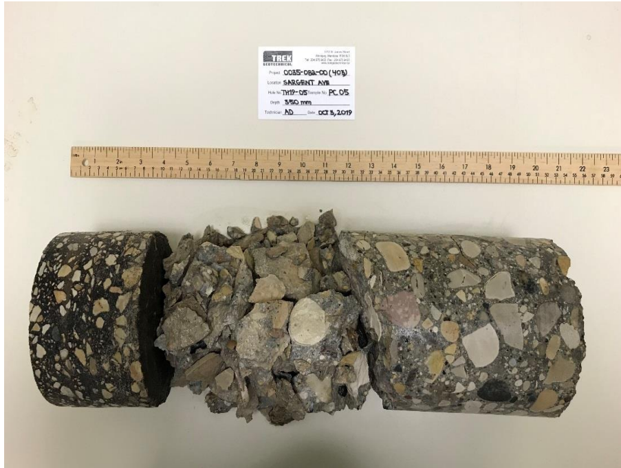
Photo 5: Pavement Core Sample at Test Hole TH19-05
