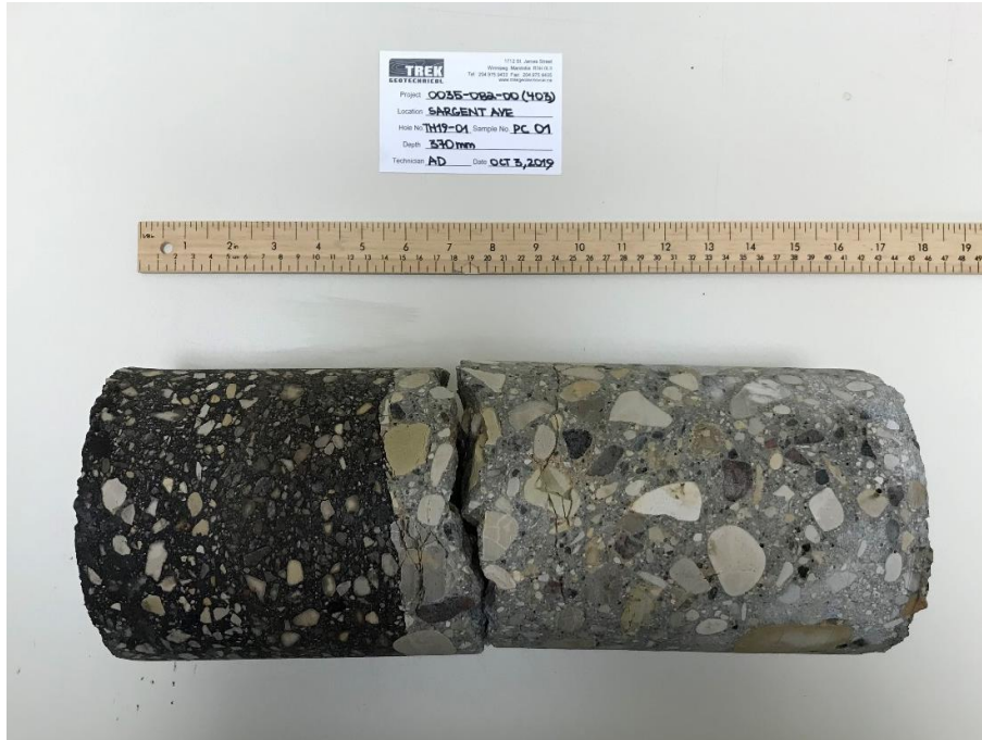
Photo 1: Pavement Core Sample at Test Hole TH19-01
