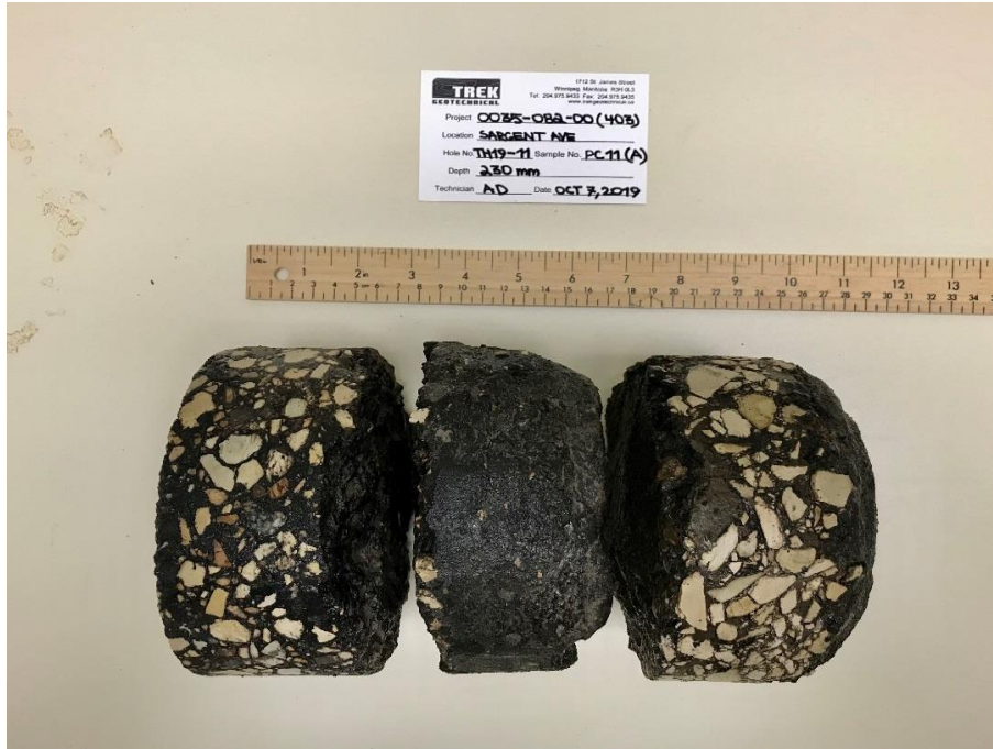
Photo 11: Pavement Core Sample at Test Hole TH19-11A
