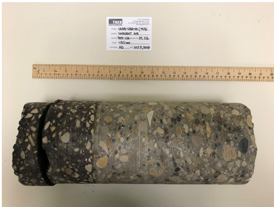
Photo 2: Pavement Core Sample at Test Hole TH19-02
