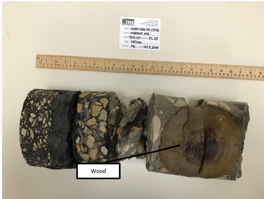
Photo 7: Pavement Core Sample at Test Hole TH19-07
