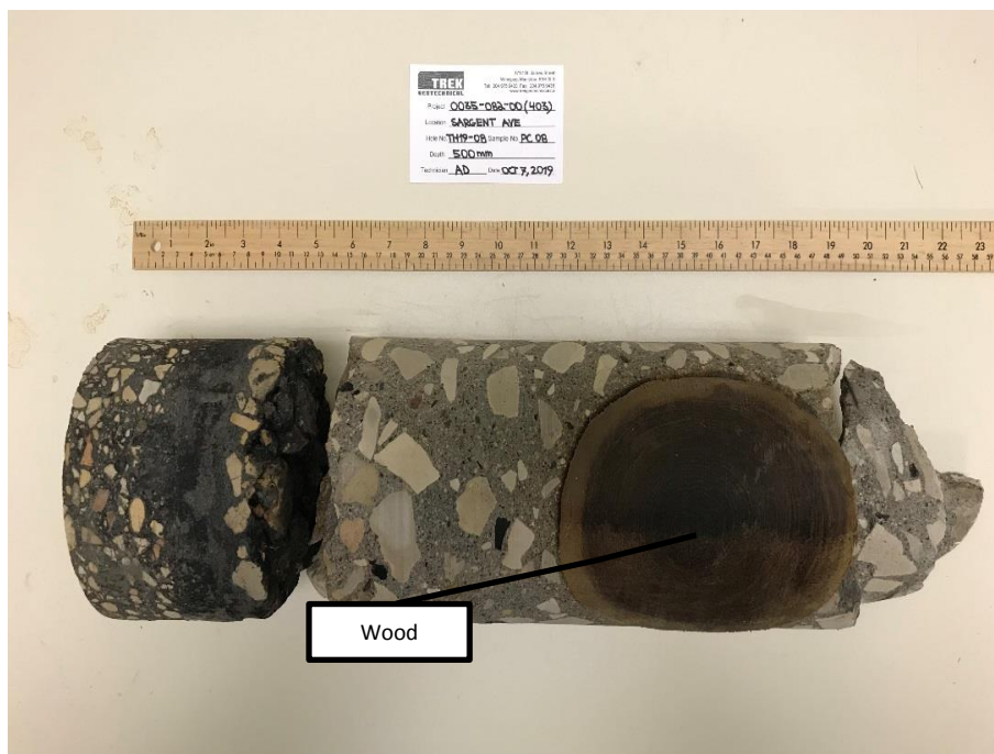
Photo 8: Pavement Core Sample at Test Hole TH19-08
