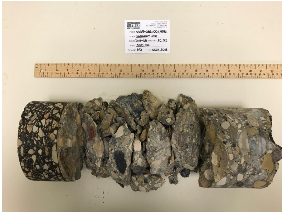
Photo 3: Pavement Core Sample at Test Hole TH19-03
