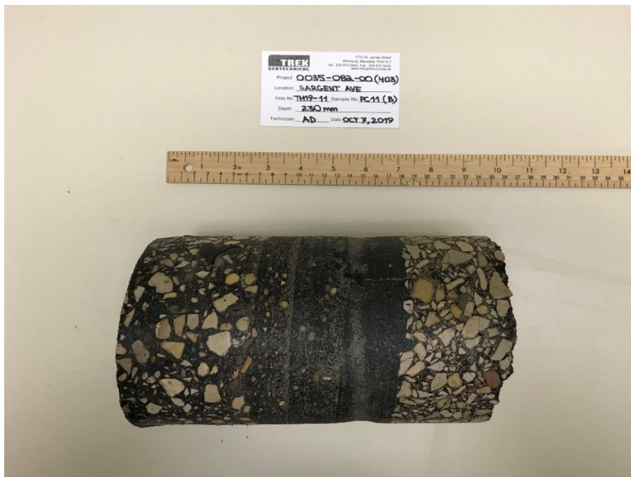
Photo 12: Pavement Core Sample at Test Hole TH19-11B
