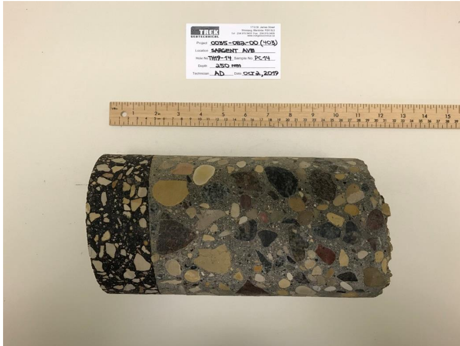
Photo 15: Pavement Core Sample at Test Hole TH19-14
