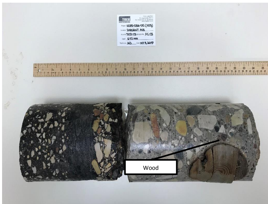
Photo 14: Pavement Core Sample at Test Hole TH19-13
