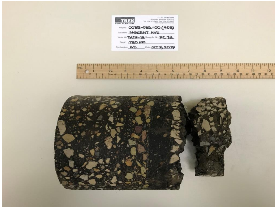
Photo 13: Pavement Core Sample at Test Hole TH19-12
