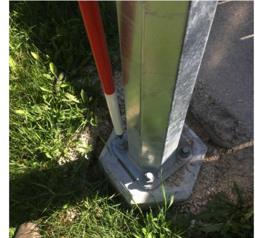
TBM 1: Top of southeast nut of streetlight base
