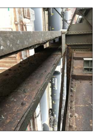
EXISTING CONDITION OF TRUSS BOTTOM CHORD AT SPAN 19 - BAY 4
