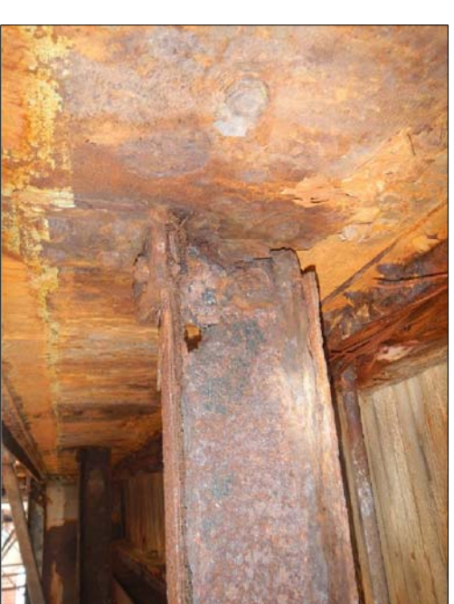
EXISTING CONDITION OF A DIAPHRAGM AT SPAN 30
