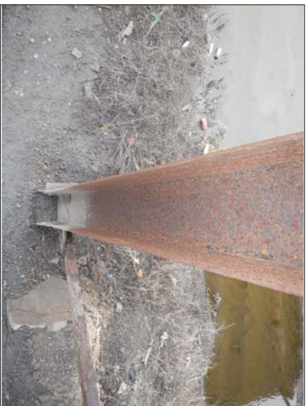
EXISTING CONDITION @ EAST COLUMN ABOVE FOOTING #25
