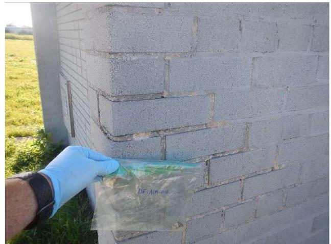
Photo 4. Sample location DF-ACM-01B, mortar sample, north-west corner of exterior wall of Drainage Facility Building.
