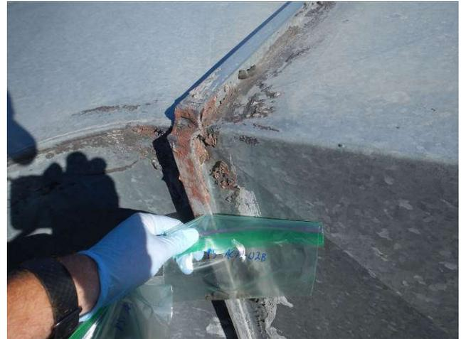
Photo 8. Sample location PS-ACM-02B, red duct mastic (also with black and grey layers), roof of Pumping Station Building.
