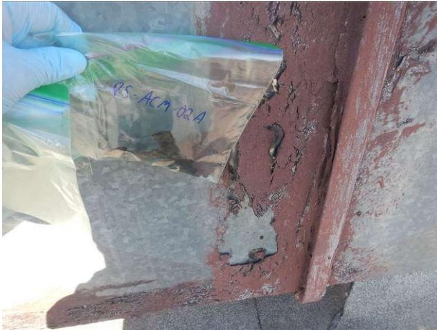
Photo 7. Sample location PS-ACM-02A, red duct mastic (also with black layer), roof of Pumping Station Building.
