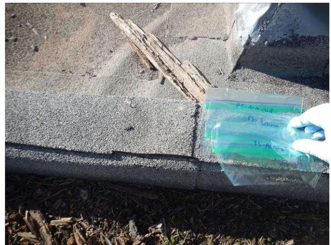
Photo 6. Sample location PS-ACM-01A/B/C, asphalt roof membrane, roof of Pumping Station Building.
