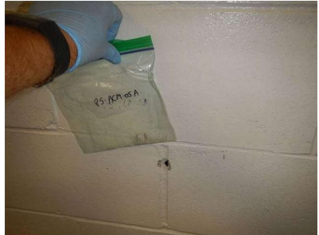
Photo 14. Sample location PS-ACM-05A, grey mortar, interior wall of "choline storage room" in Pumping Station Building.
