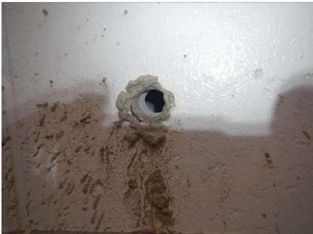
Photo 17. Hole drilled in concrete block wall in "chlorine storage room" in Pumping Station Building. Cavity was empty.
