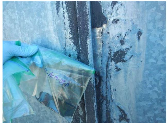
Photo 10. Sample location PS-ACM-03A, black duct mastic, roof of Pumping Station Building.
