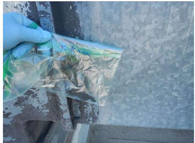
Photo 12. Sample location PS-ACM-03C, black duct mastic, roof of Pumping Station Building.
