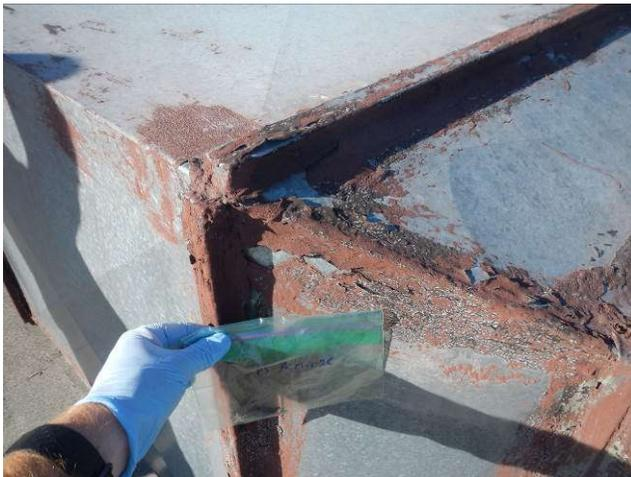
Photo 9. Sample location PS-ACM-02C, red duct mastic (also with black layer), roof of Pumping Station Building.
