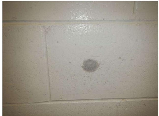
Photo 18. Repair of hole drilled in "chlorine storage room" in Pumping Station Building.
