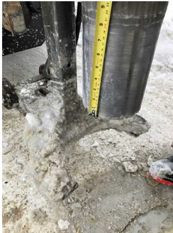
Photograph 38: Core Hole CH20-40 – Cathedral Avenue – Concrete not recovered
