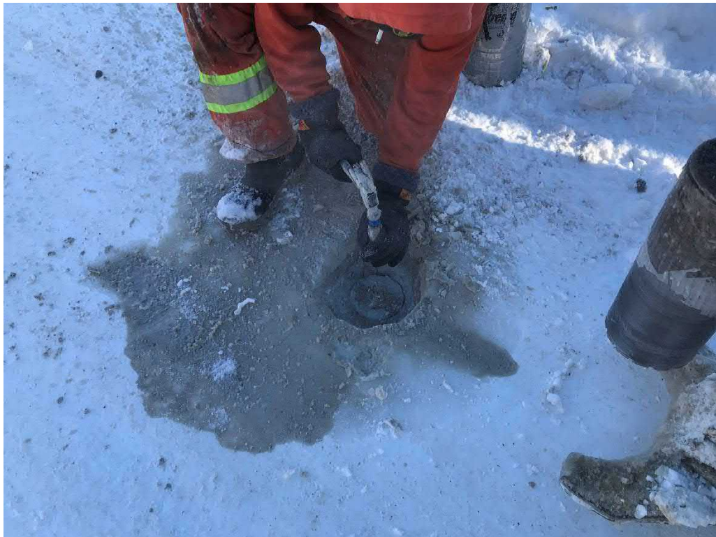
Photograph 54: Core Hole CH20-56 – Tanner Street – Concrete not recovered
