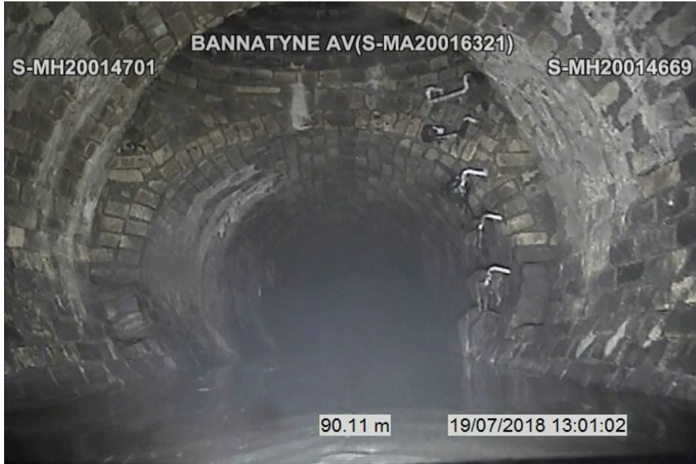
Figure 5 - Site 1: Bannatyne S-MA20016321 – Downstream Manhole
