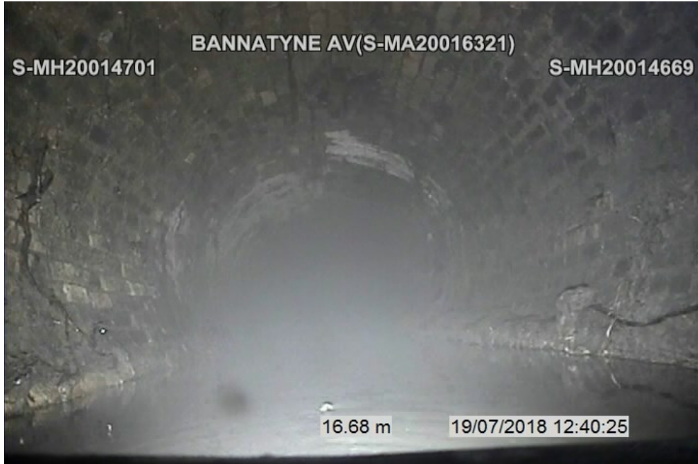
Figure 1 - Site 1: Bannatyne S-MA20016321 - General Conditions
