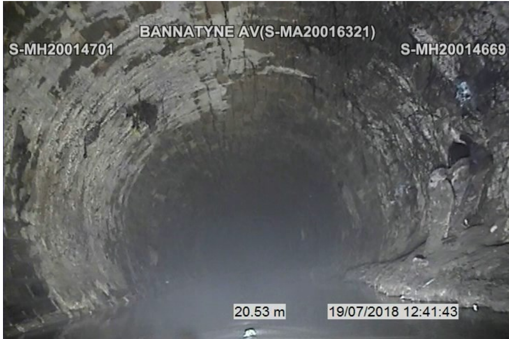
Figure 3 - Site 1: Bannatyne S-MA20016321 – General Condition
