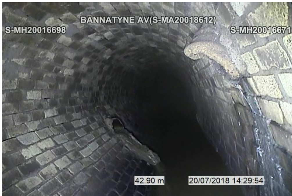
Figure 8 - Site 2: Bannatyne S-MA20018612 - General Condition w/ intruding service and encrustation
