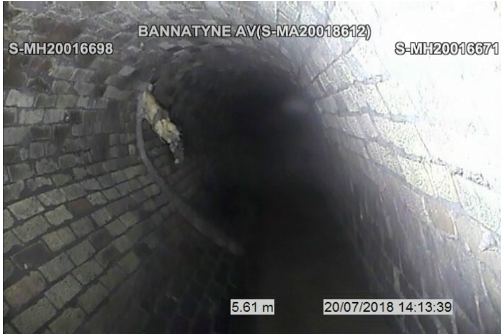
Figure 7 - Site 2: Bannatyne S-MA20018612 - General Condition w/ encrusted service
