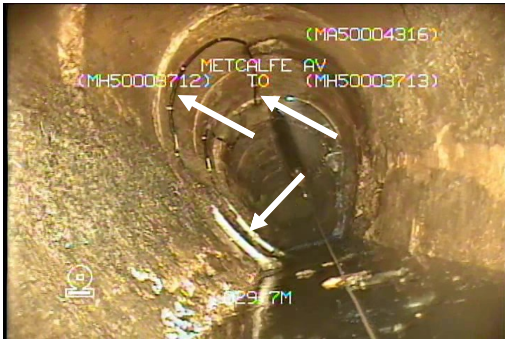
Figure 18 - Site 4: Metcalfe Av S-MA50004316 - Instrumentation and Cabling at S-MH50003713
