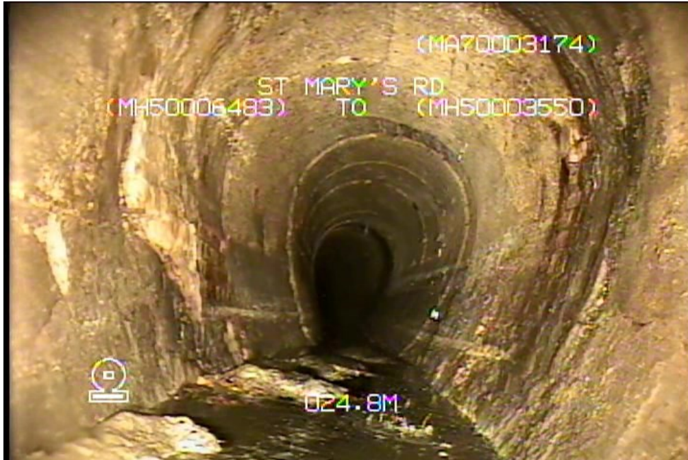
Figure 19 - Site 4: St Mary's Rd S-MA70003174 – General Conditions w/ Surface Spalling
