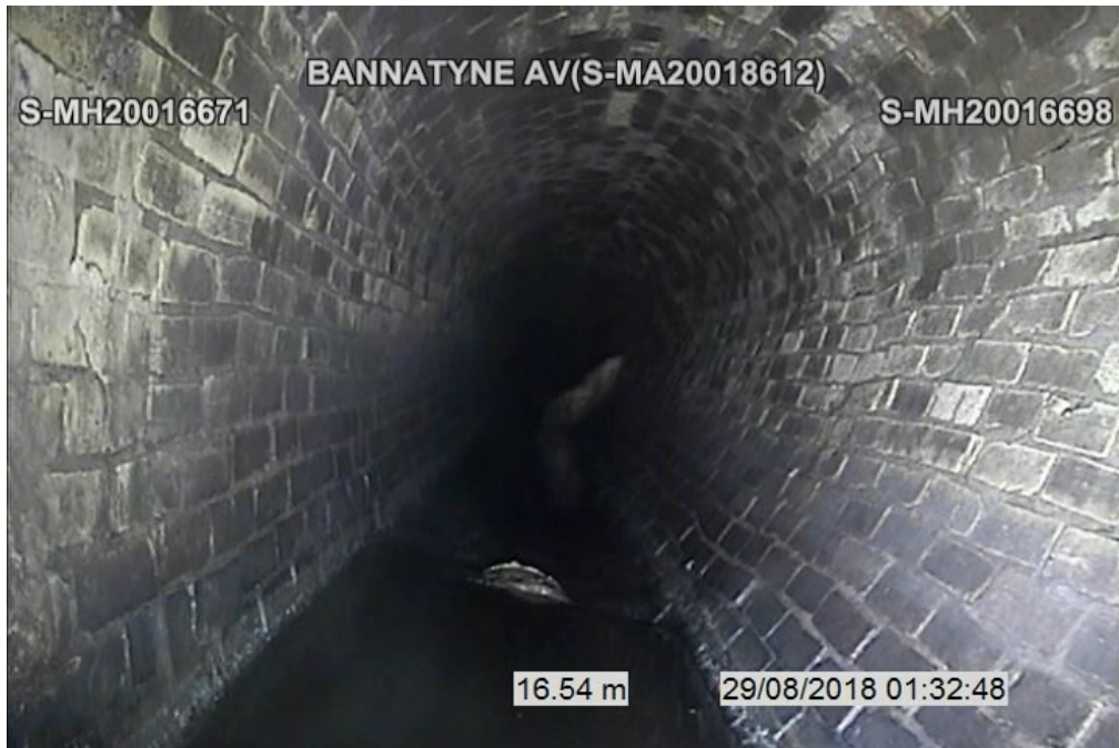
Figure 6 - Site 2: Bannatyne S-MA20018612 - General Condition
