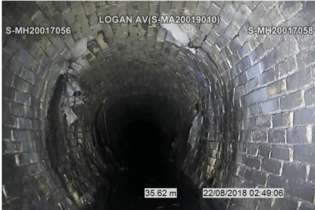
Figure 11 - Site 3: Logan Av S-MA20019010 - General Conditions w/ missing grout
