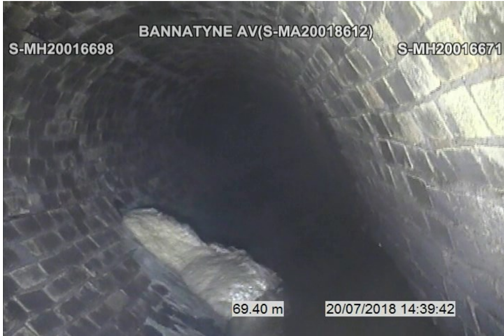
Figure 9 - Site 2: Bannatyne S-MA20018612 - General Condition w/ encrusted service
