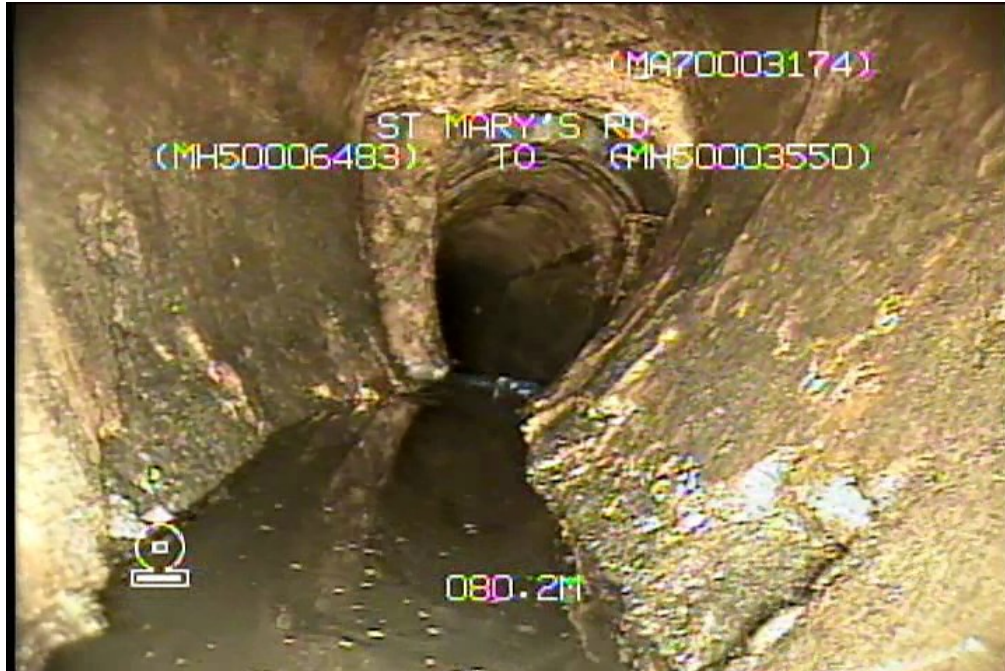
Figure 21 - Site 4: St Mary's Rd S-MA70003174 – General Conditions w/ Surface Spalling
