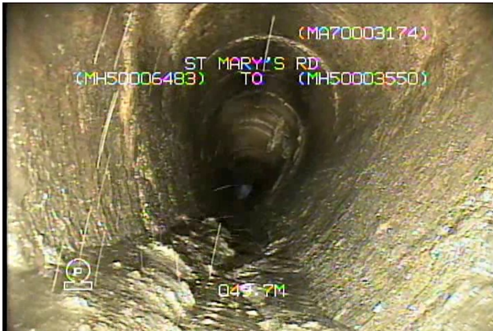
Figure 20 - Site 4: St Mary's Rd S-MA70003174 – General Conditions
