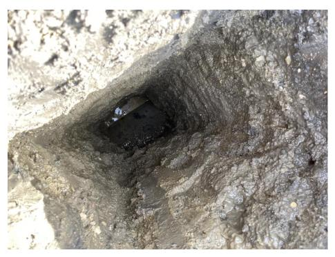
Photo 3. Land drainage sewer (LDS), obvert at 2.0 m below surface
