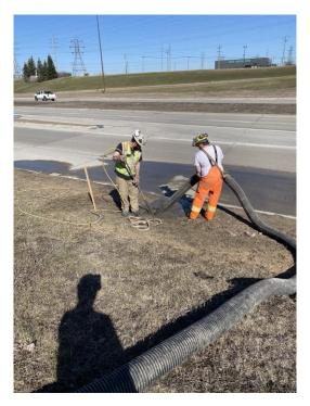
Photo 2. Looking west, hydro-excavation at the toe
