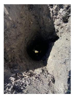
Photo 6. High pressure gas line at the cress, obvert at 2.7 m below surface
