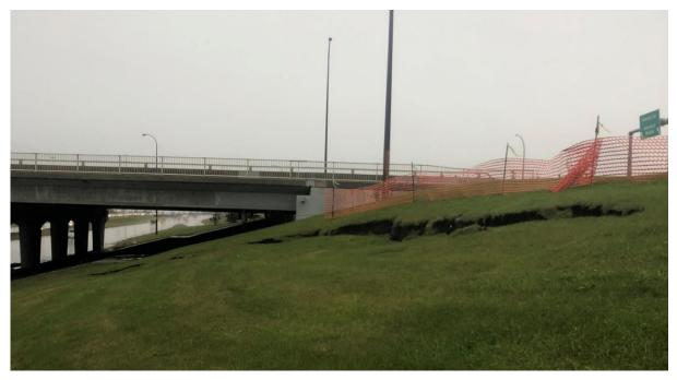
Photo 1 (2019-10-21) Looking East at Head Scarp (Pembina Highway bridge in background)
