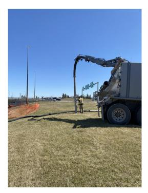
Photo 5. Looking east, hydro-excavation at the cress
