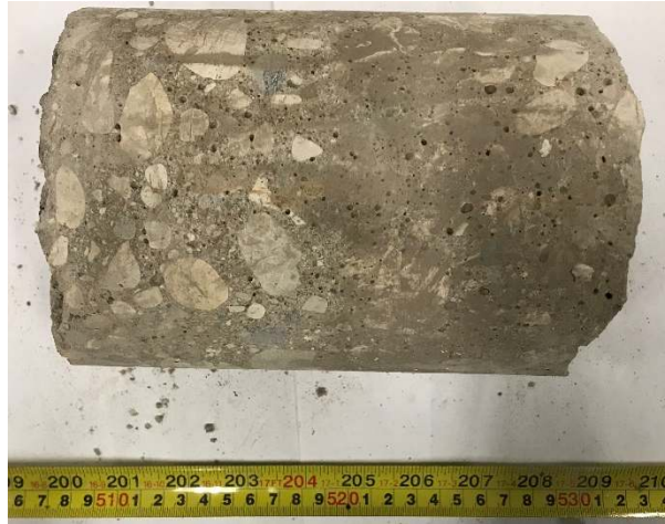
GRO1-03: Concrete Layer, Profile View
