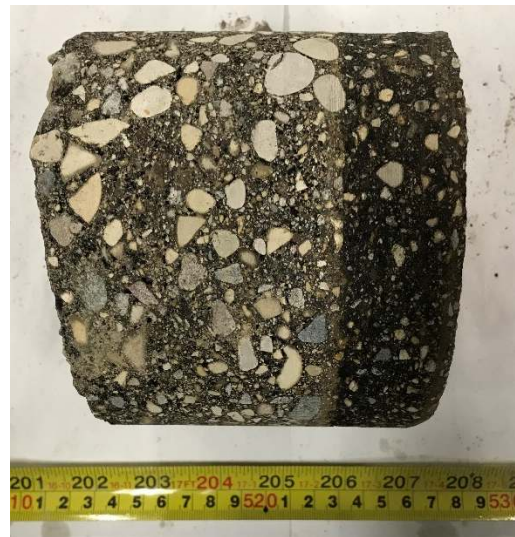
DOW-04: Asphalt Layer, Profile View
