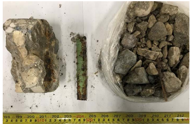
GRO1-02: Concrete Layer, Profile View
