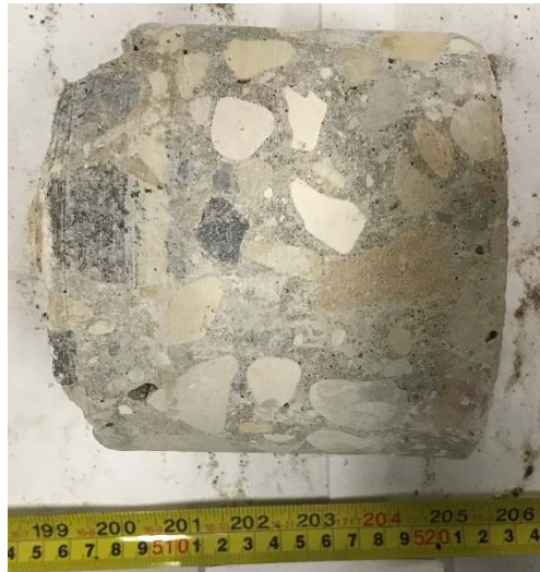
SYR-06: Broken Concrete Layer, Profile View
