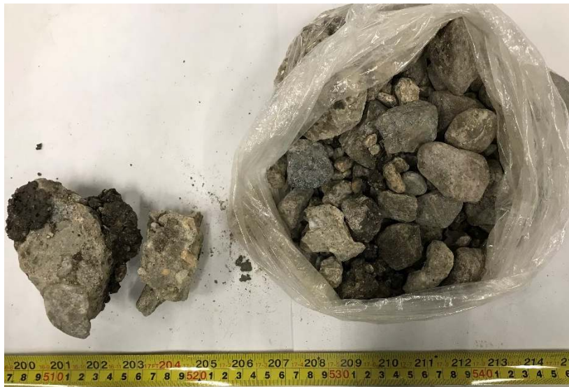
RIL-04: Concrete Layer (Broken), Plan View
