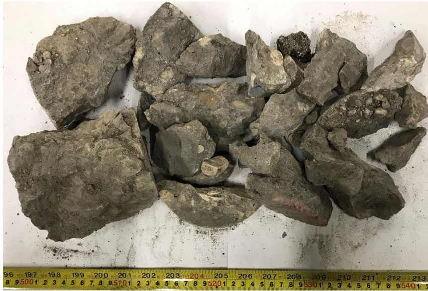
NAT1-01: Broken Concrete Core. Plan View
