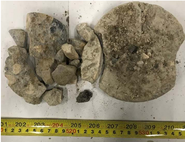
SYR-06: Broken Concrete Layer, Plan View
