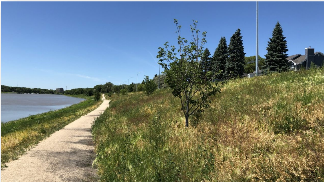
Photo 1 - Mid-bank pathway / stabilized riverbank from Monck to Gauvin
