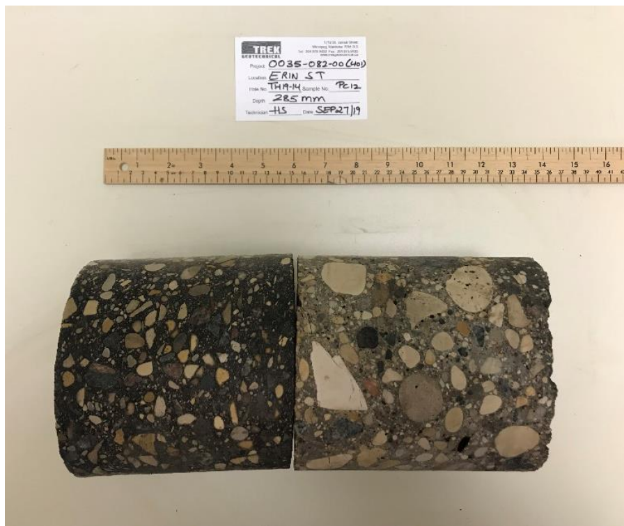
Photo 14: Pavement Core Sample at Test Hole TH19-14
