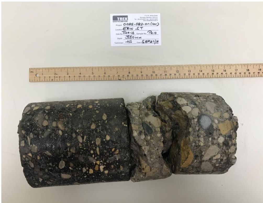
Photo 16: Pavement Core Sample at Test Hole TH19-16
