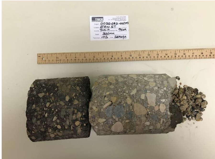
Photo 17: Pavement Core Sample at Test Hole TH19-17
