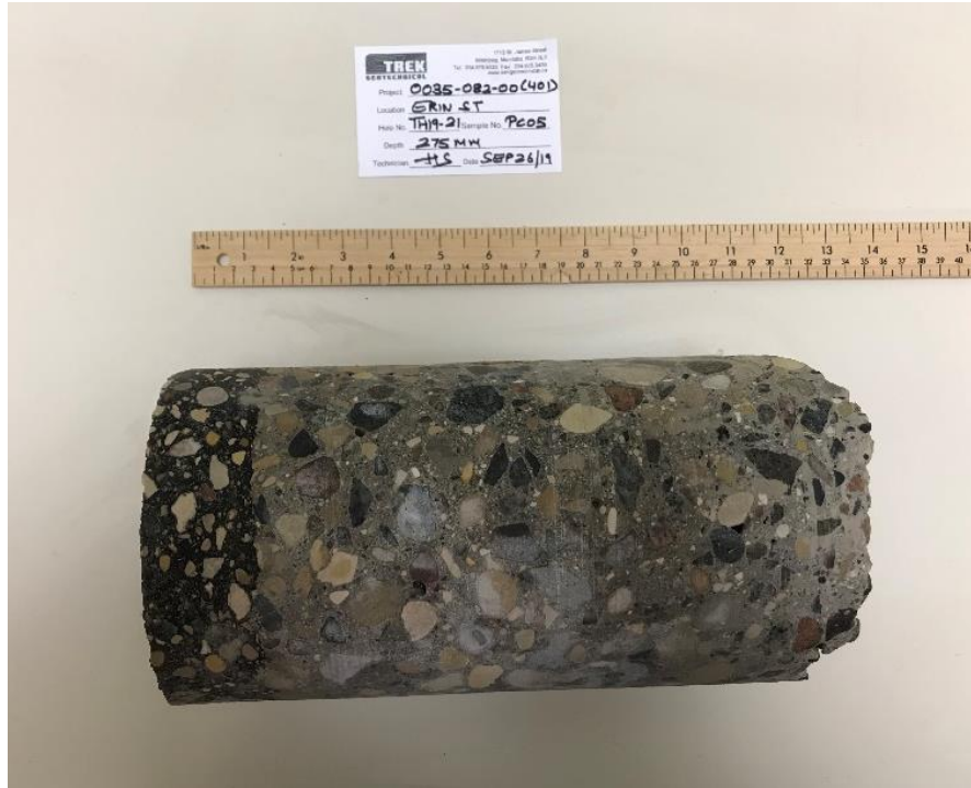
Photo 21: Pavement Core Sample at Test Hole TH19-21
