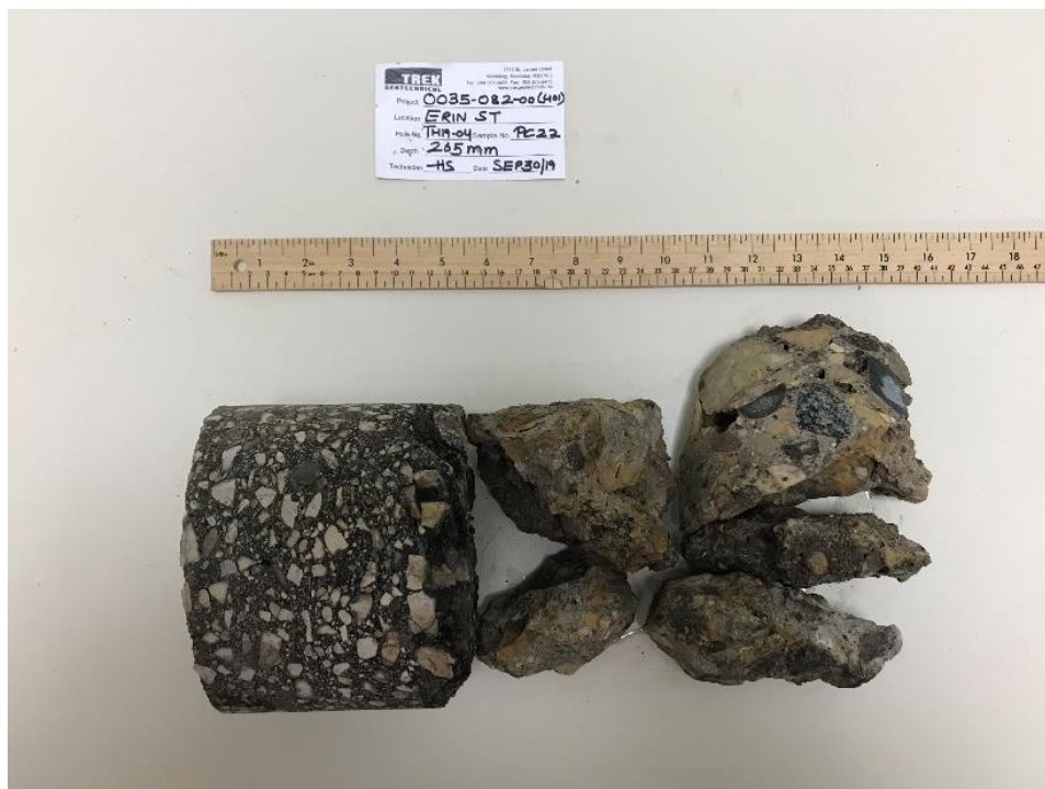
Photo 4: Pavement Core Sample at Test Hole TH19-04
