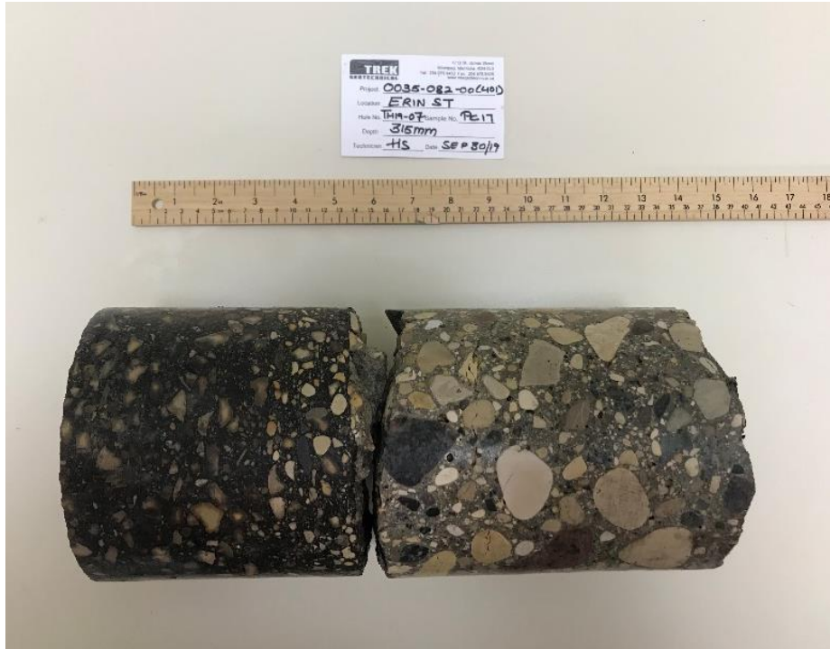
Photo 9: Pavement Core Sample at Test Hole TH19-09
