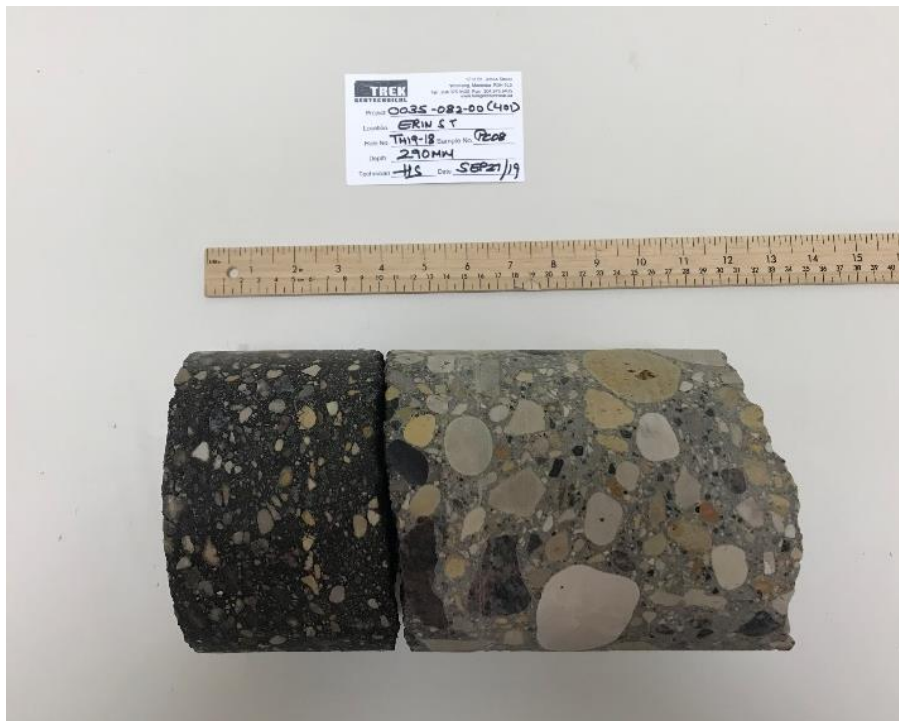
Photo 18: Pavement Core Sample at Test Hole TH19-18
