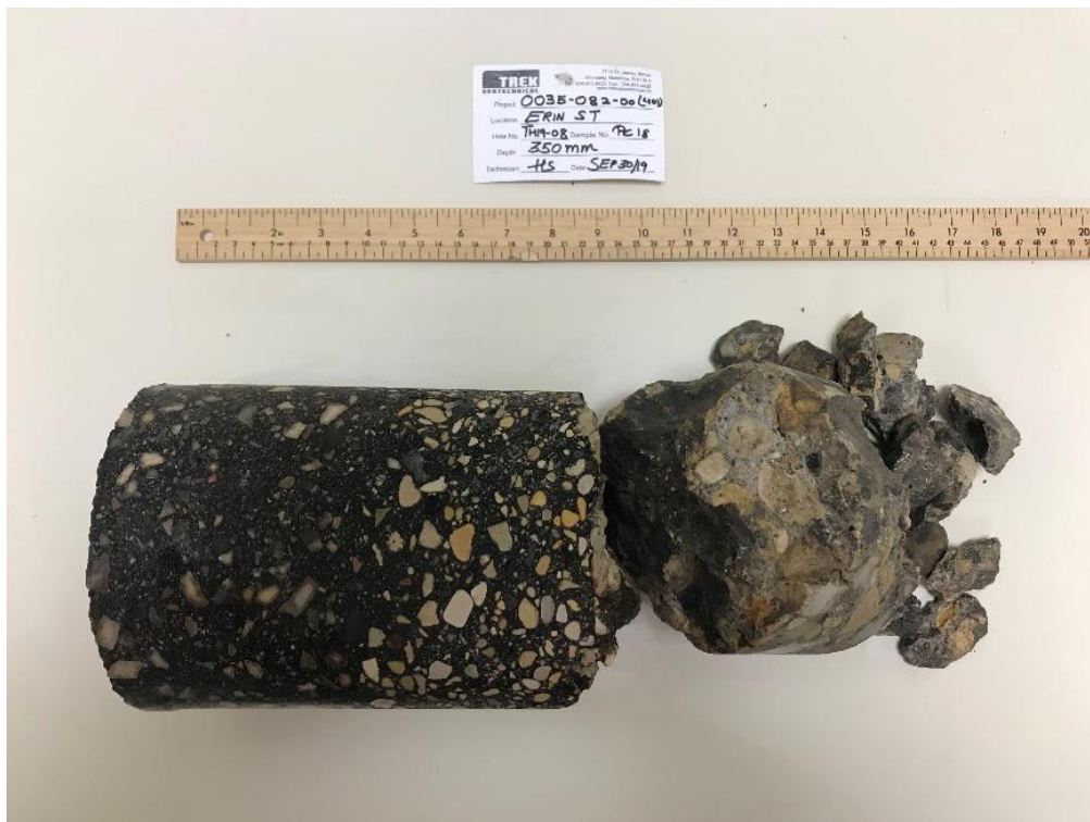
Photo 8: Pavement Core Sample at Test Hole TH19-08
