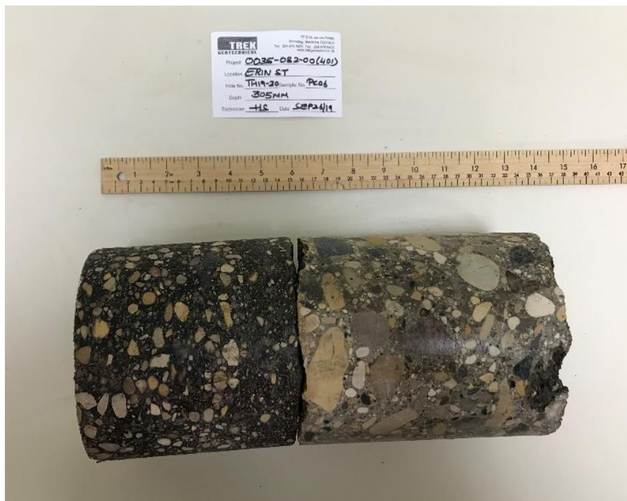
Photo 20: Pavement Core Sample at Test Hole TH19-20
