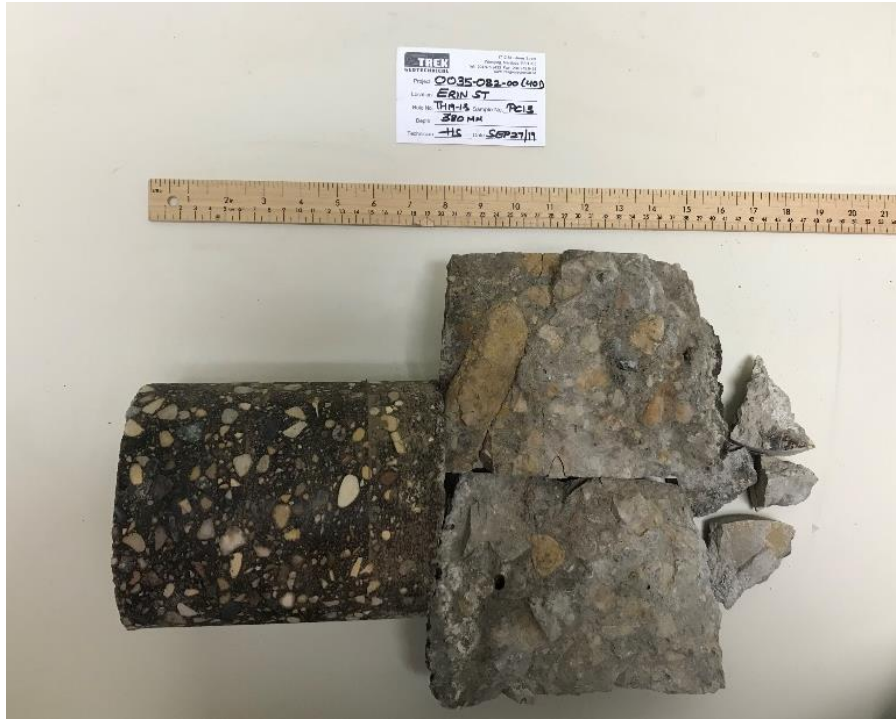
Photo 13: Pavement Core Sample at Test Hole TH19-13
