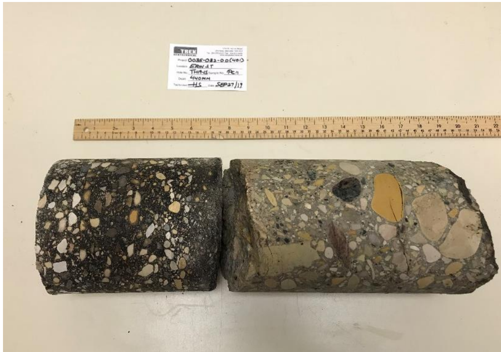
Photo 15: Pavement Core Sample at Test Hole TH19-15
