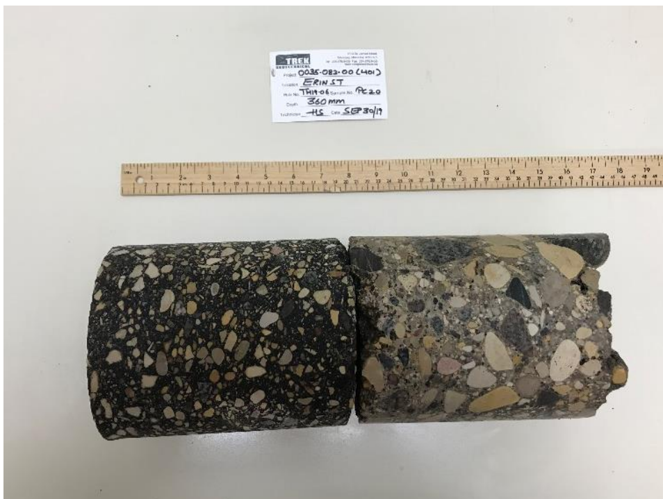
Photo 6: Pavement Core Sample at Test Hole TH19-06
