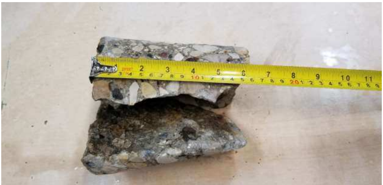
South bound transverse joint, Sta. 1+200
