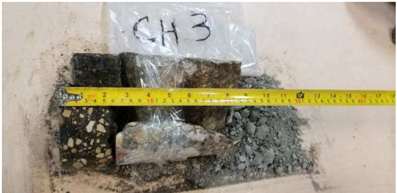
South bound transverse joint, Sta. 1+515
