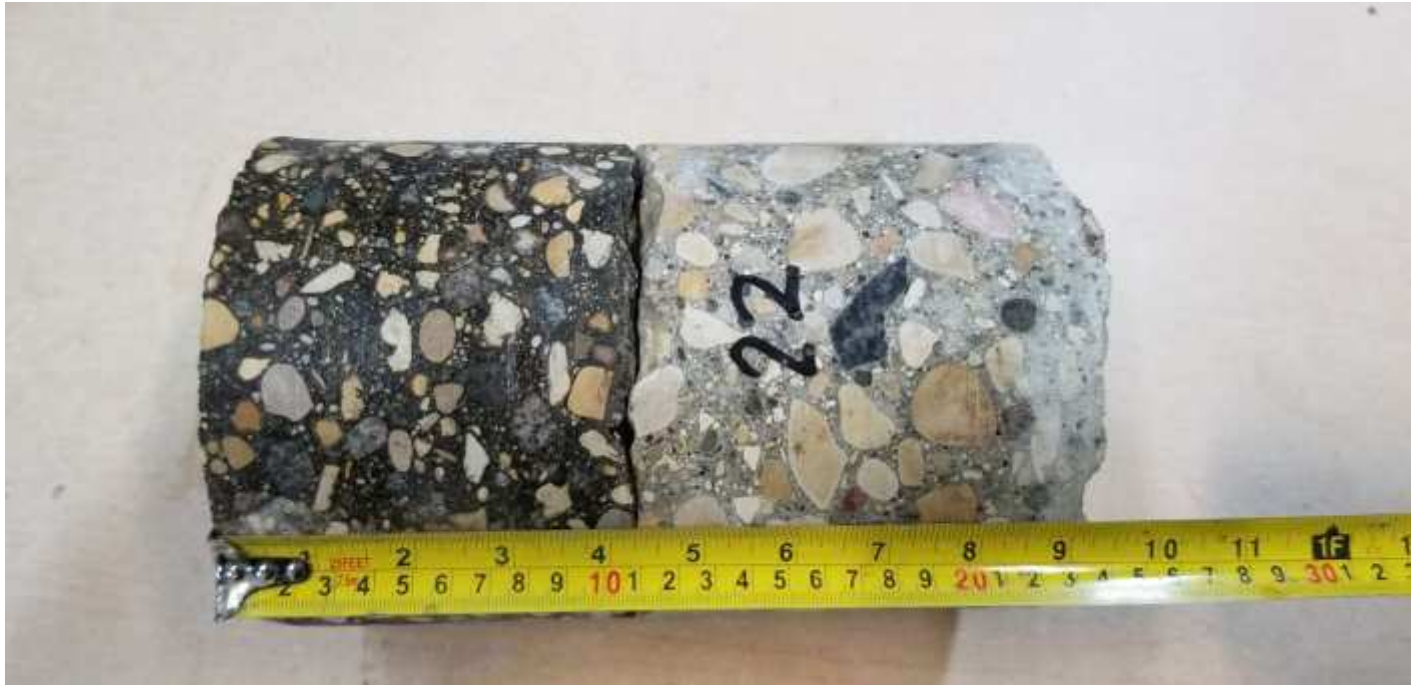
TH 12, north bound Sta. 1+000, lower part of concrete core could not be recovered
