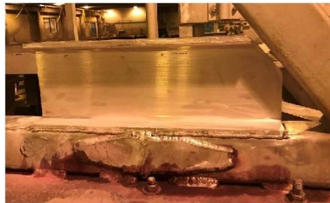
Emergency repair to crack – November 21, 2019
