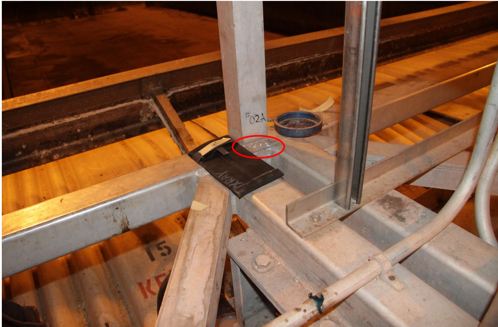
Fig. 15: North-East Corner of Bridge, Rough welding at Location #2A
