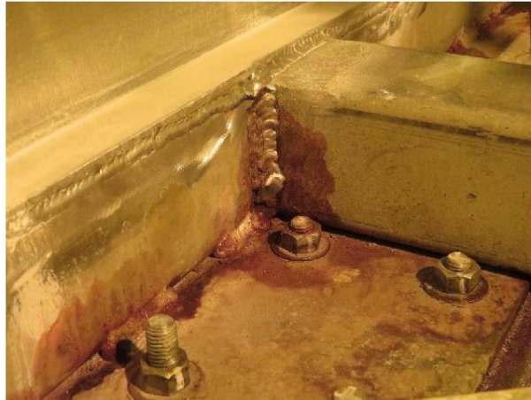
Cracked fillet weld east side of HSS member at joint (11B)
