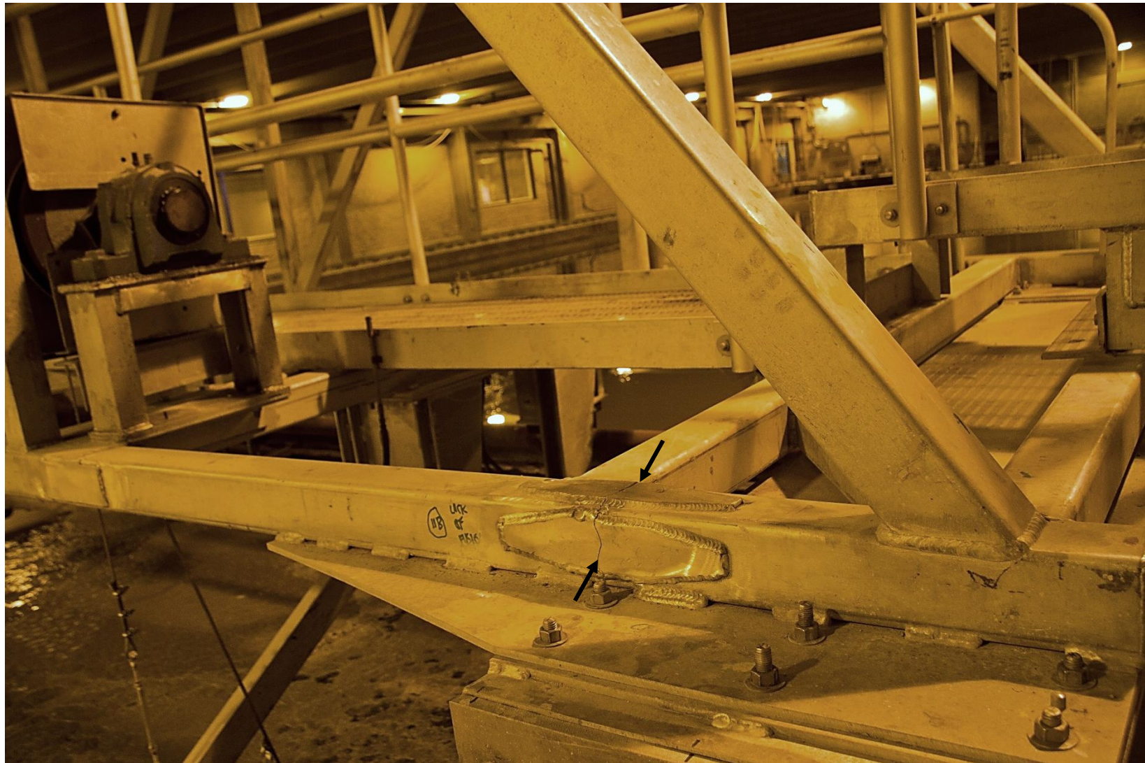
Fig. 6: South-West Corner of Bridge, Location #11B
