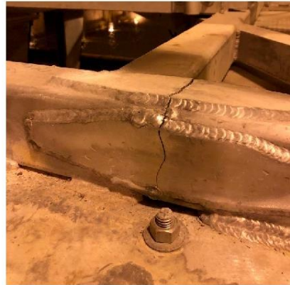
Crack in primary clarifier No. 3 travelling bridge truss
