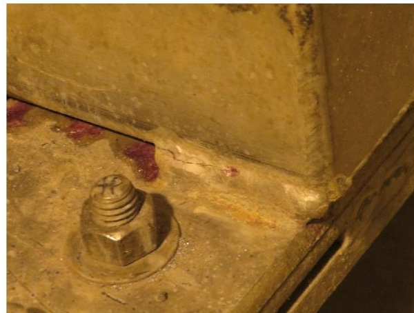
Cracked fillet weld on the top of the chord gusset plate above the end truck (southwest corner)
