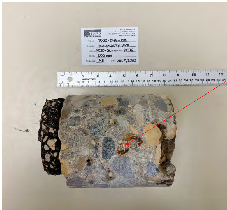
Photo 6: Pavement Core Sample at PC20-06
