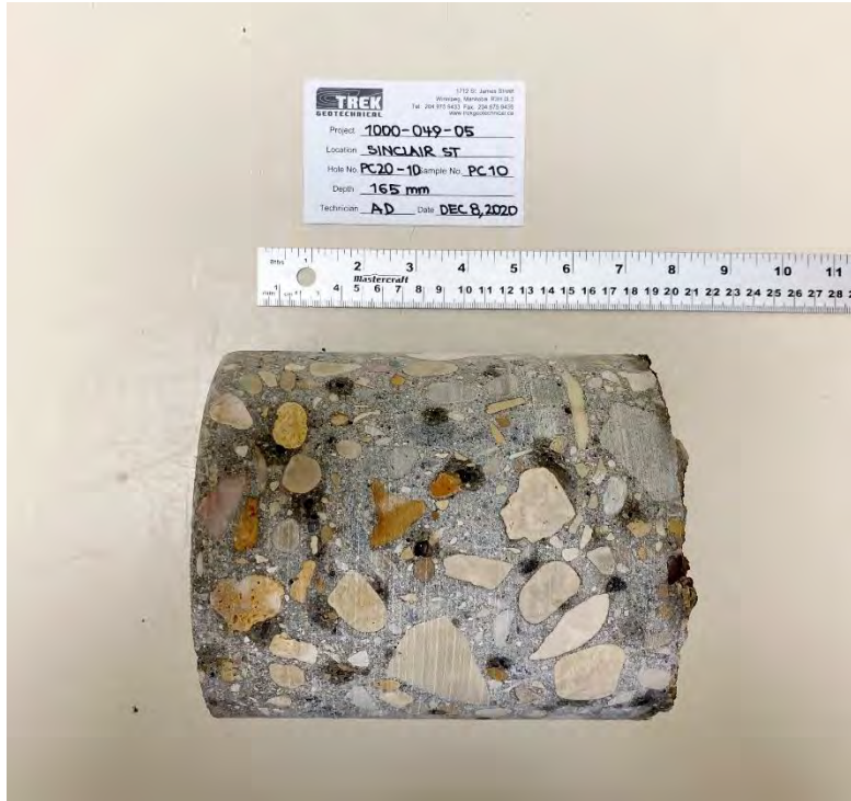
Photo 3: Pavement Core Sample at PC20-10
