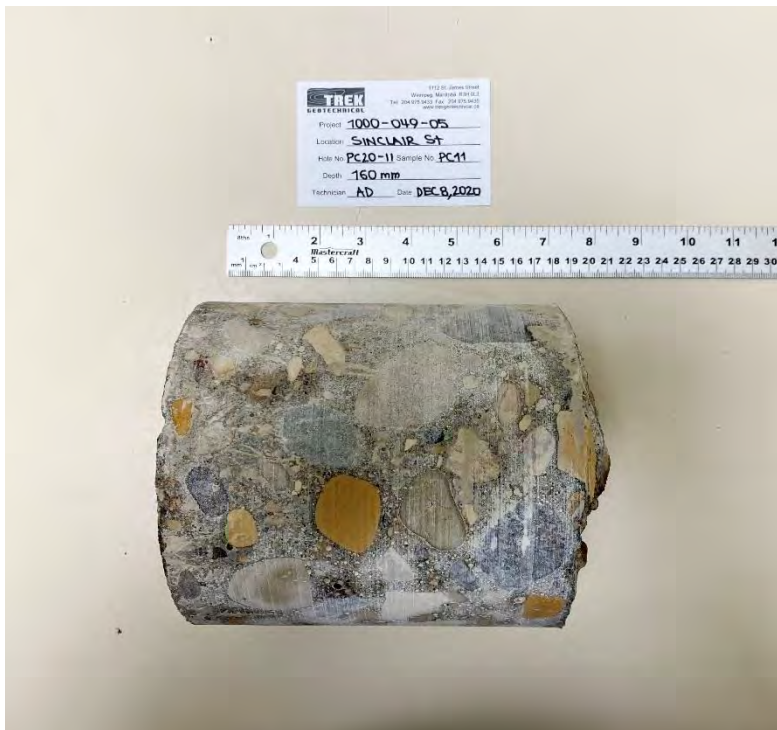
Photo 4: Pavement Core Sample at PC20-11
