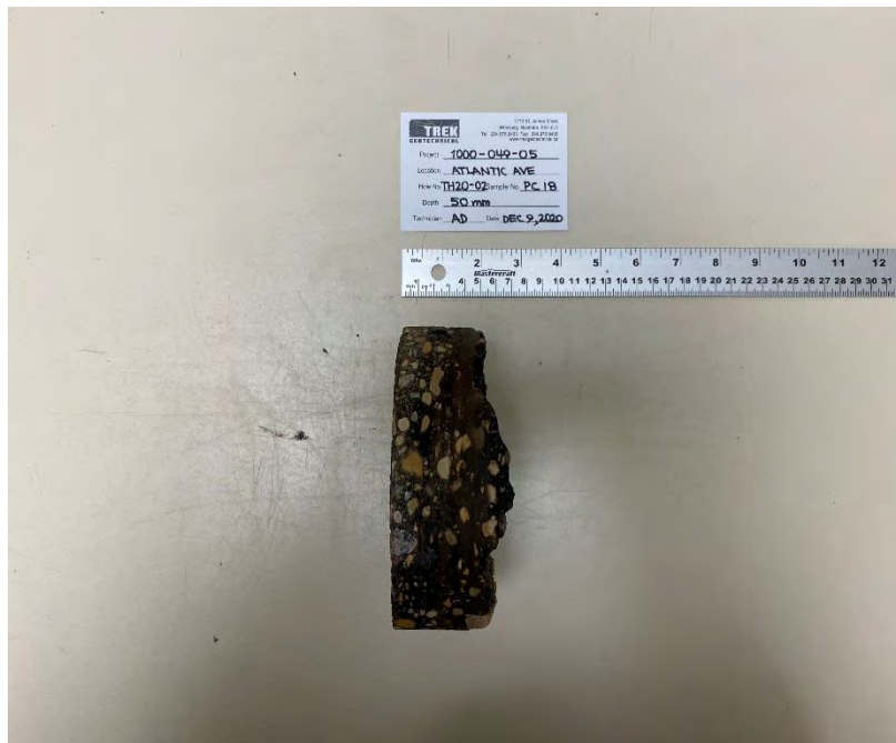
Photo 2: Pavement Core Sample at Test Hole TH20-02
