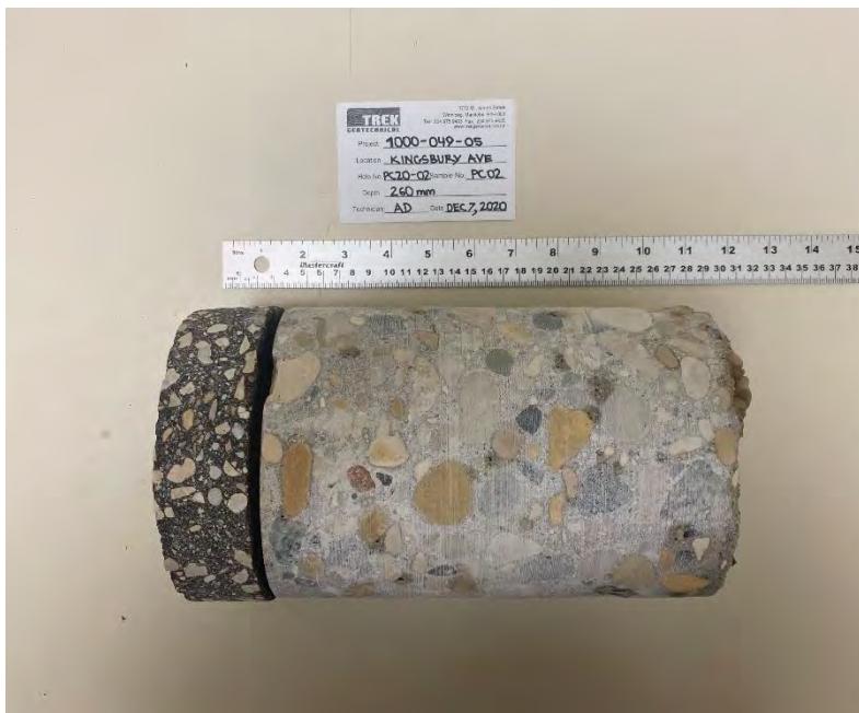
Photo 2: Pavement Core Sample at PC20-02
