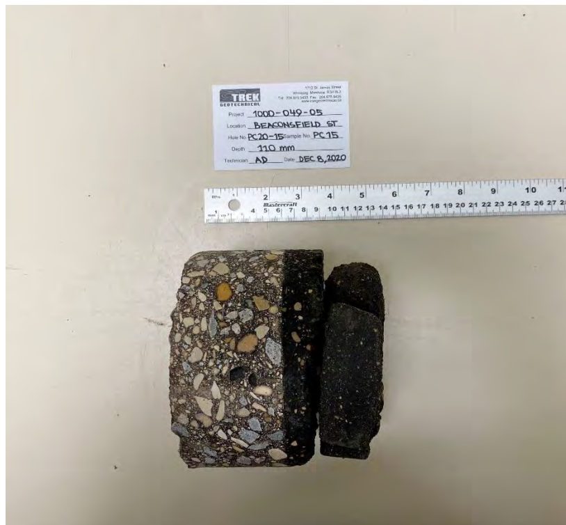
Photo 2: Pavement Core Sample at PC20-15
