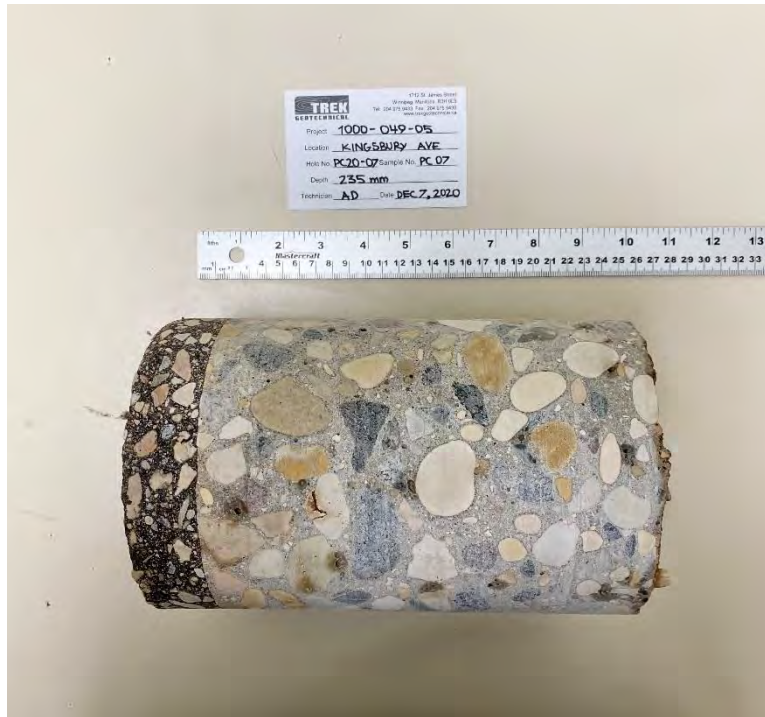
Photo 7: Pavement Core Sample at PC20-07
