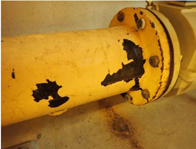
Photo 1. Paint Sample S-01 location (beige piping system; RAS 1; composite sample).
