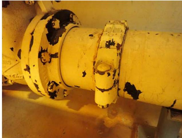
Photo 2. Paint Sample S-01 location (beige piping system; RAS 1; composite sample).
