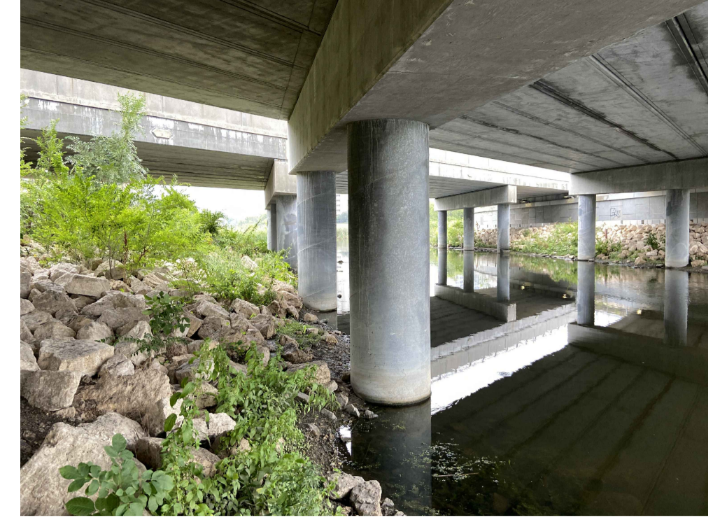
LOOKING WEST ALONG LOWER BANK DATE 2021-09
