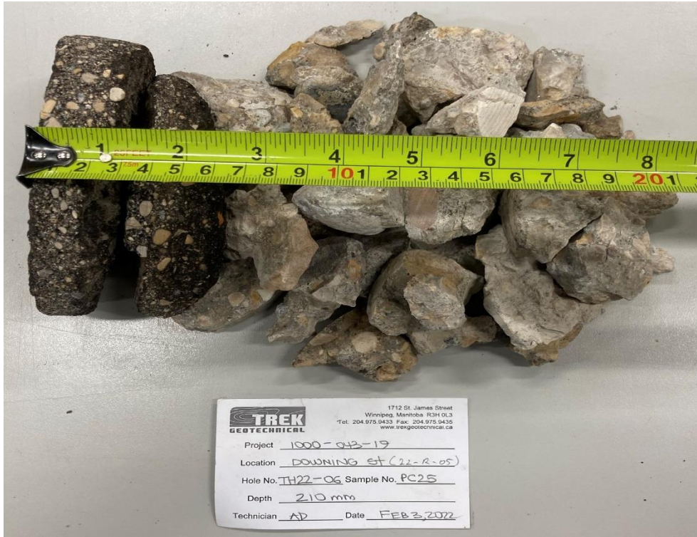
Photo 3: Pavement Core Sample at Test Hole TH22-06
