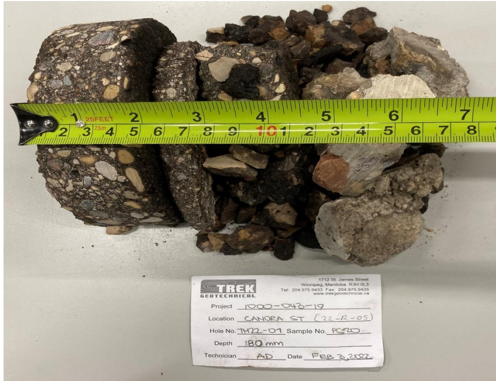
Photo 1: Pavement Core Sample at Test Hole TH22-01
