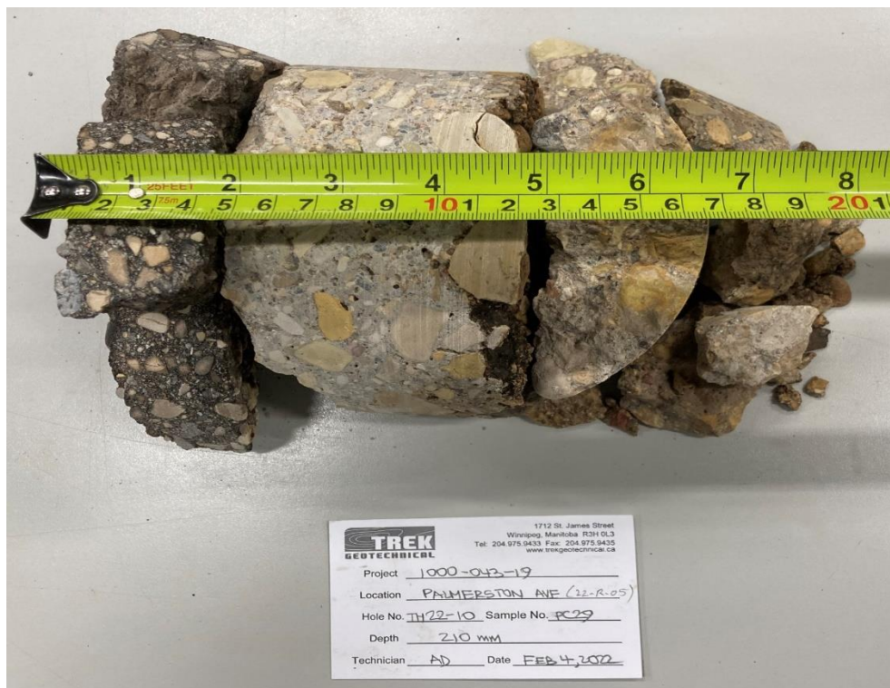
Photo 4: Pavement Core Sample at Test Hole TH22-10
