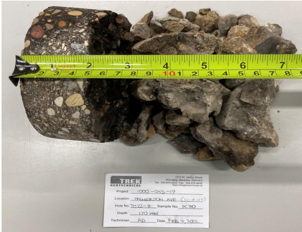
Photo 5: Pavement Core Sample at Test Hole TH22-11
