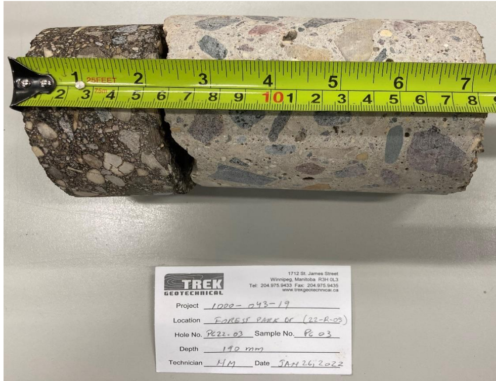
Photo 3: Pavement Core Sample at PC22-03
