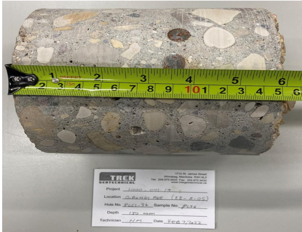
Photo 3: Pavement Core Sample at PC22-36
