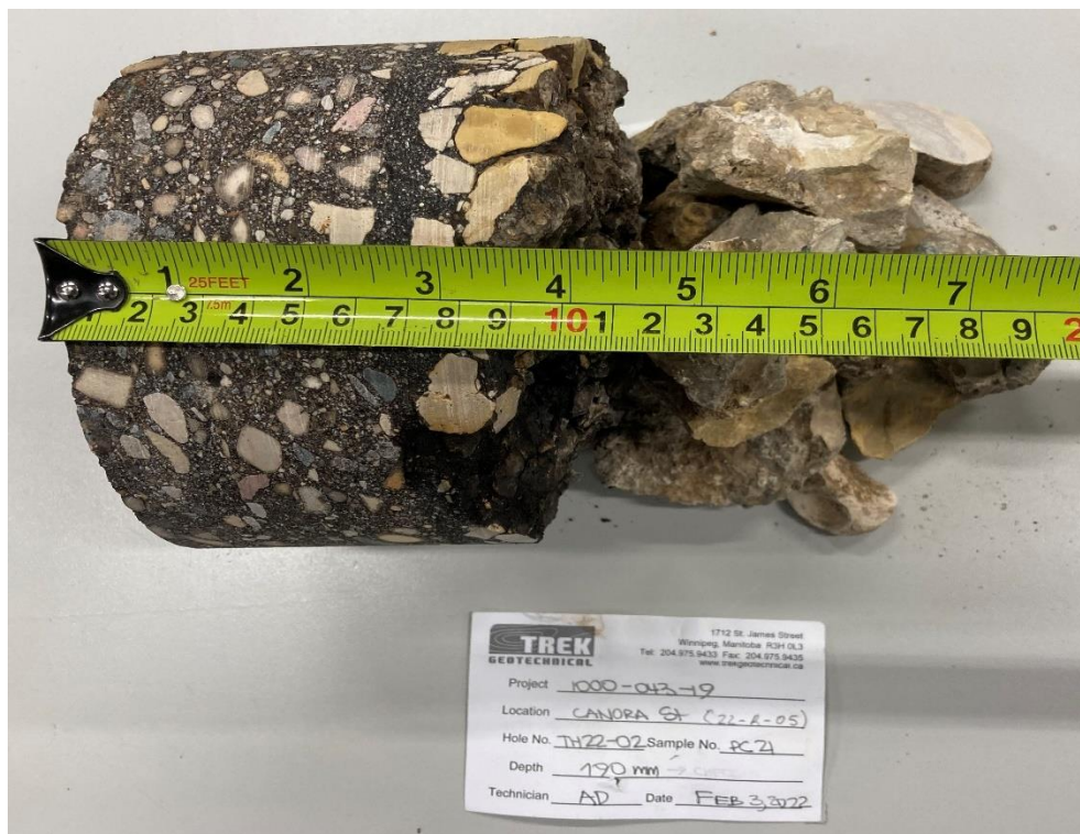
Photo 2: Pavement Core Sample at Test Hole TH22-02
