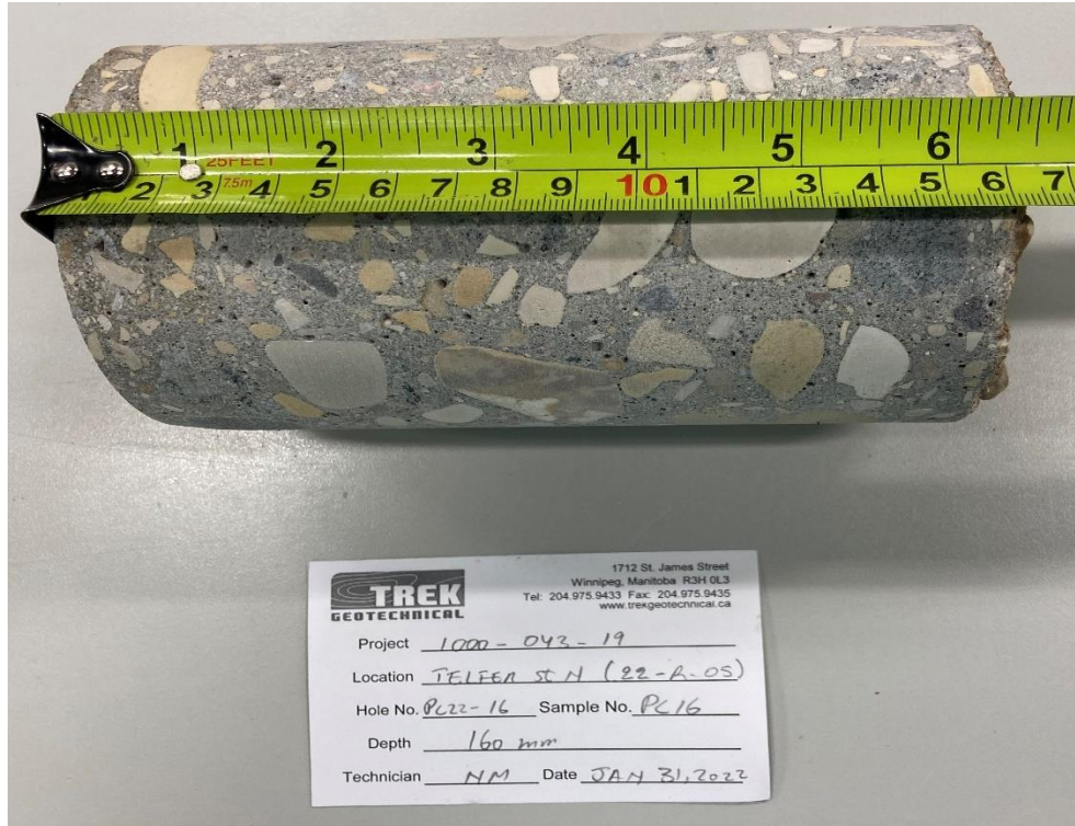
Photo 5: Pavement Core Sample at PC22-16
